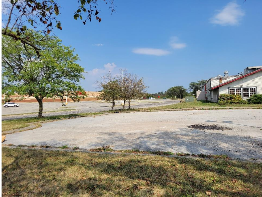
Photo 3: Subject Site from West
