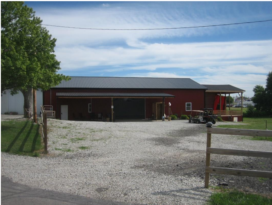
Subject site accessory structure, looking south
