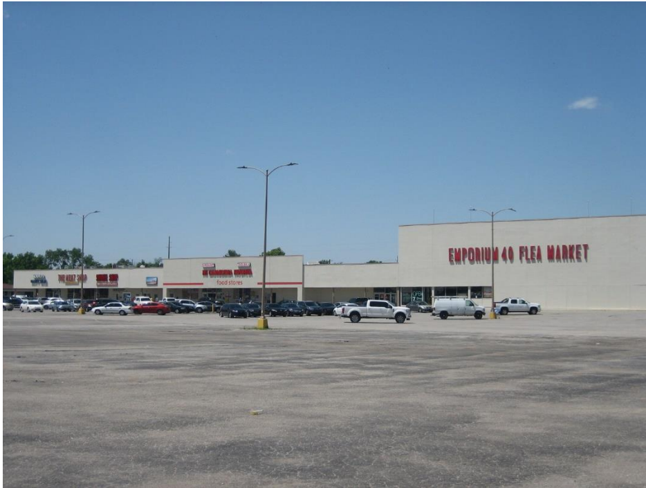
Adjacent commercial retail intergaged center, looking north.
