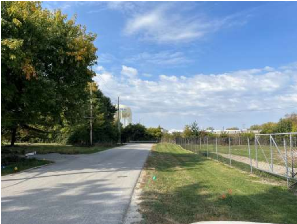
Photo looking west on Hanna Avenue.
