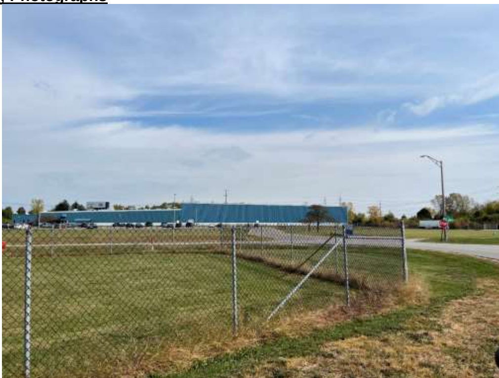
Photo of industrial property to the northeast.
