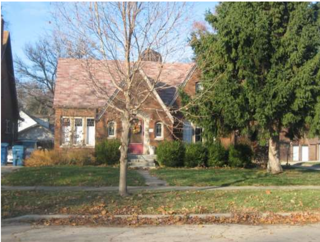
Adjacent property to the south, looking north.
