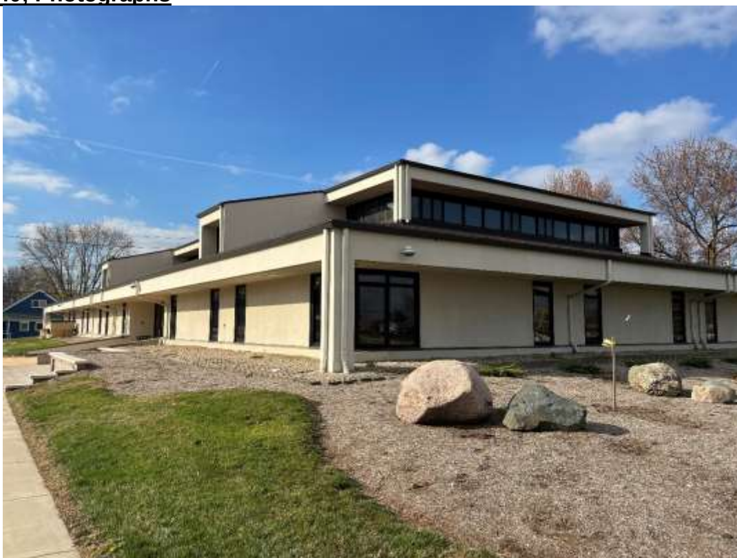
Photo of the Subject Property: 1220 South High School Road
