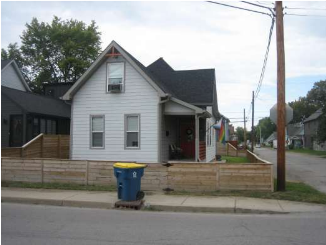
Subject site, looking north.
