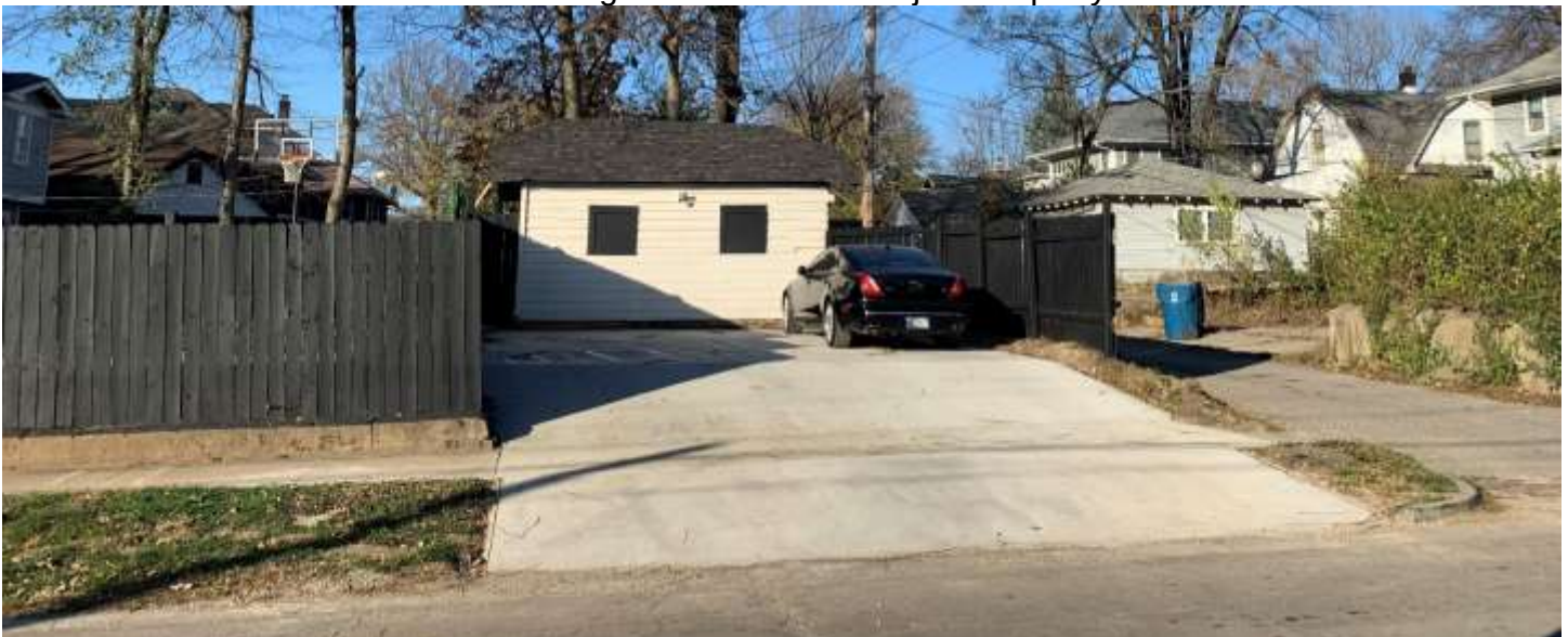
2022 Photo of the Subject Property.
