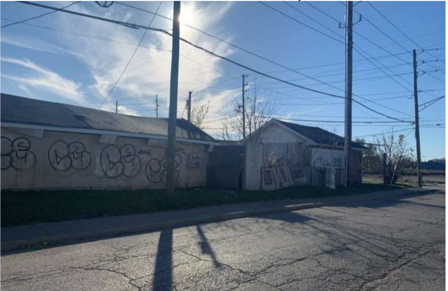
Photo of the industrial property to the south.
