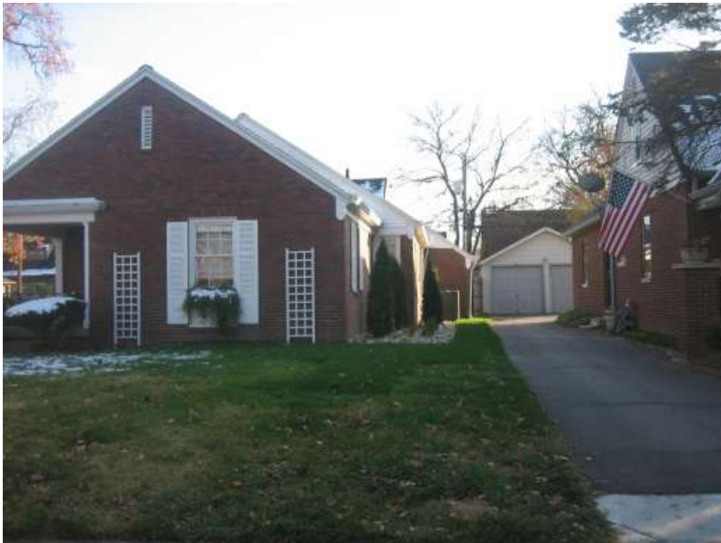
Subject site with existing one-foot west side setback, looking south
