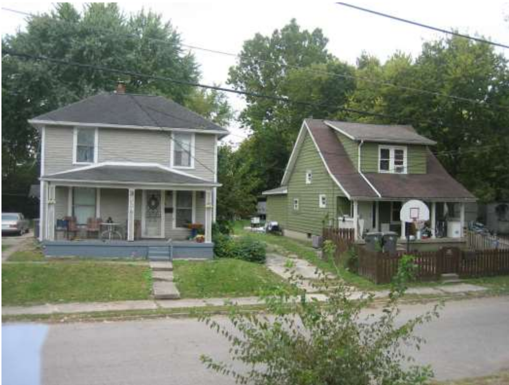
Adjacent single-family dwellings to the south.
