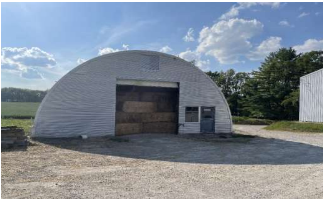
Photo Six: Storage Building, Facing West
