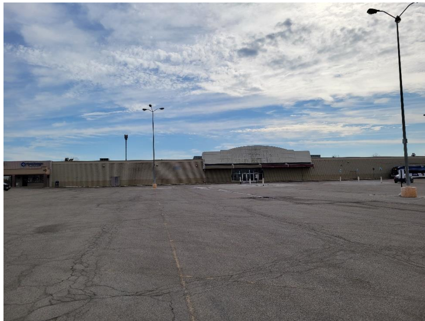
Photo 2: Lot 1 Building Site + Vacant Building (to be removed)
