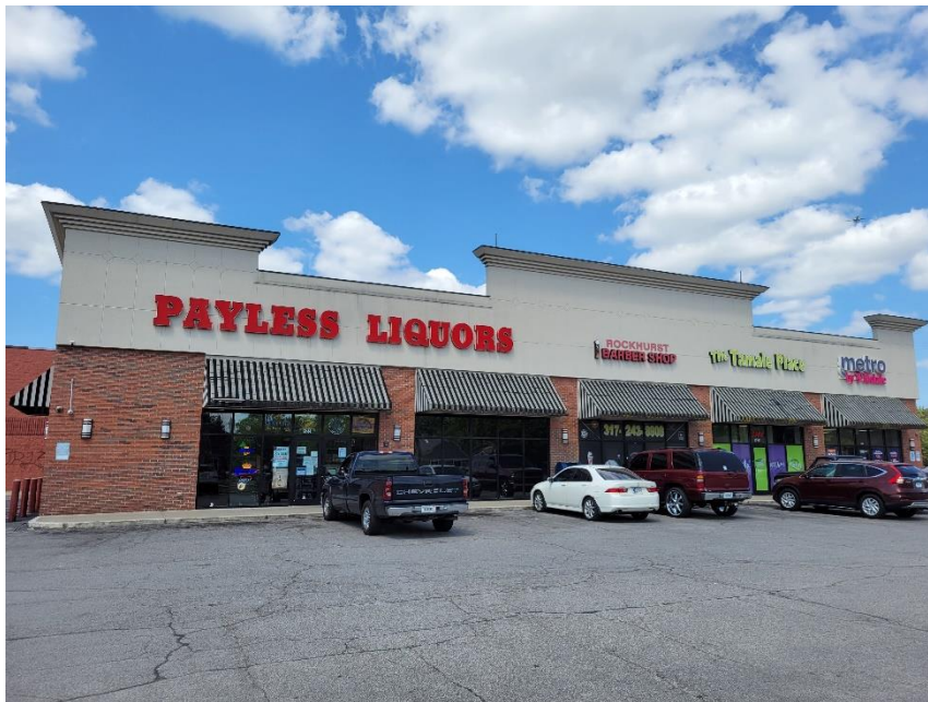
Photo 2: Subject Property Viewed from South
