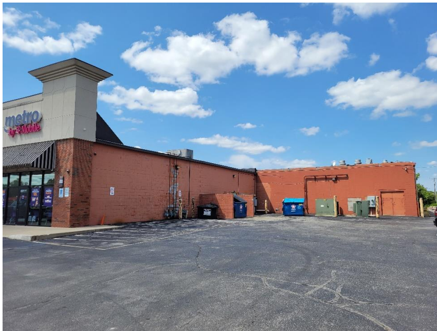
Photo 4: Subject Property + Dumpster Viewed from Southeast
