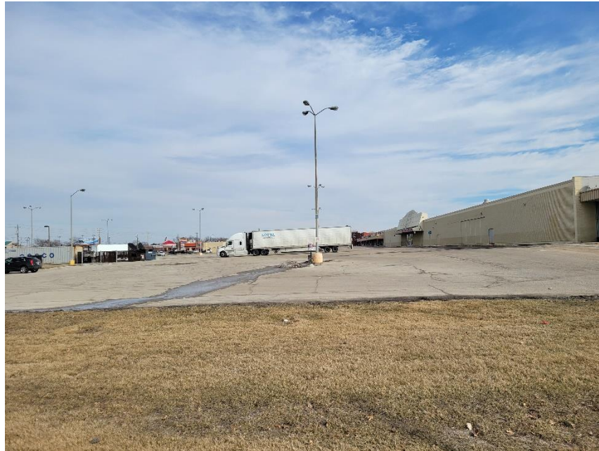
Photo 3: Lot 3 Building Site from Emerson to West
