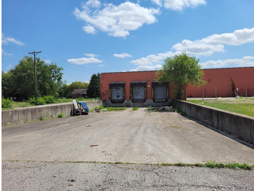
Photo 3: Subject Property + Loading Docks Viewed from North
