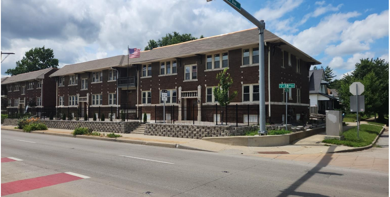
Subject site, 546 East 38 th Street with existing non-compliant fencing. Looking northwest.
