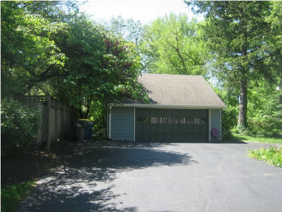
Existing garage with 5.5-foot side yard setback, looking west.
