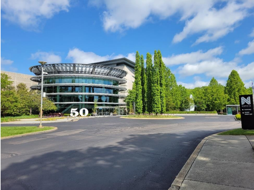
Photo 1: Primary Building Viewed from South
