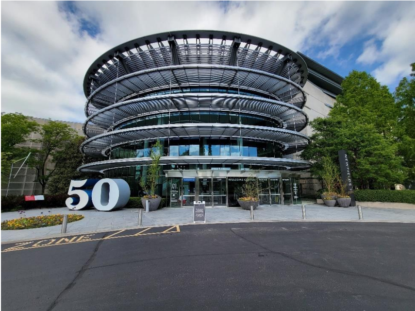
Photo 2: S1 Sign Location Viewed from West
