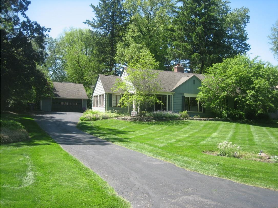
Subject site, existing dwelling, looking west.
