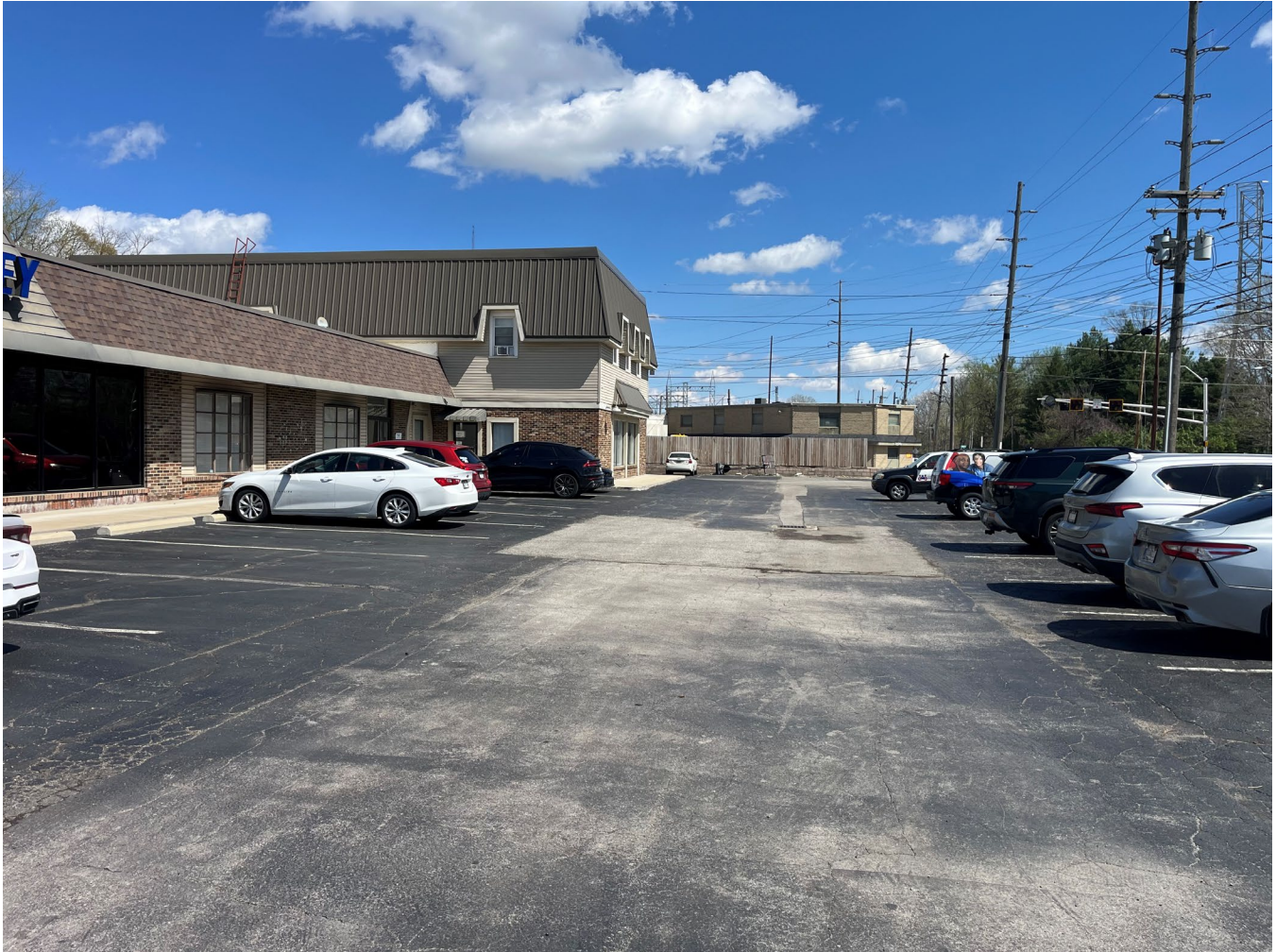
Photo 3: Parking lot of subject site looking east. Pedestrian beacon for Nickel Plate Trail can be seen in background
