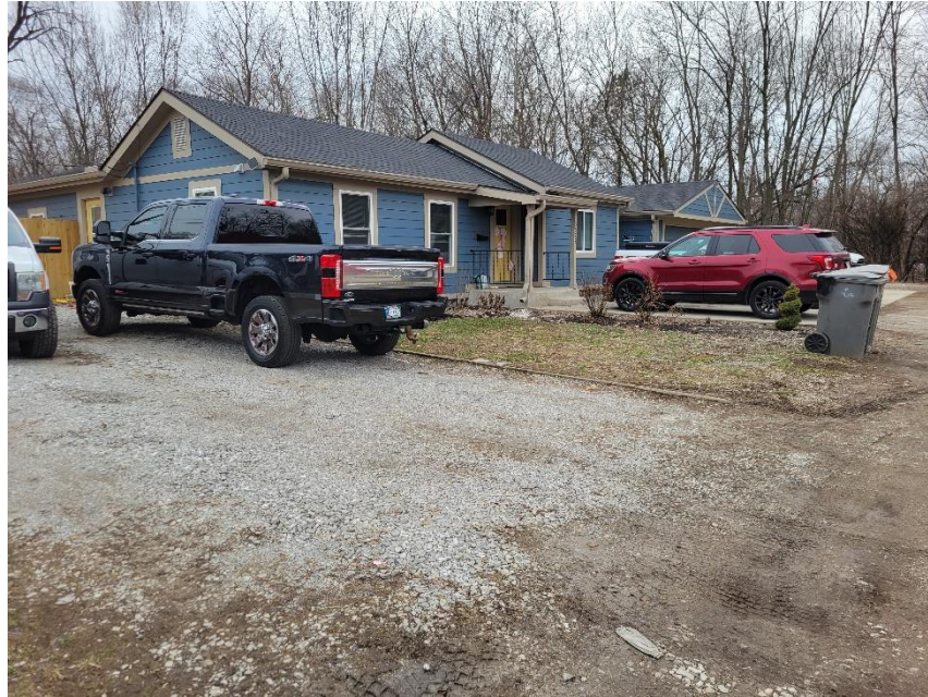
Photo 3: Subject Site Front Yard Viewed from East
