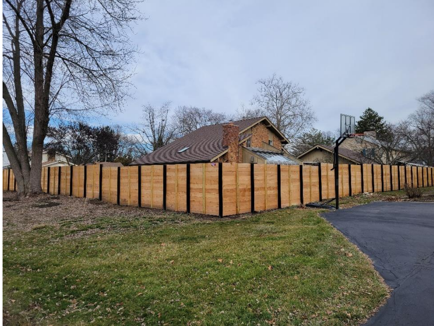
Photo 3: Fence from Southwest
