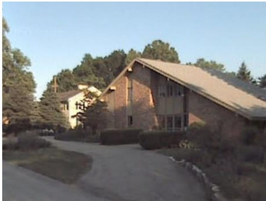
Photo 6: Driveway/Parking Area in Front Yard (taken September 2007)
