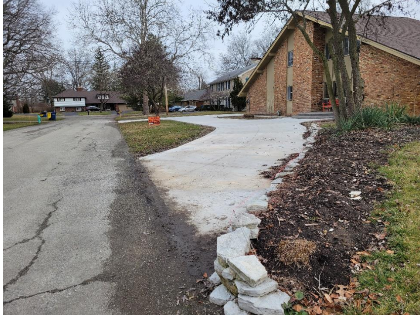
Photo 5: Existing Driveway/Parking Area in Front Yard (North)
