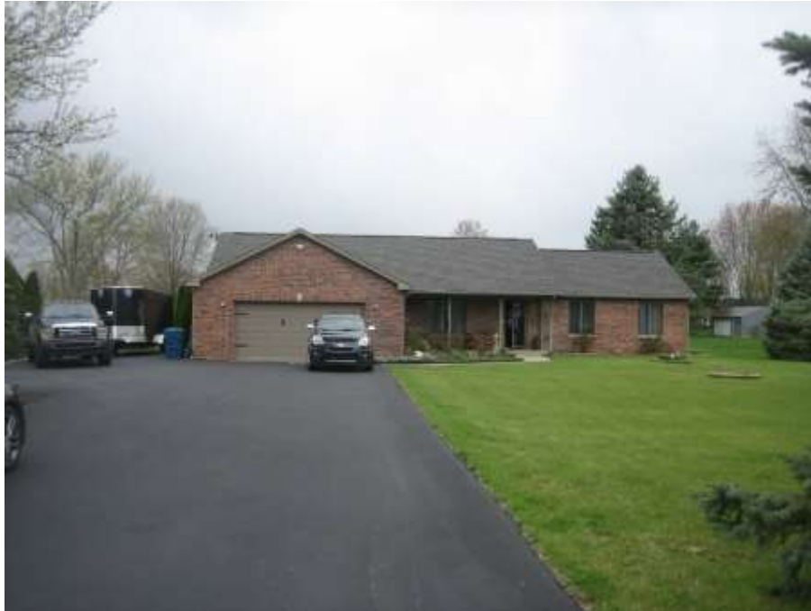
Subject site single family dwelling, looking west
