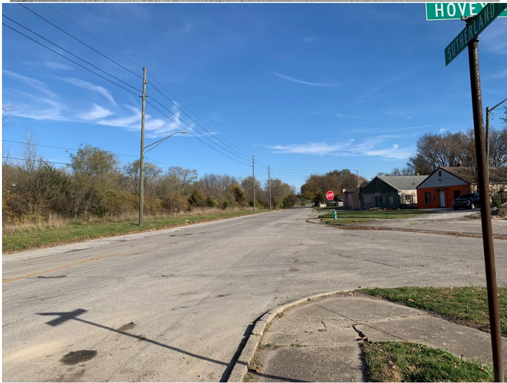
Views of the site from Sutherland Avenue (top); view of Sutherland Avenue
