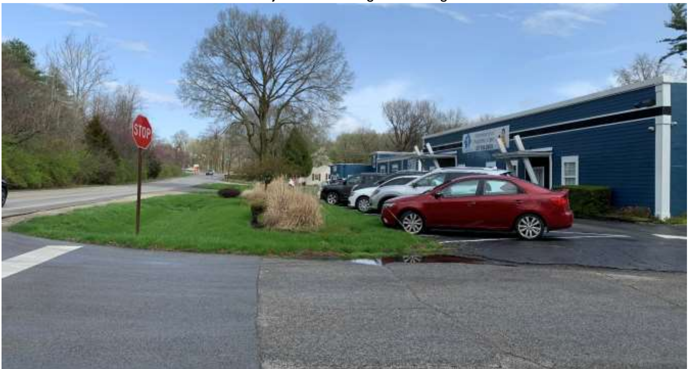
Photo of 7405 Westfield Boulevard looking north on the site.
