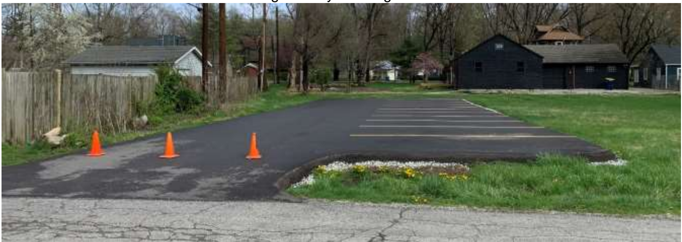
Photo of a parking lot at 7429 Westfield Boulevard that received a zoning violation.
