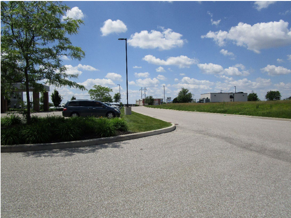
View looking south along Belfast Drive
