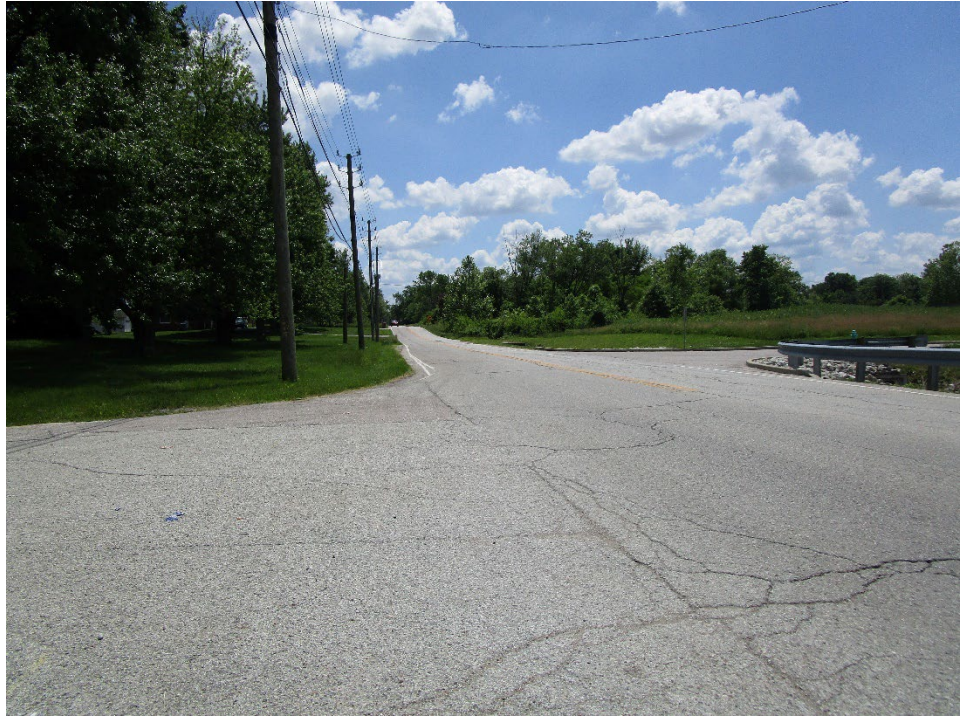
View looking south along Flynn Road
