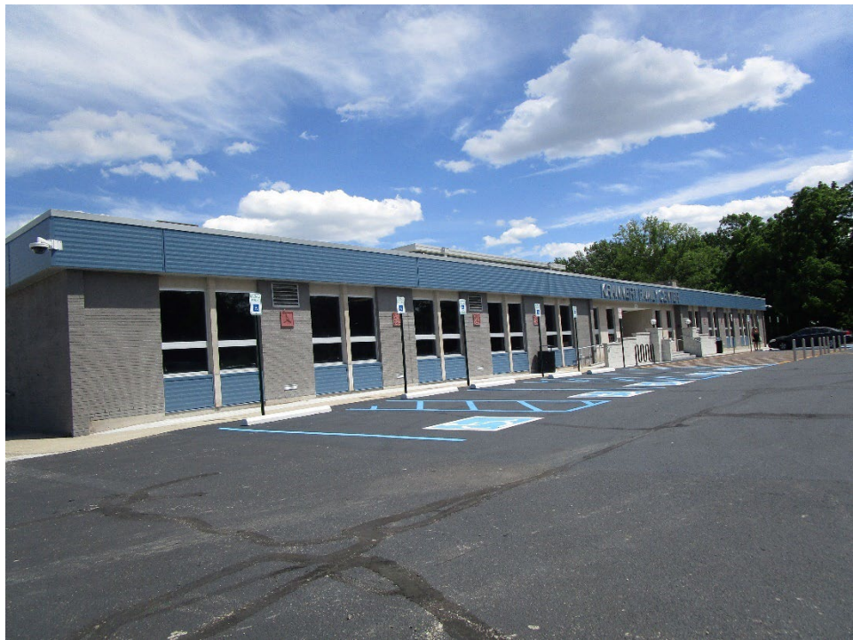
View of community building looking southeast
