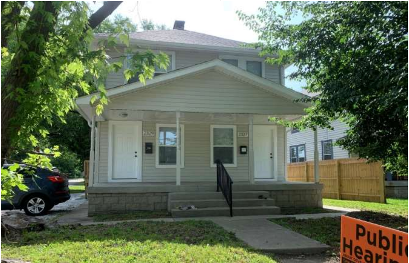
Close up view of the existing duplex.
