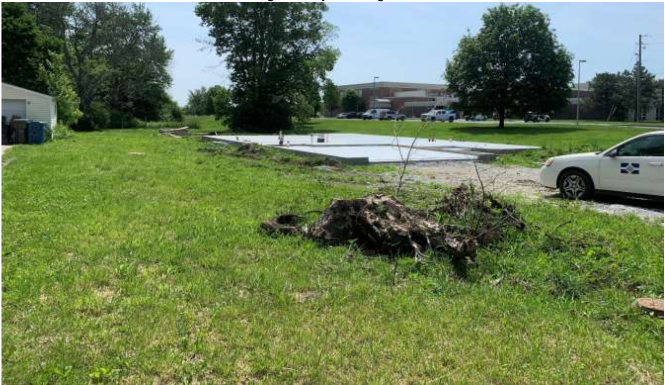
Photo of a residential dwelling under construction east of the site.
