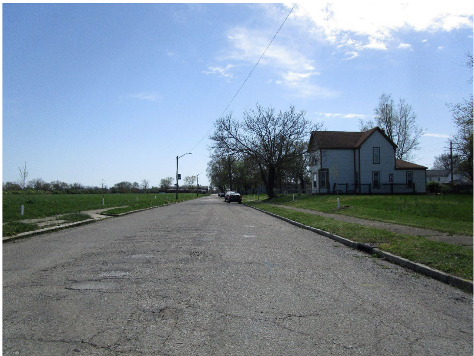
View looking south along Winthrop Avenue
