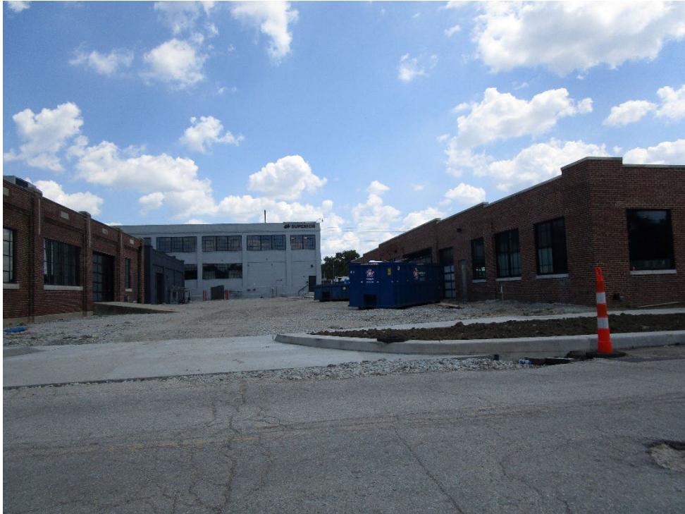
View of eastern portion of site looking south across Roosevelt Avenue
