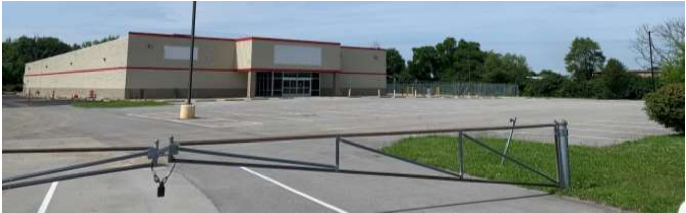
Vacant commercial building west of the site.
