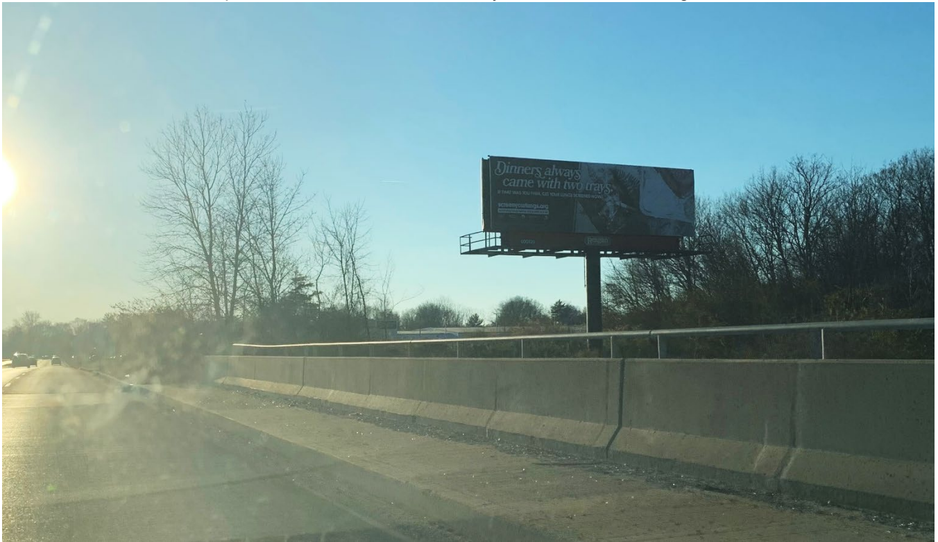
Existing bridge on Pike Plaza Road frontage of Lot Two, looking west
