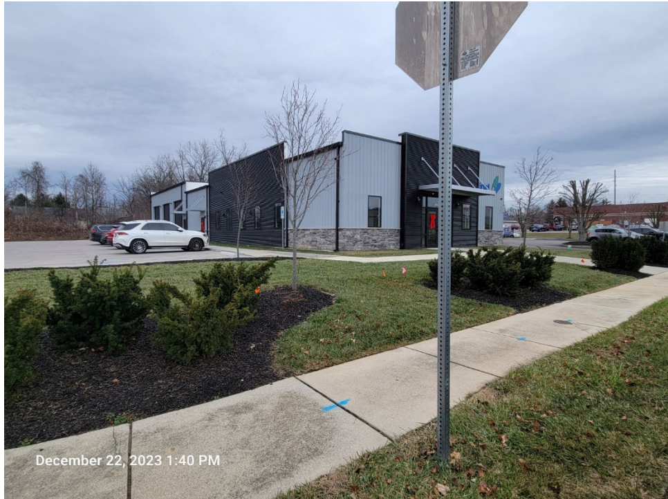
Figure 4 - Existing building on proposed Lot 6B
