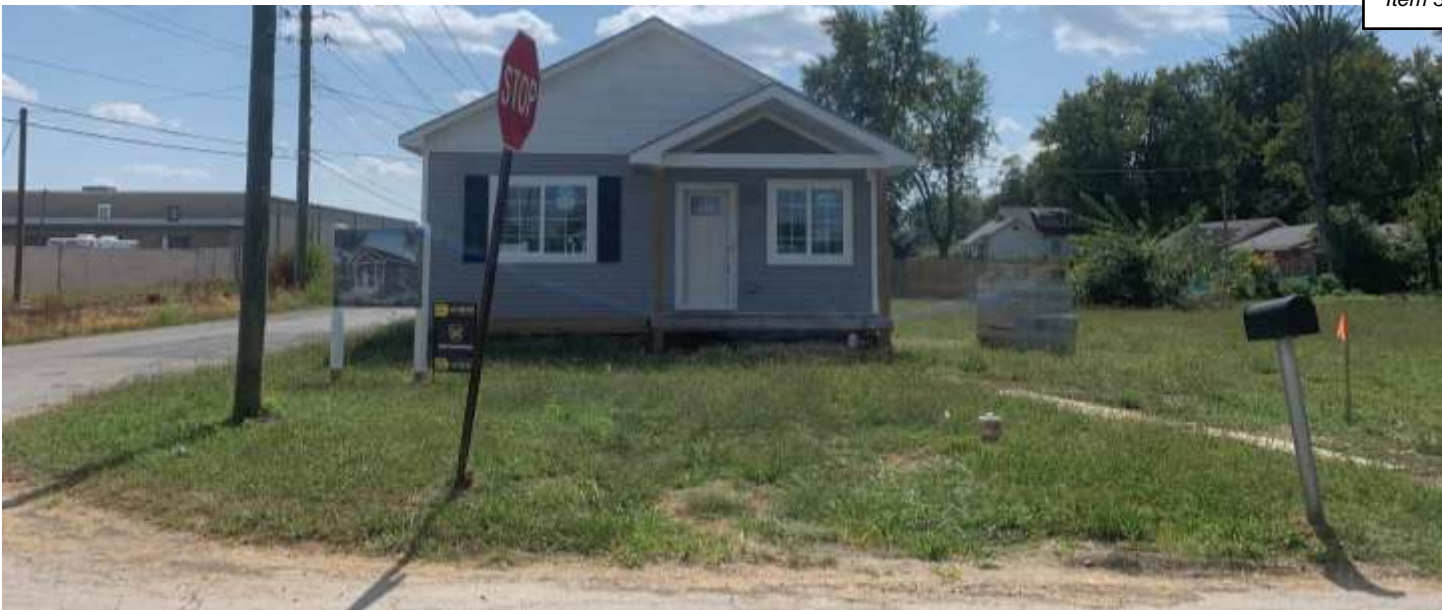
Photo of the single-family dwelling east of 4505 West Caven Street.
