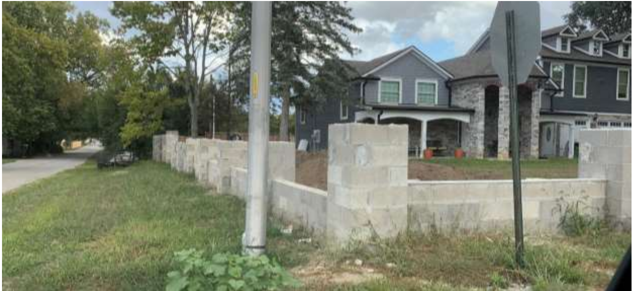
View of fence along Chelsea Road, looking east
