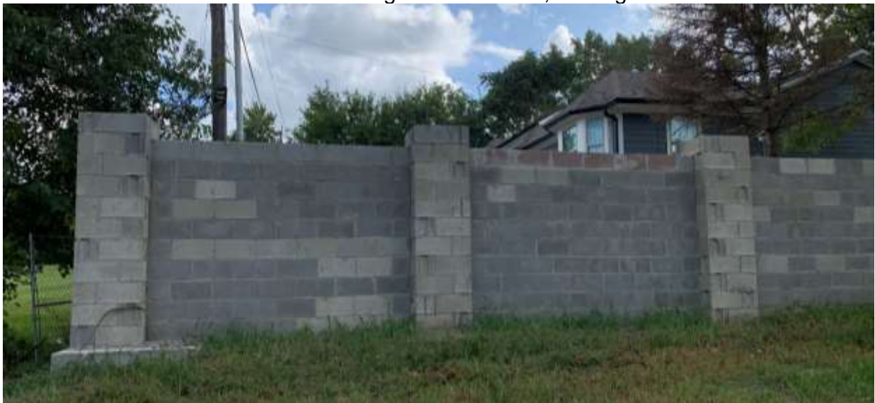
View of fence along Chelsea Road, looking south
