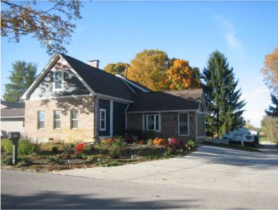
Subject site existing dwelling, looking north.
