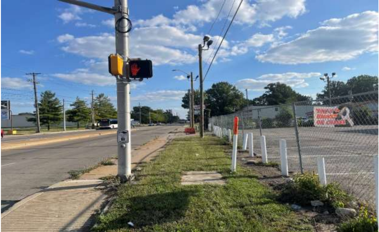
Photo One: Looking South Along Arlington Avenue
