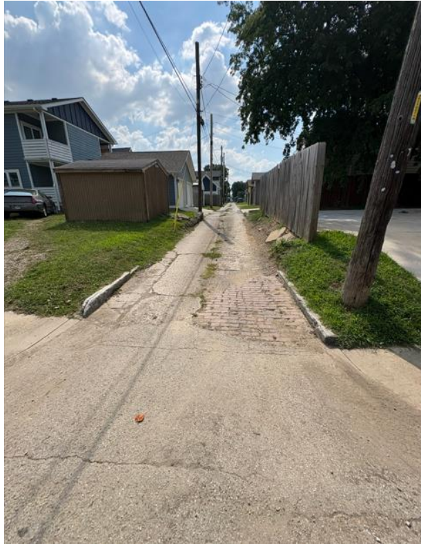
Photo 5: Subject Site View of Rear Alley Access
