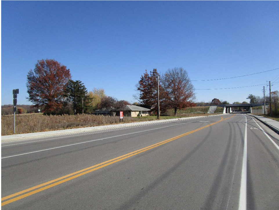
View of site looking east along Wicker Road
