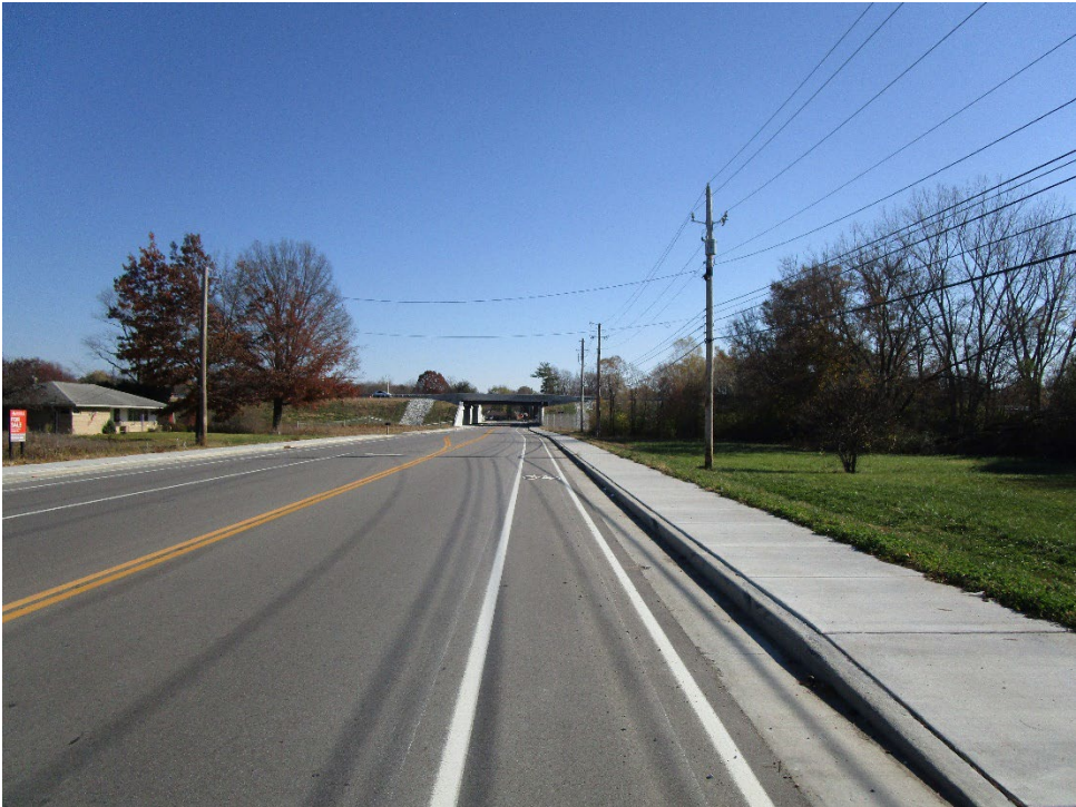
View looking east along Wicker Road
