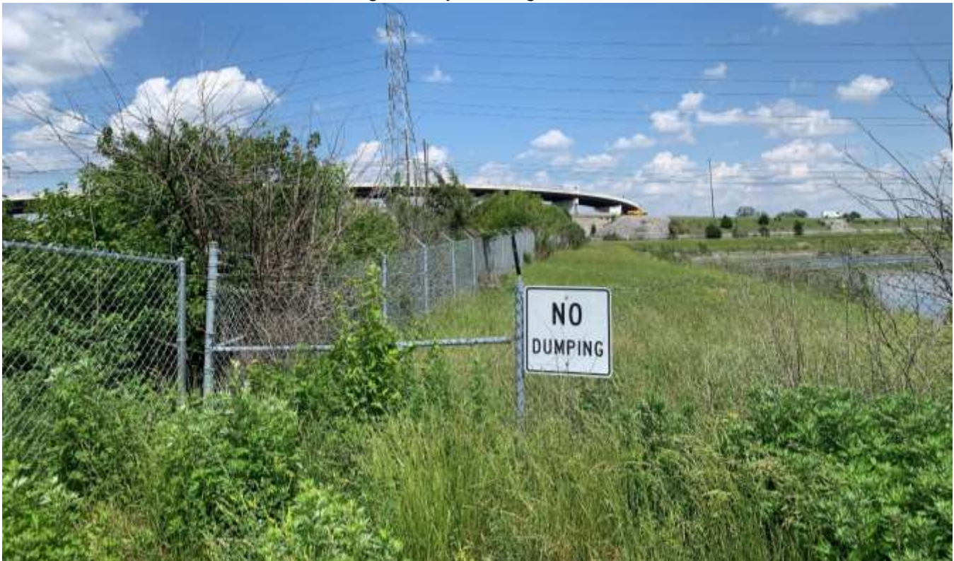
Photo of the southern property boundary fence looking east.
