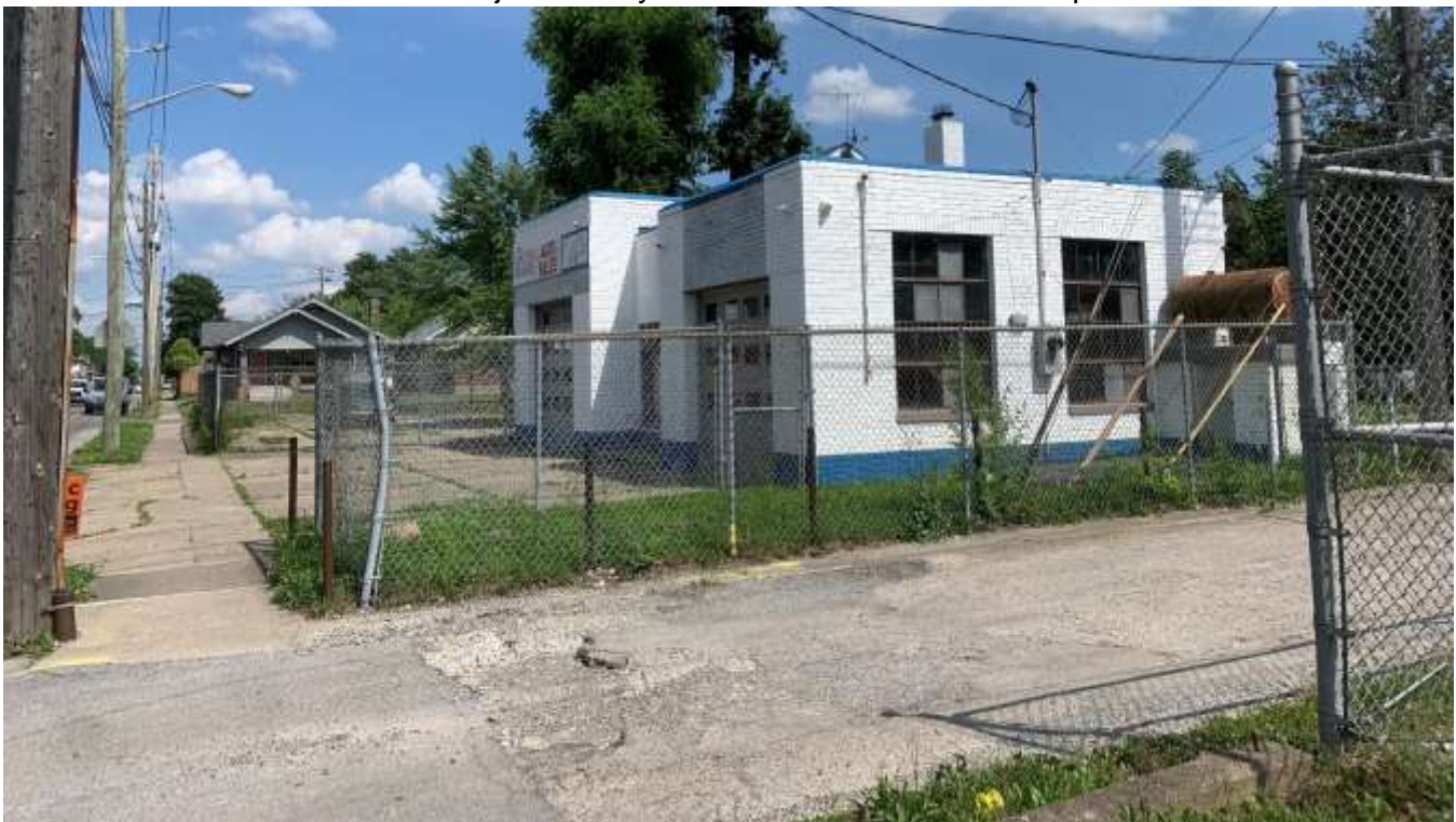
Photo of the subject site looking east.
