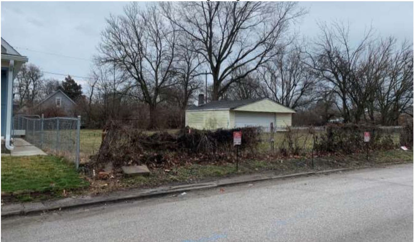
Photo of the existing detached garage on the subject site.
