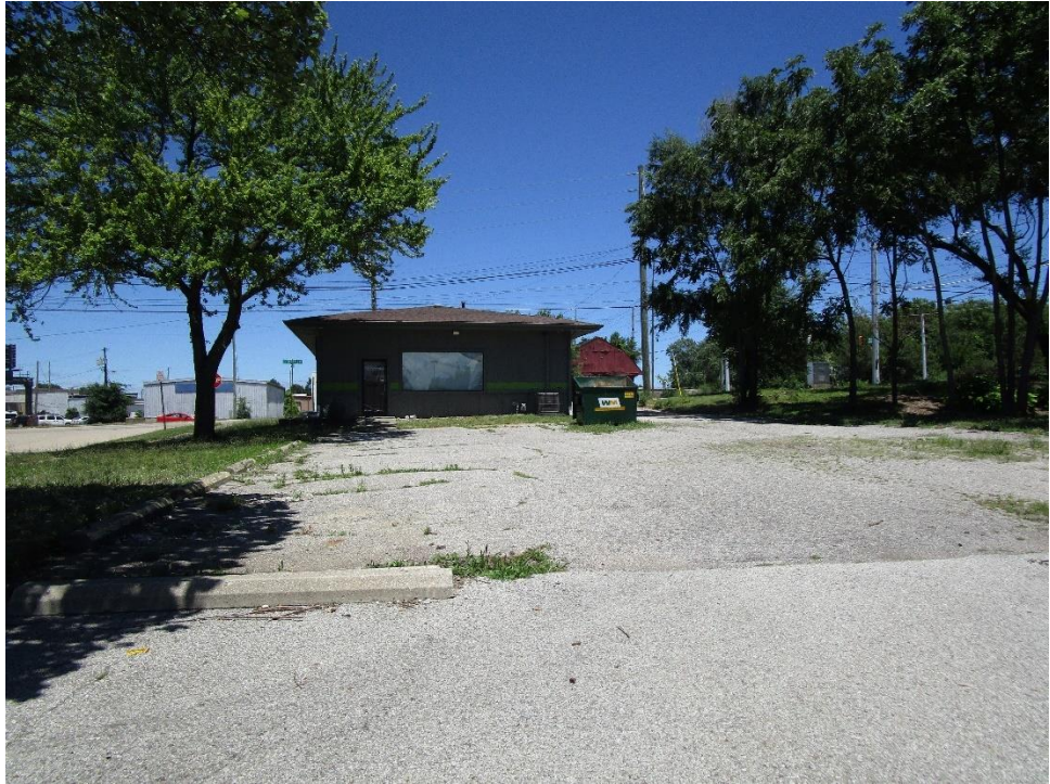
View of site looking north
