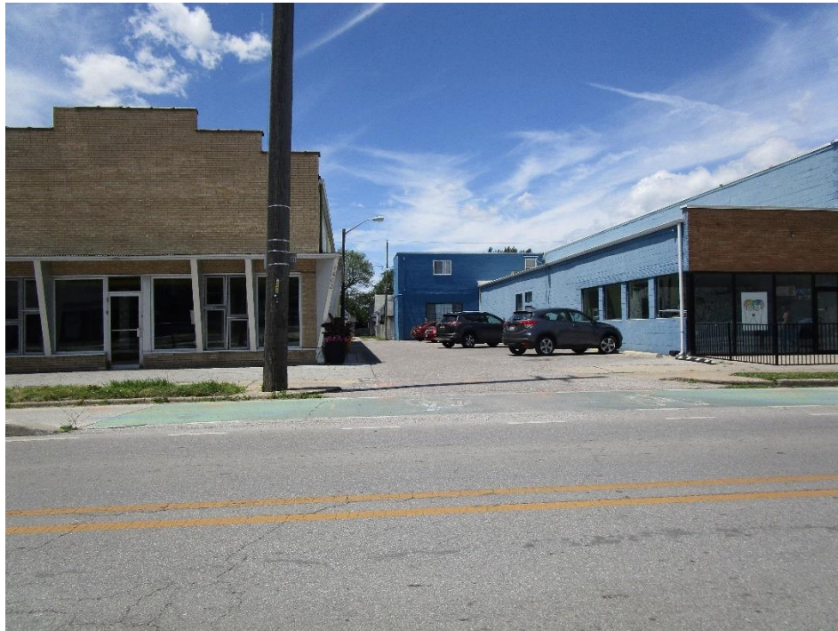
View of site looking west across Shelby Street
