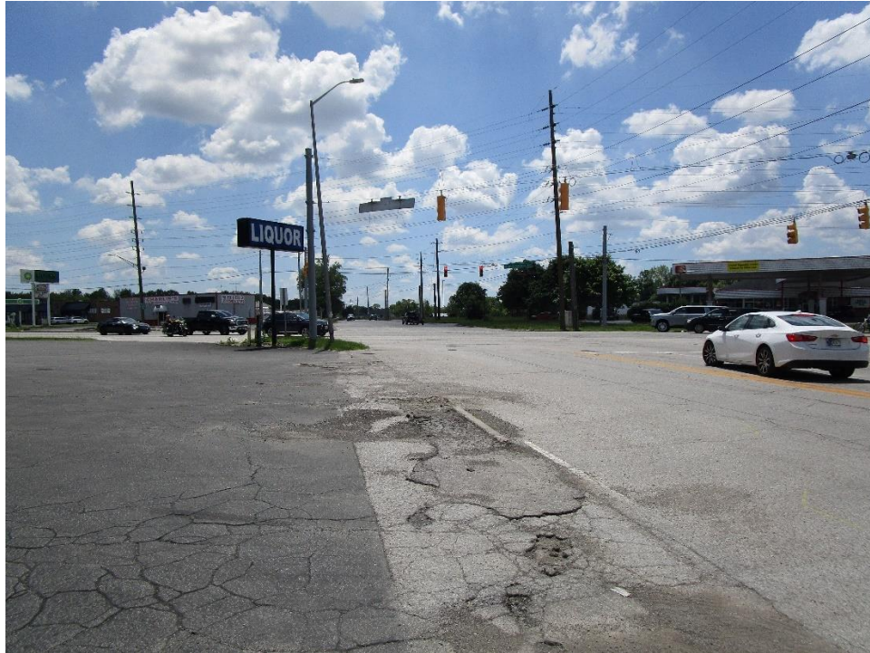
View looking south along South Arlington Avenue
