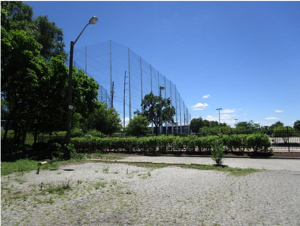
View from site looking south
