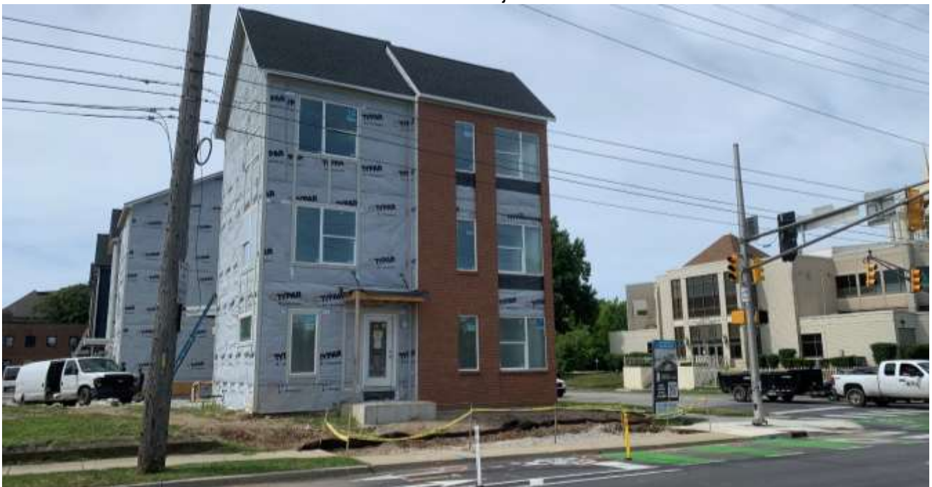
Photo of townhomes west of the site.
