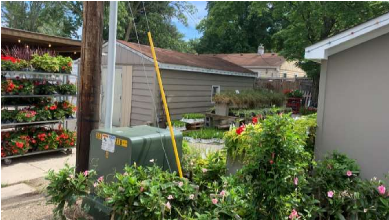
Photo of the existing detached garage to be demolished looking northeast towards the fence line.
