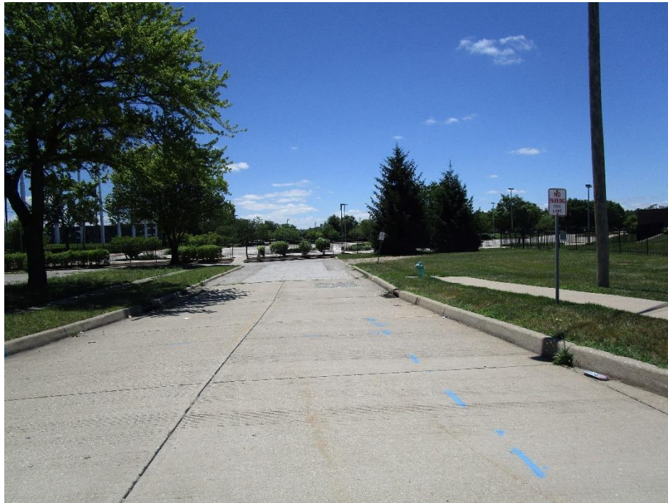
View looking south along Bridge Street
