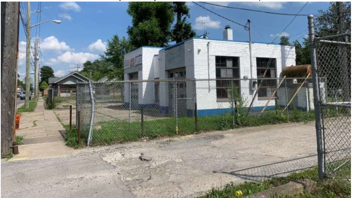
Photo of the subject site looking east.
