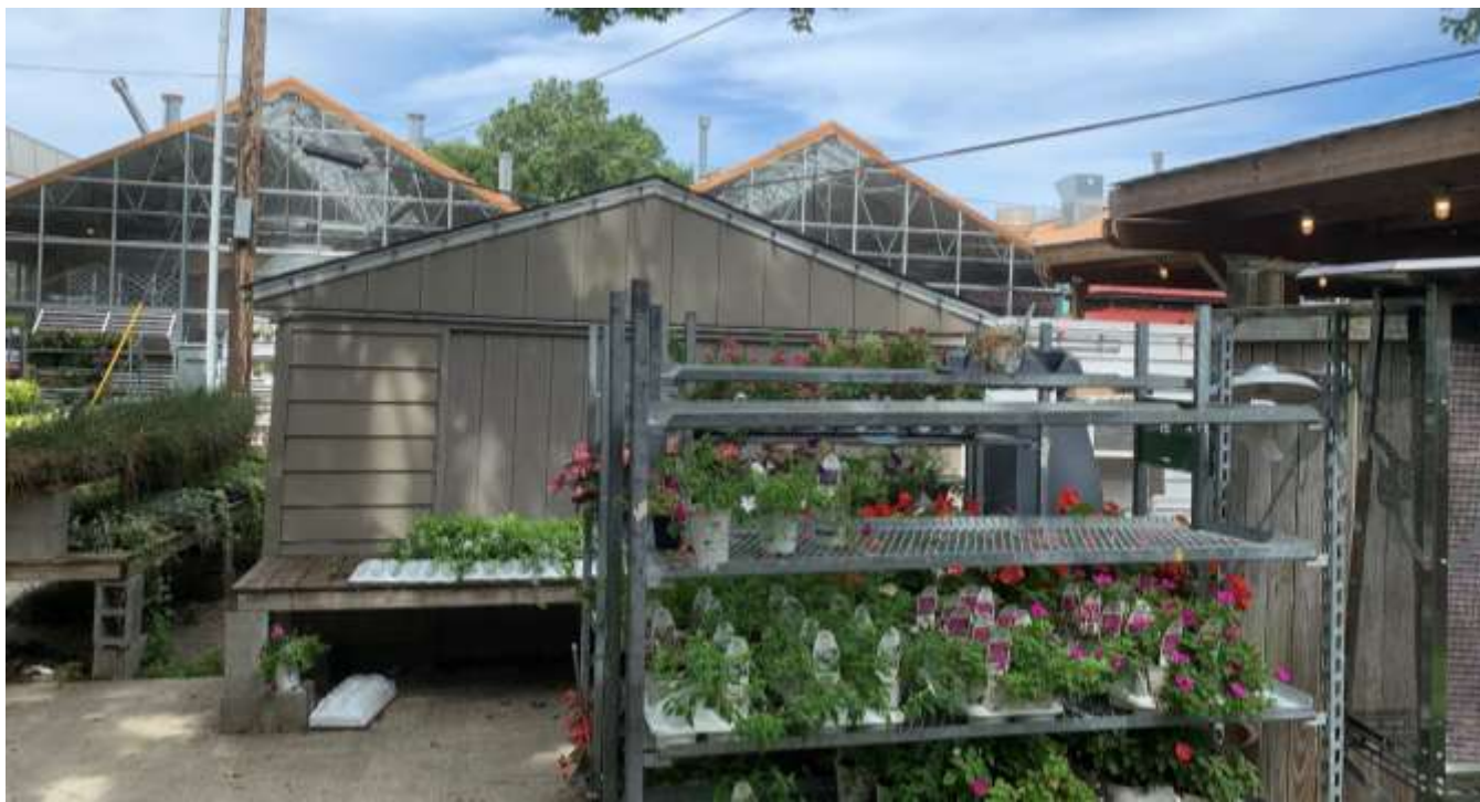
Photo of the existing detached garage to be demolished on the west side of the existing fence line.
