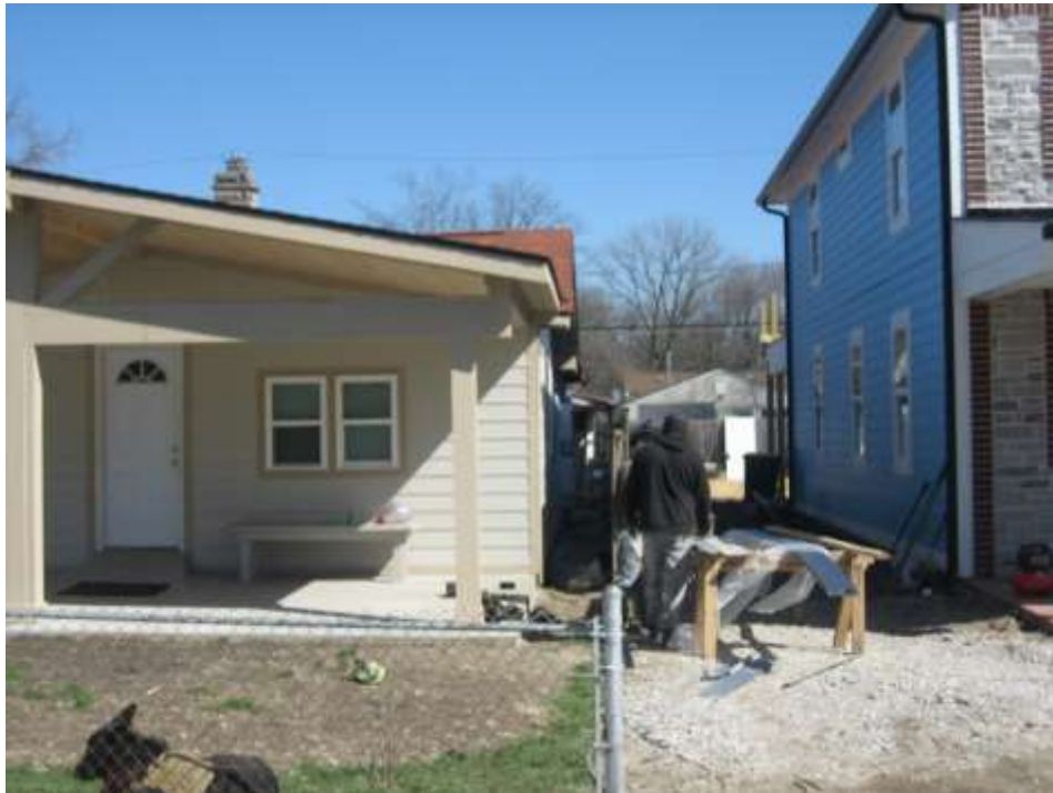
Photo of the existing single-family dwelling zzero-foot south side setback, looking east.
