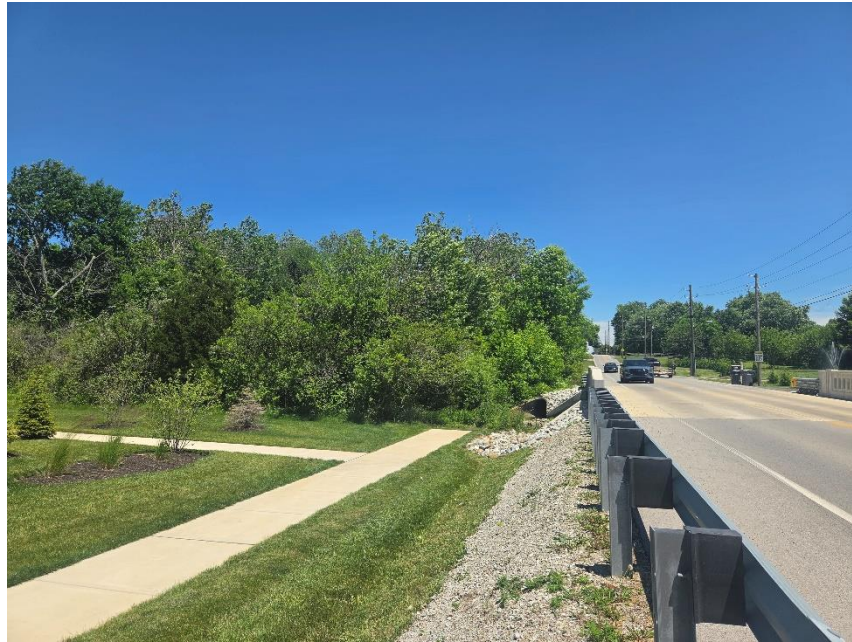
Photo 3: Horn Creek Bridge Viewed from West
