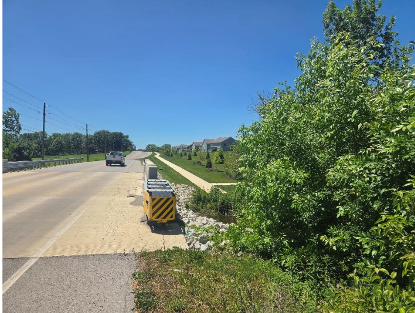
Photo 5: Horn Creek Bridge Viewed from East
