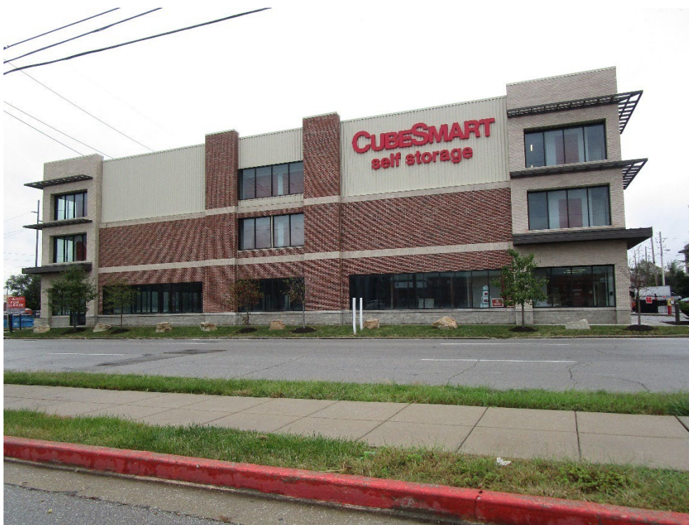
View of site looking east across North Illinois Street
