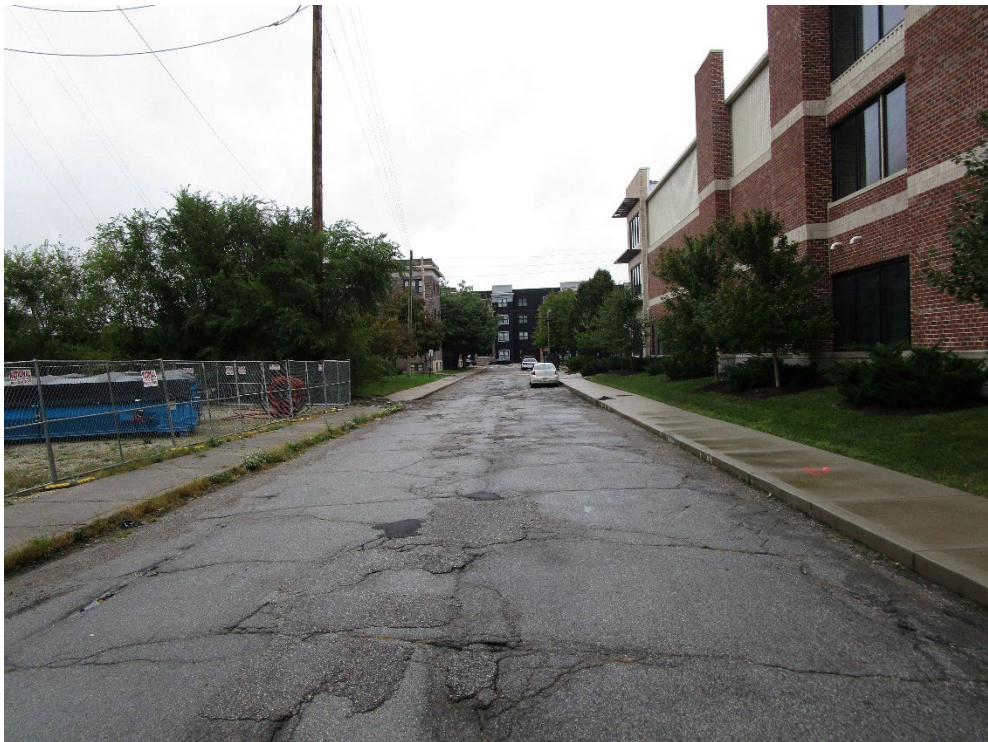
View looking east along Mc Lean Place
