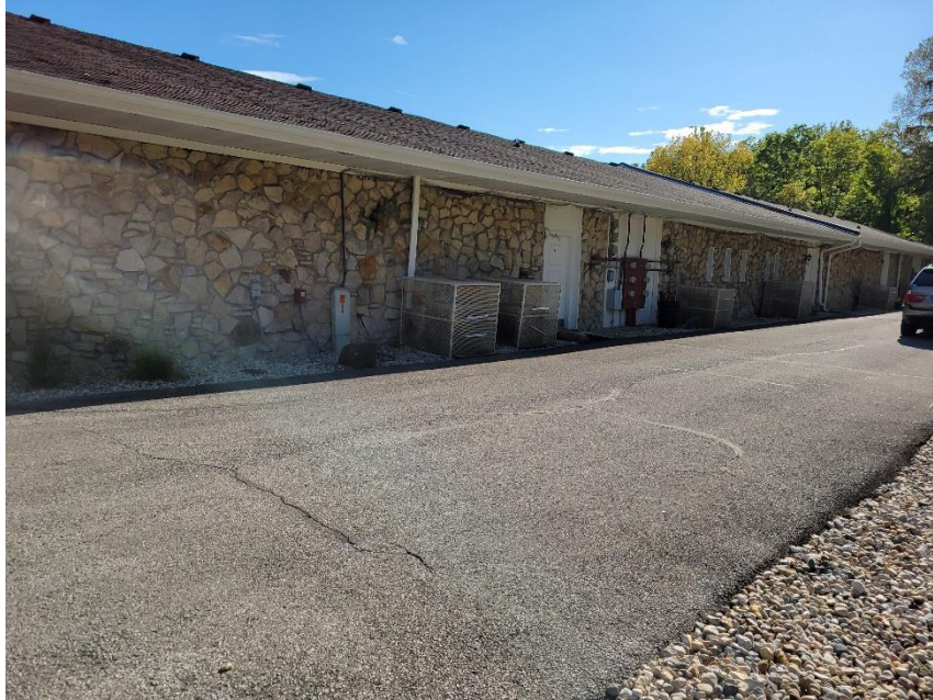
Photo 5: Subject Site viewed from North
