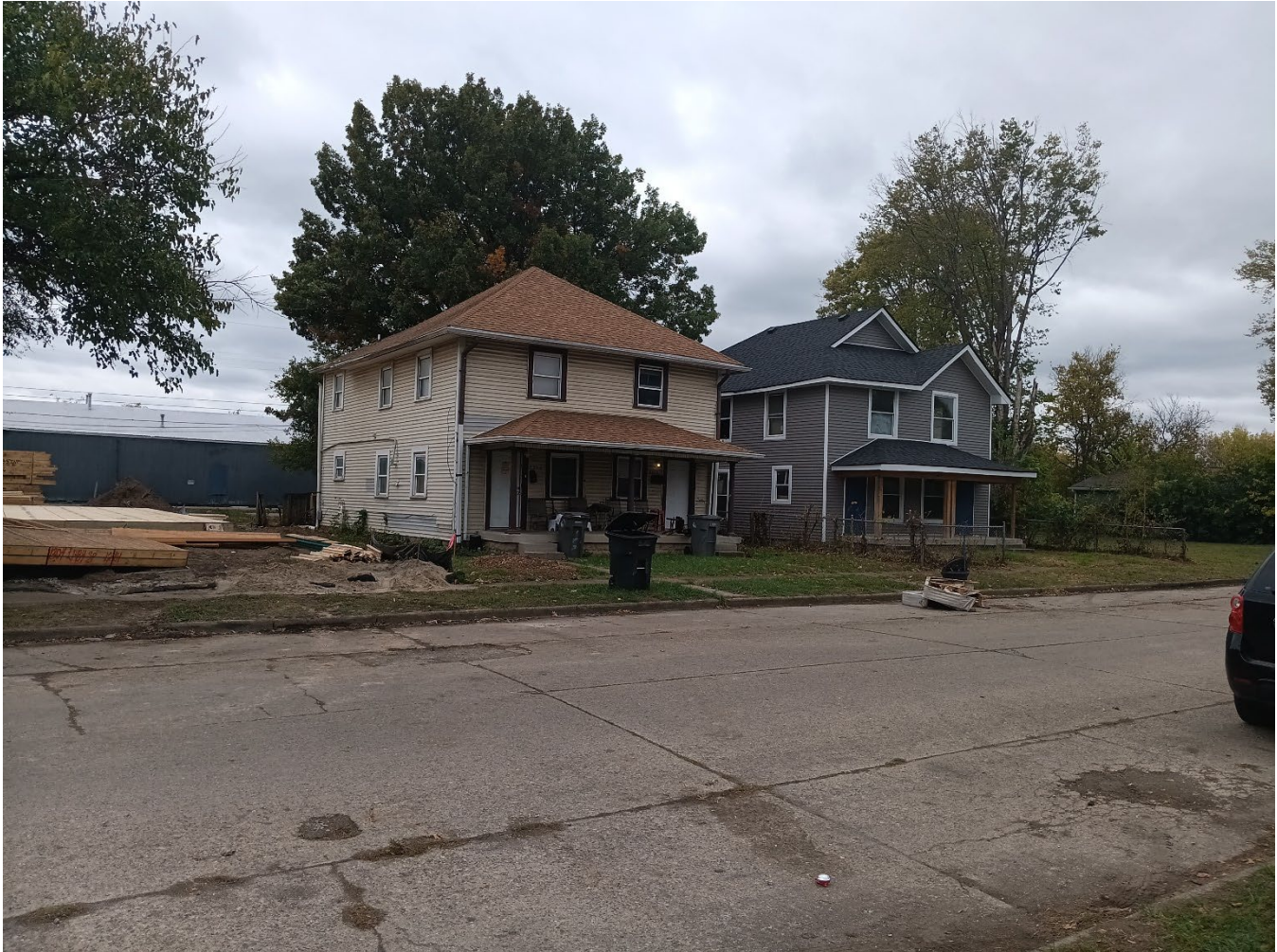
Exhibit 8: Two story duplexes that sit to the northwest of 2511 Columbia Avenue.
