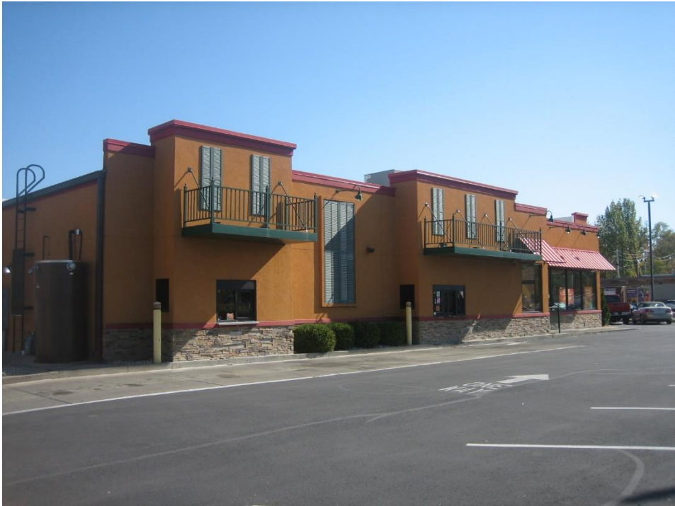
Subject site drive thru stacking spaces in front yard of North Keystone Avenue, looking southeast.
