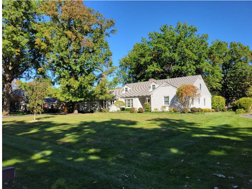
Photo 7: Adjacent Property to North
