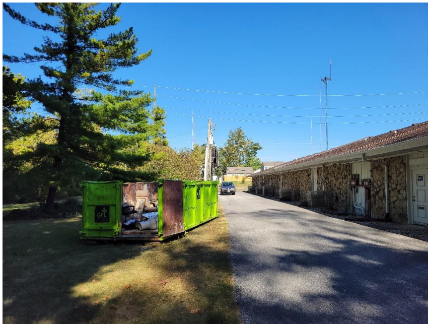
Photo 6: Rear of Building (multiple tenant bays)
