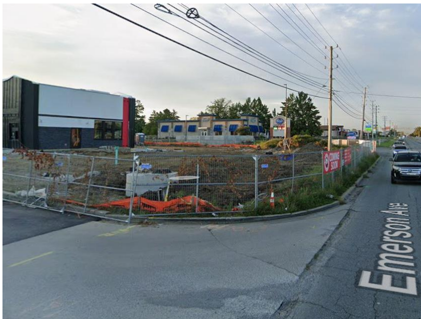
Photo 2: Subject Site from Northwest (September 2024)
