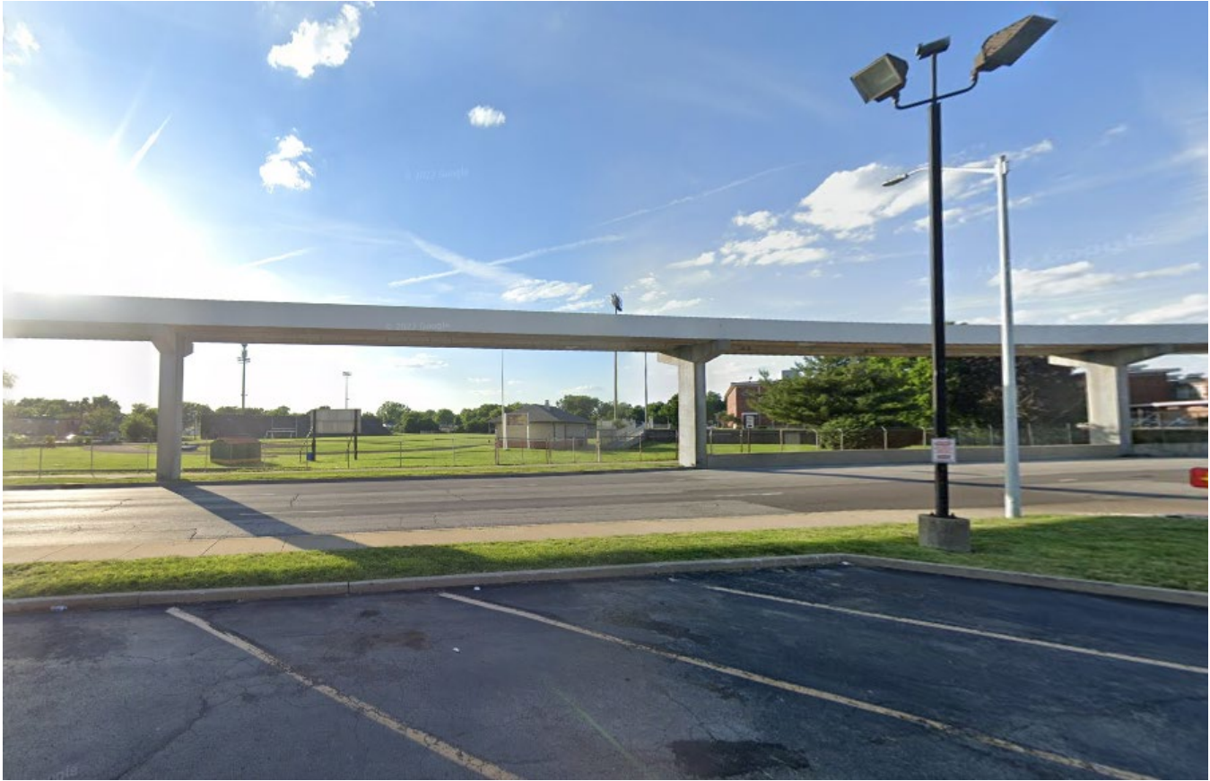
Approximate location of proposed wireless communication facility along Oscar Robertson Boulevard
