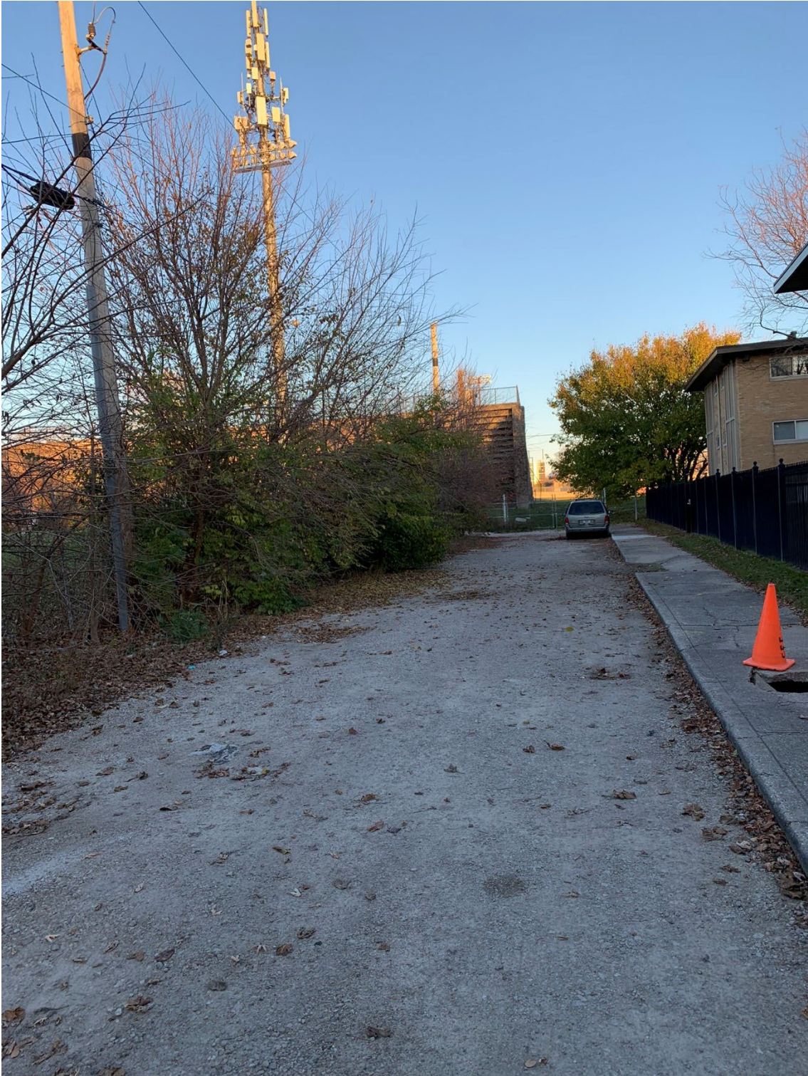
Existing wireless communications facility from vacated 11 th Street (private access to site)
