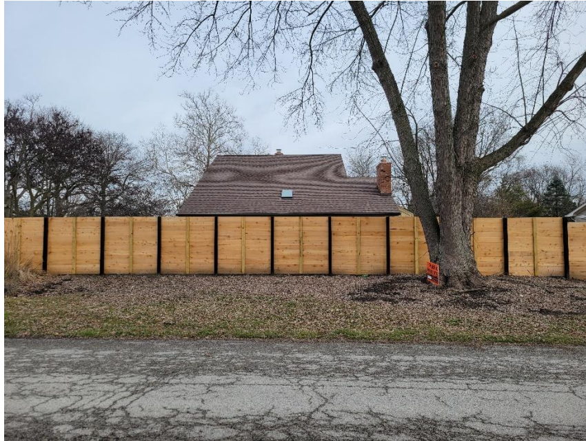
Photo 1: Fence from Front Yard (West)
