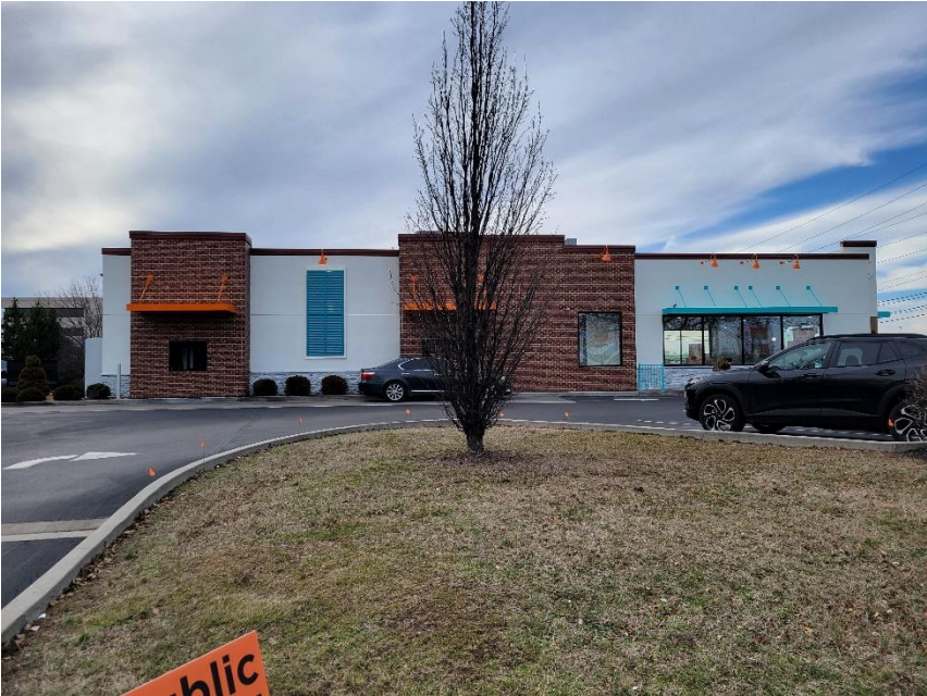
Photo 1: Eastern Elevation (Front Yard)
