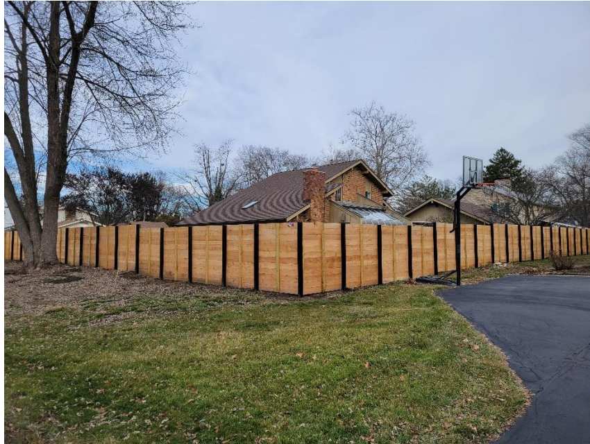
Photo 3: Fence from Southwest
