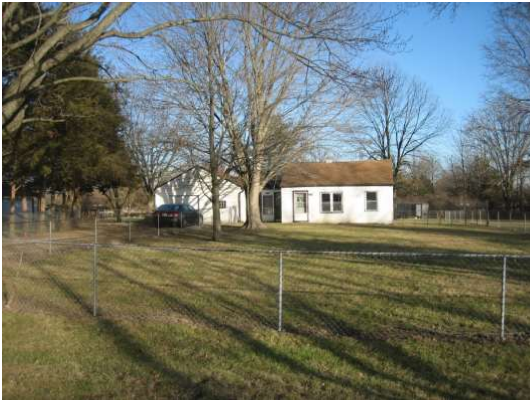
Subject site 2745 Curry Road existing dwelling, looking east.
