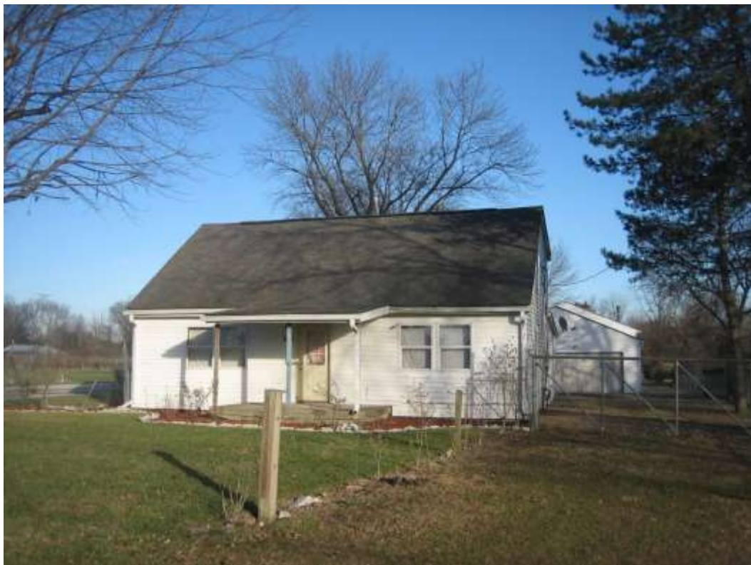
Subject site 2815 Curry Road existing dwelling, looking east.
