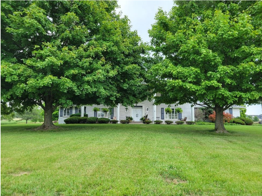
Photo 1: Existing House viewed from West
