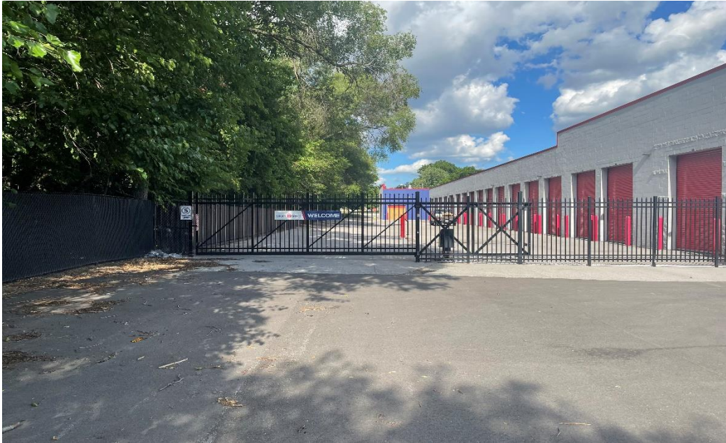
Photo Five: Existing Fencing Within North Side Yard
