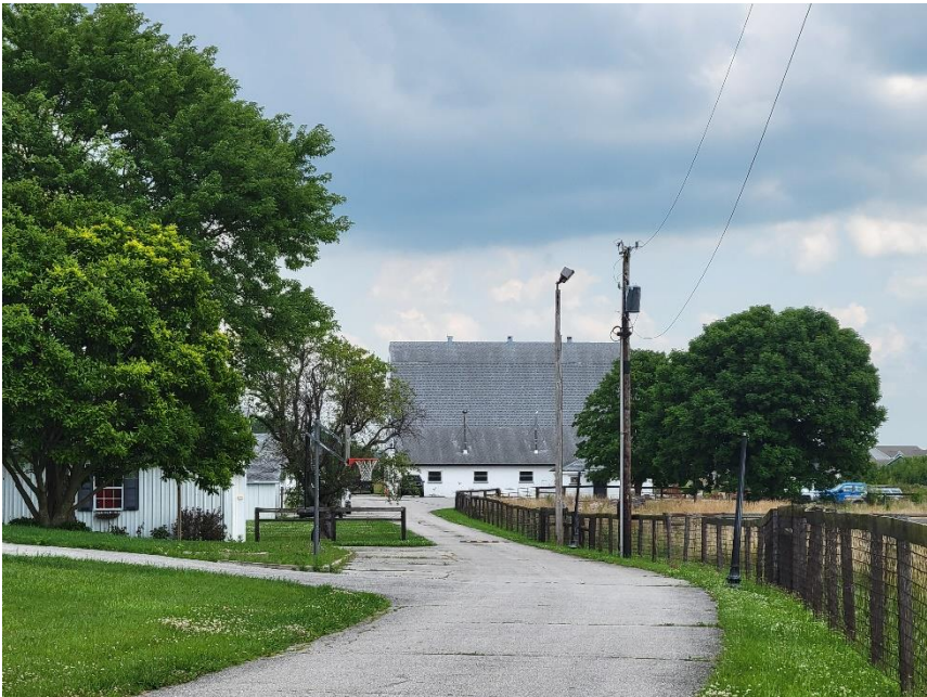
Photo 2: Existing Rear Buildings viewed from West
