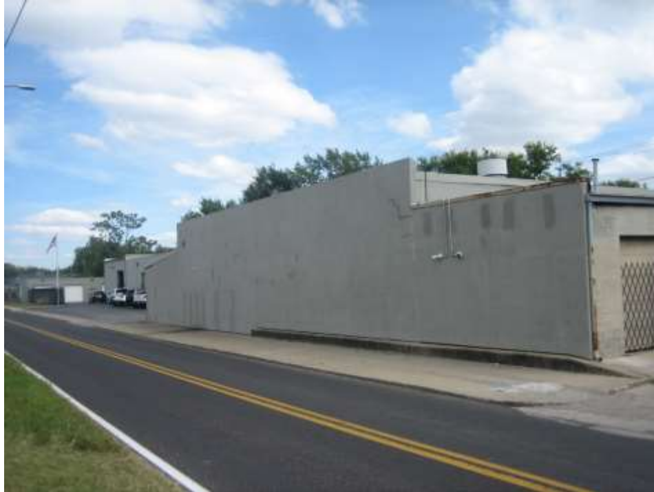
Subject site 2343 Massachusetts Avenue frontage, looking northeast
