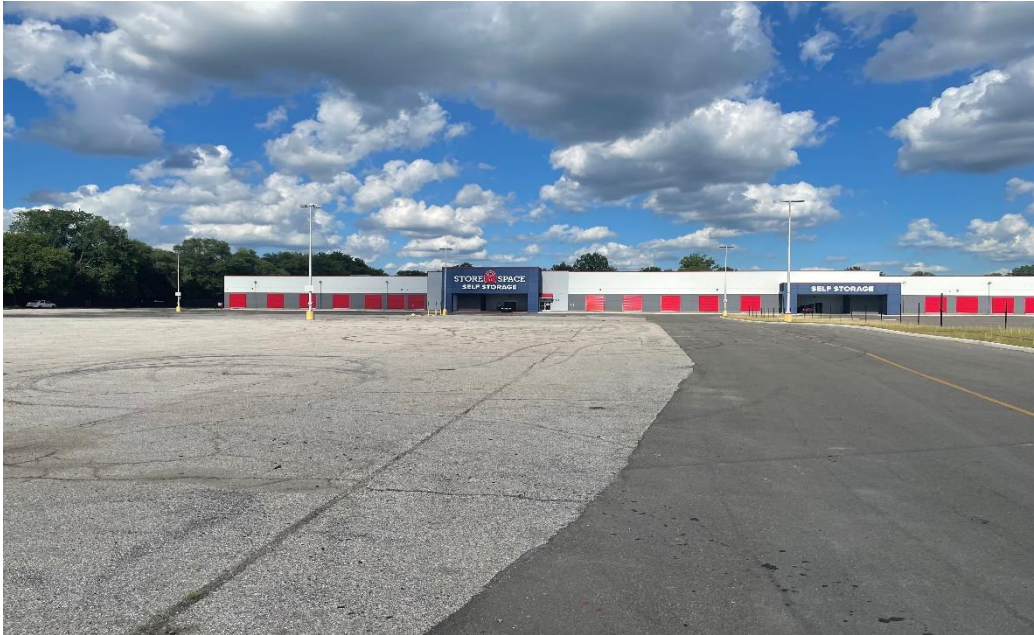
Photo Three: Primary Building, Facing East
