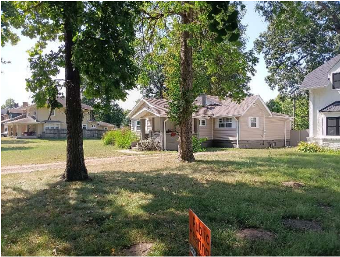
Exhibit 10: The homes south of 3450 Winthrop Ave.
