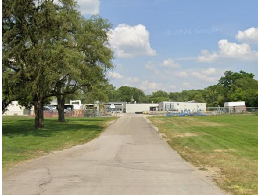
Photo 17: Subject Site Viewed from Emerson (June 2024)
