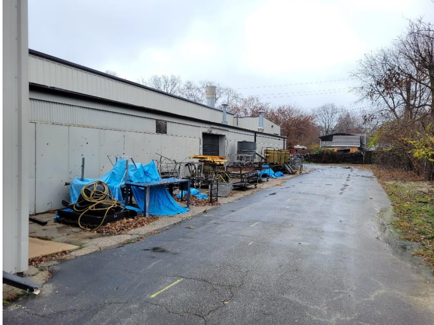
Photo 11: Portion of Primary Building (Southeast)
