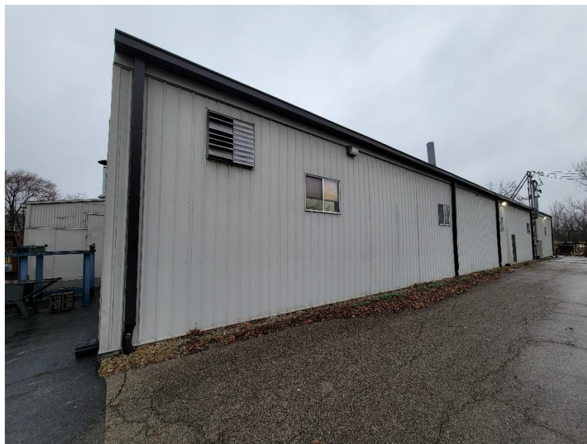
Photo 10: Primary Building Viewed from Southeast
