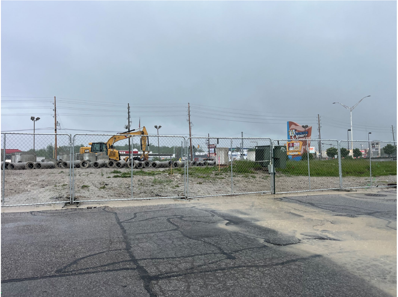
Photo 1: Subject site from mall parking lot
