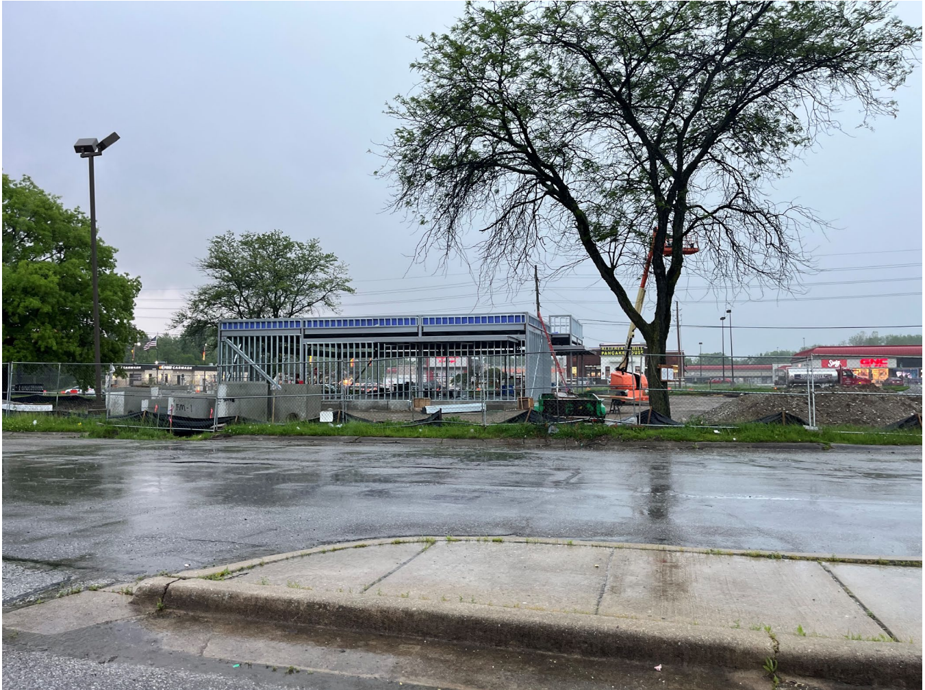
Photo 2: Framing of bank at subject site
