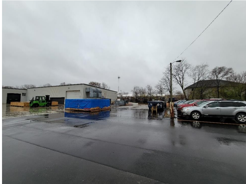
Photo 7: Southern Storage Area Viewed from Northwest
