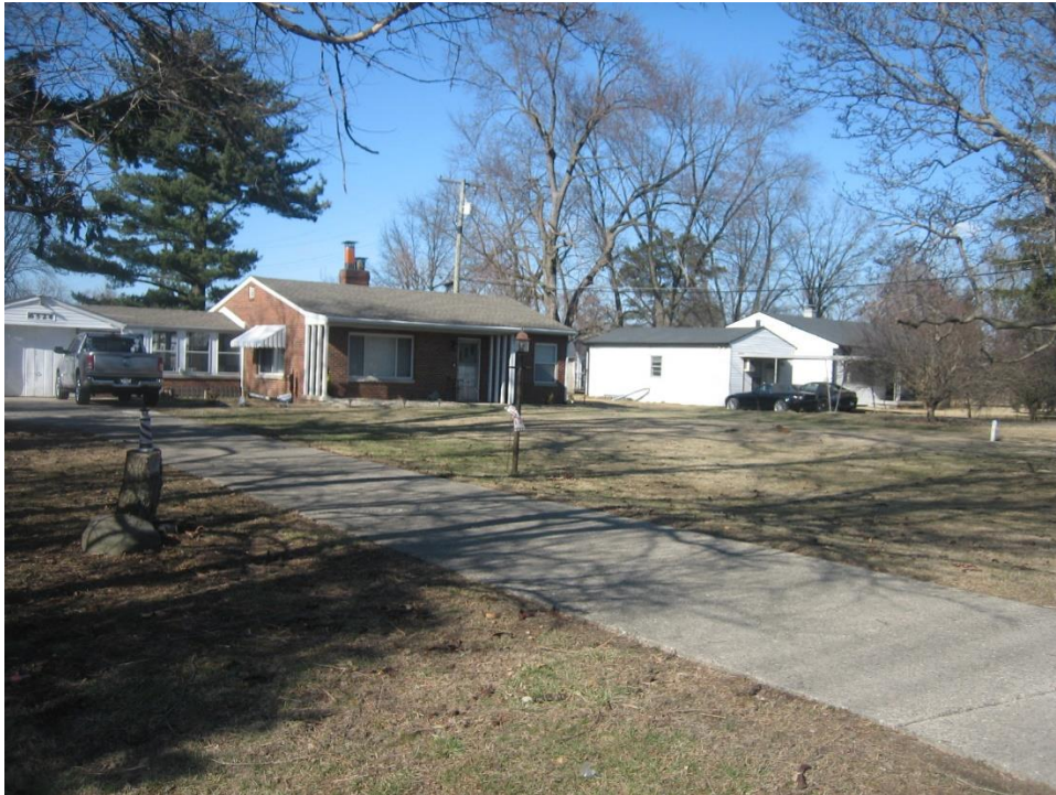
Adjacent single family dwellings zoned D-3, to the east, looking northeast
