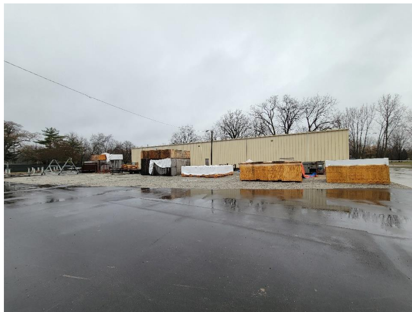
Photo 2: Accessory Building & Northern Storage Area Viewed from South
