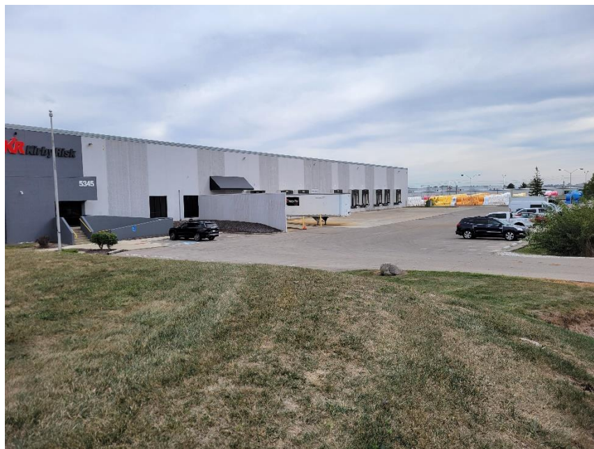
Photo 2: Existing Building & Parking Area Viewed from West
