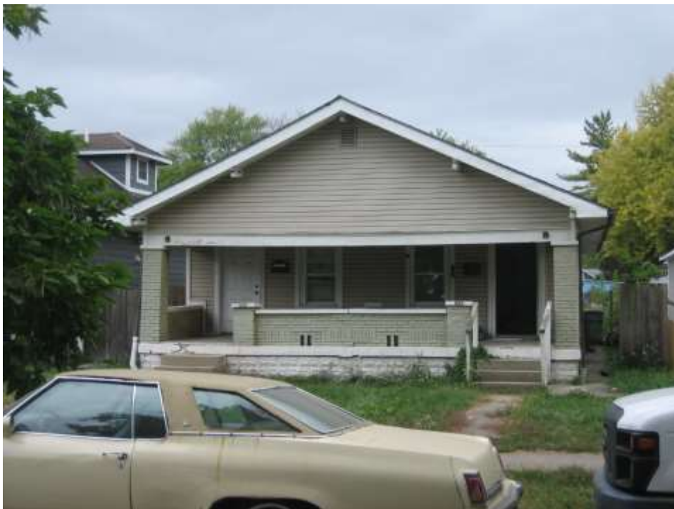
Adjacent property to the south, looking west.
