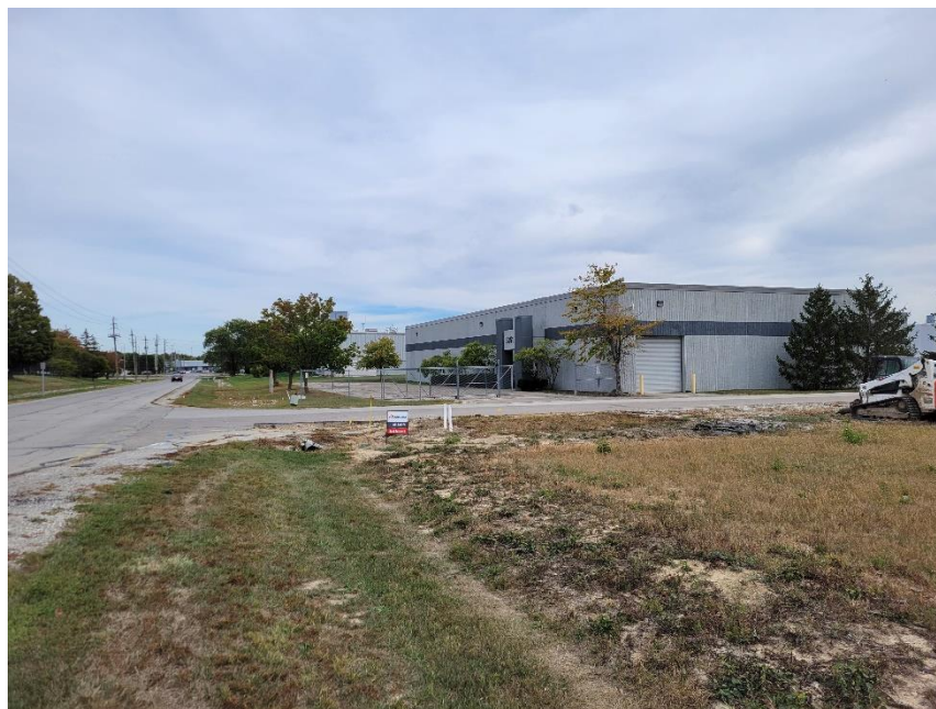
Photo 10: Adjacent Property to East
