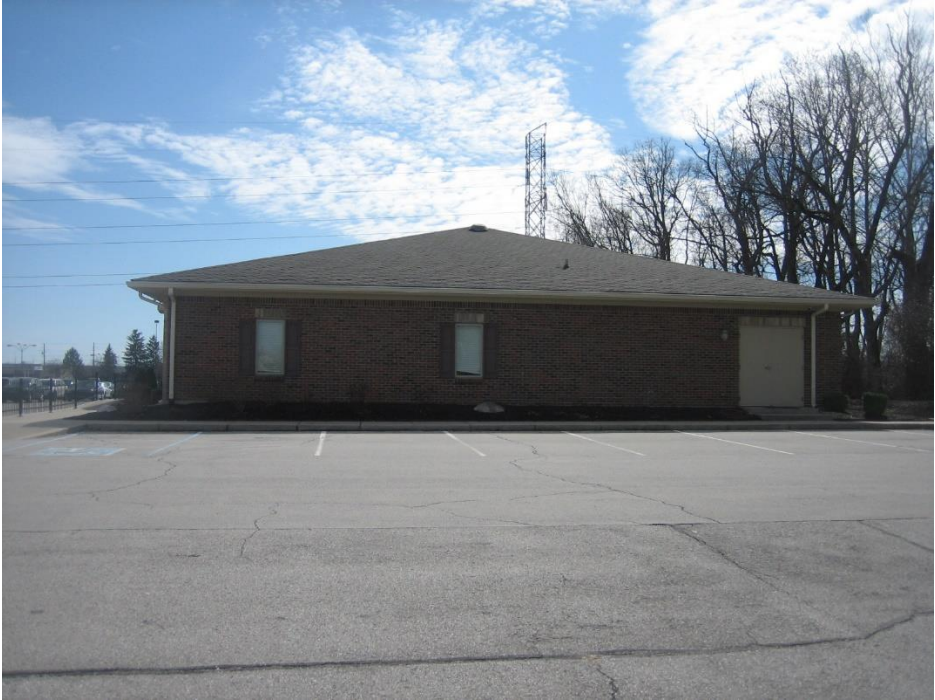
Subject site, looking south.
