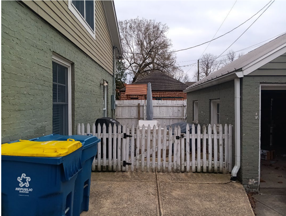
Exhibit 15: Space between the primary structure and existing garage that will be filled in by the proposed attached garage.
