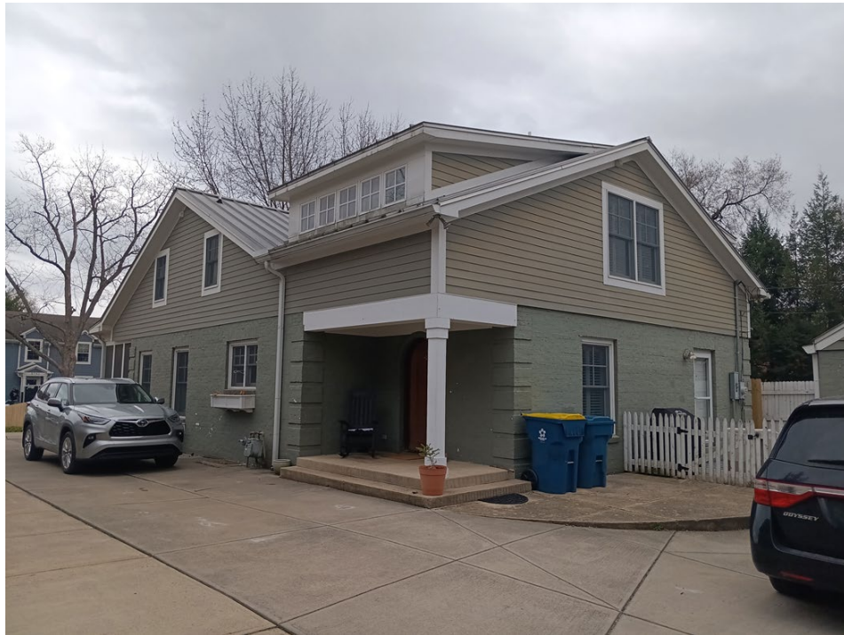
Exhibit 12: Looking southeast at the primary dwelling.
