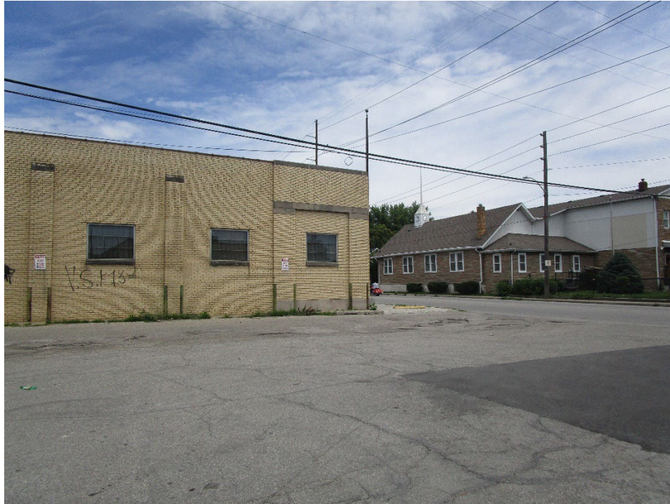
View of site looking northeast across east / west alley along the southern site boundary
