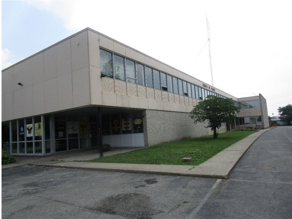
View looking southeast along existing building
