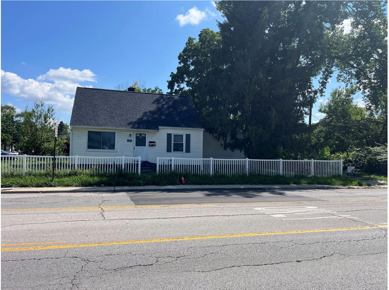
Photo 4: Looking south across 46 th Street
