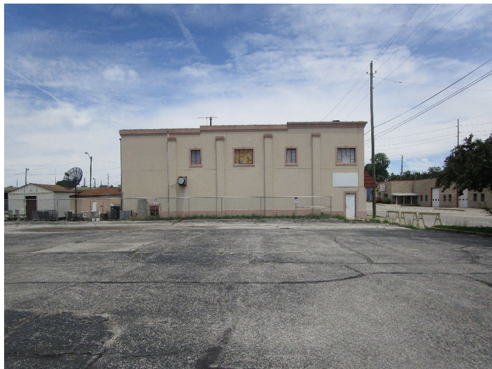
View from site looking north
