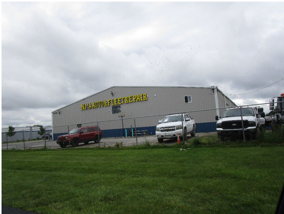
View of site looking southwest
