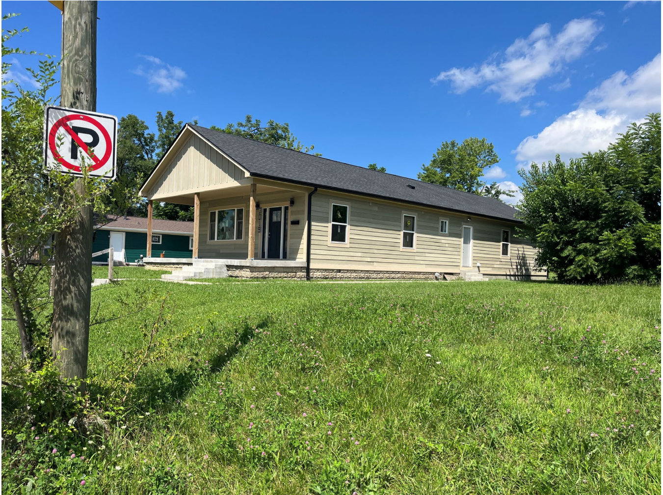
Photo 2: 3019 North Gale St (subject of 2023 rezone from SU-1 to D-5II)
