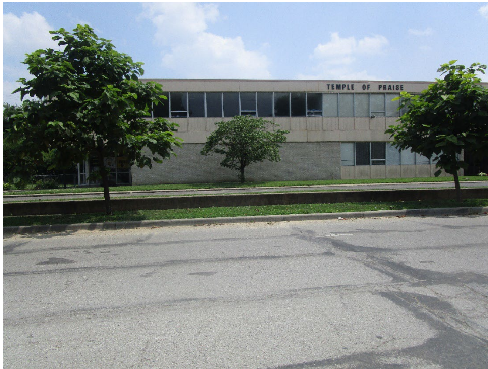
View of existing building looking east across Meadows Drive
