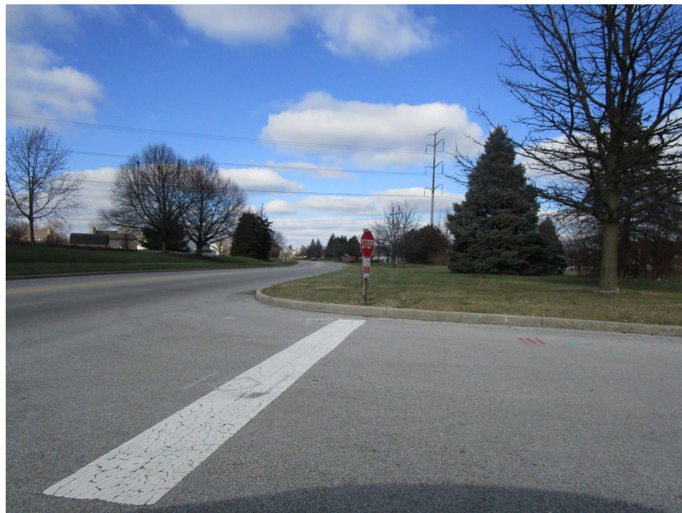
View looking north along Mc Farland Boulevard
