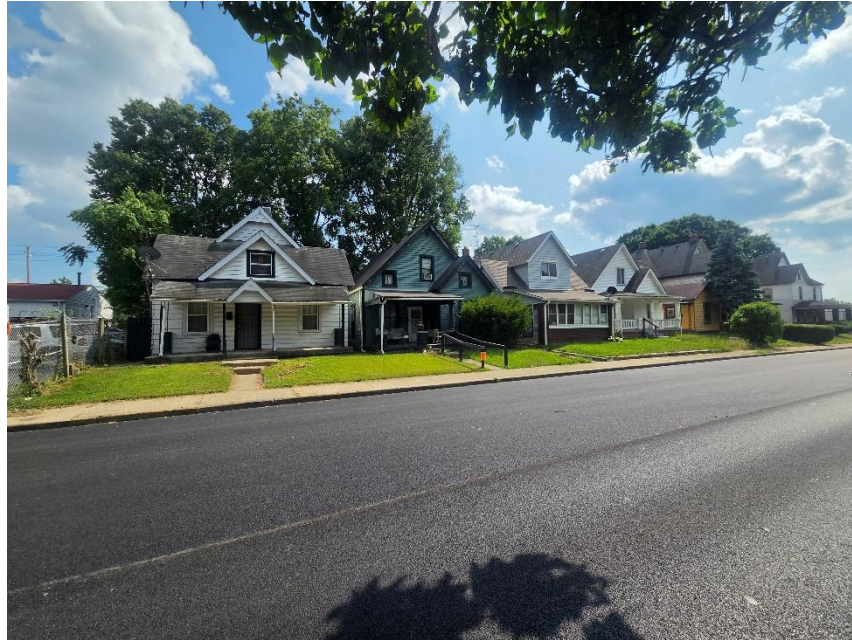
Photo 5: Adjacent Property to Southwest
