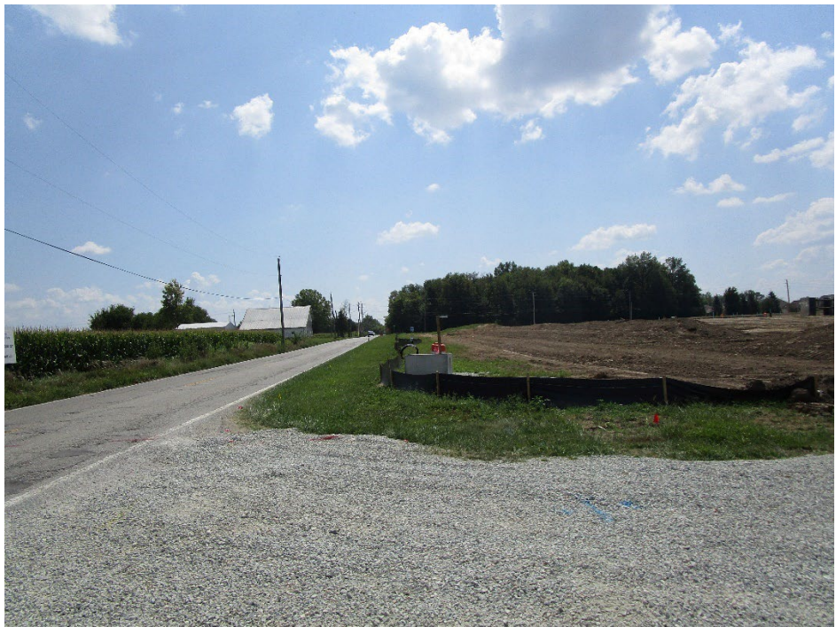
View looking south along North Carroll Road
