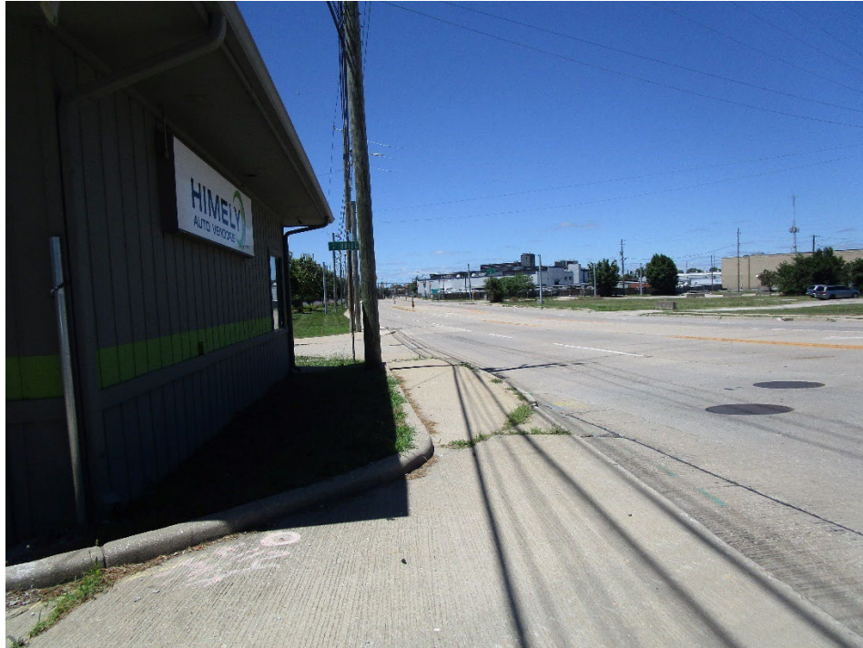
View looking east along West Morris Street
