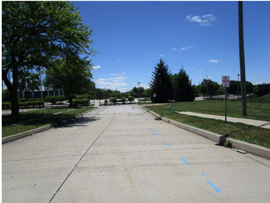
View looking south along Bridge Street
