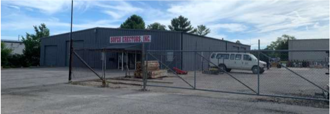
Photo of an industrial business east of the site.
