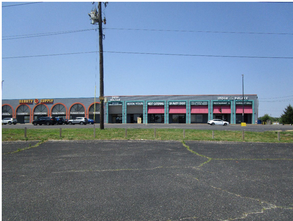
View from northern portion of site looking north
