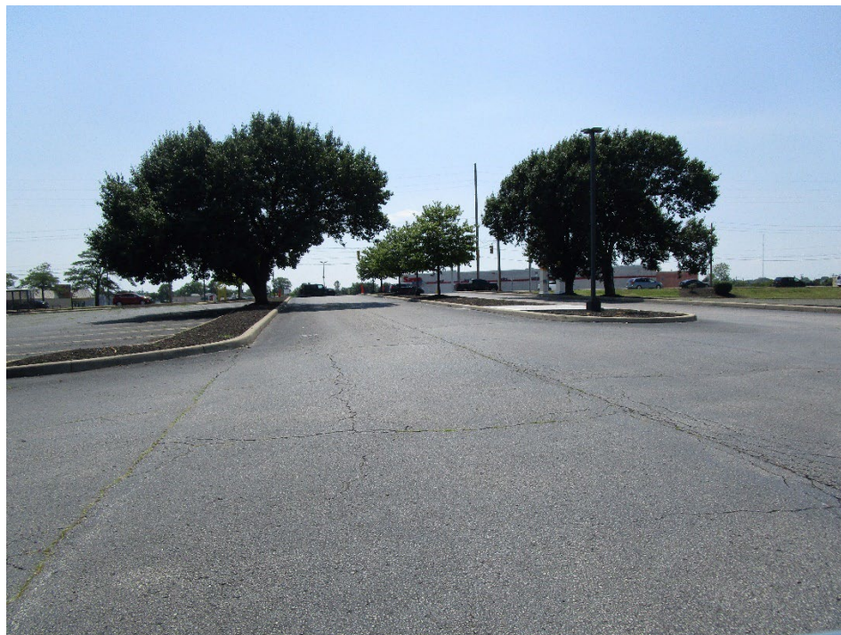
View looking west from entrance along Lafayette Road
