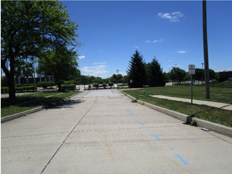
View looking south along Bridge Street
