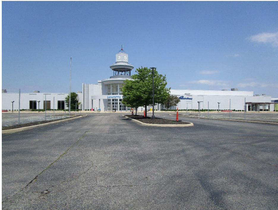
View looking east at main entrance along Lafayette Road
