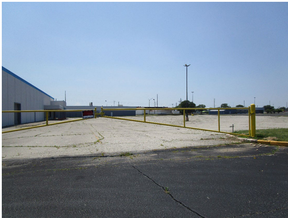
View of southern portion of site looking west
