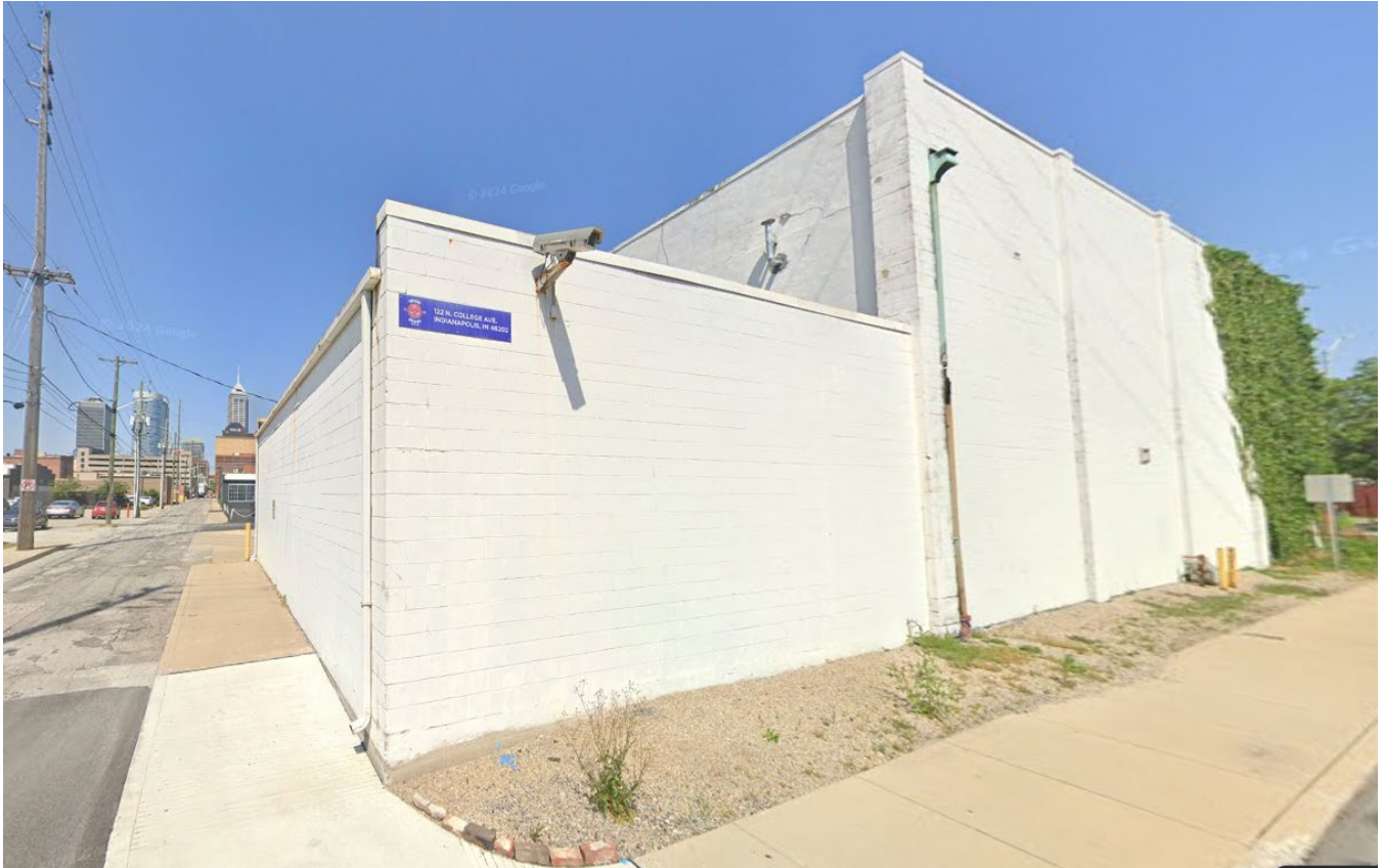
View of the warehouse structure along College Avenue
