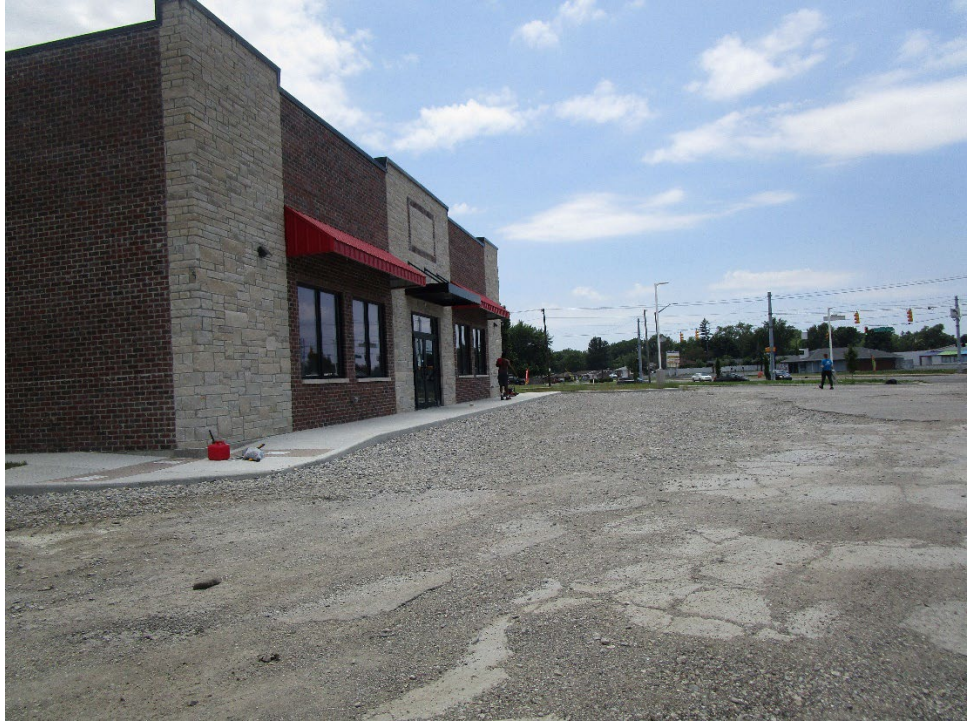
View of site looking south
