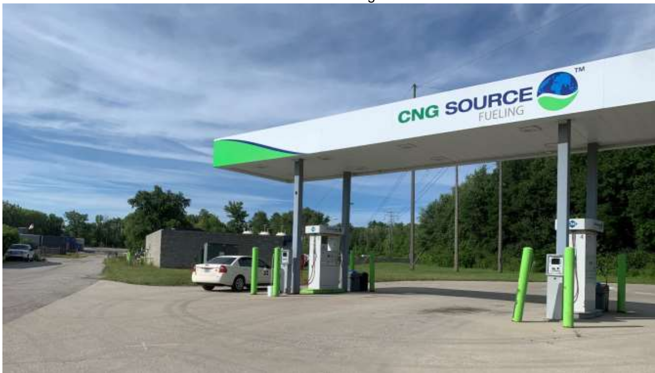
Photo of a fueling station at the north end of the site.
