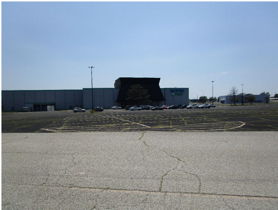
View of central portion of site looking west
