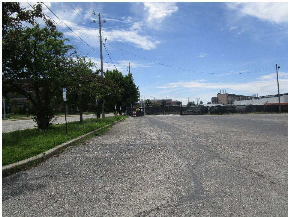
View from site south along Kentucky Avenue
