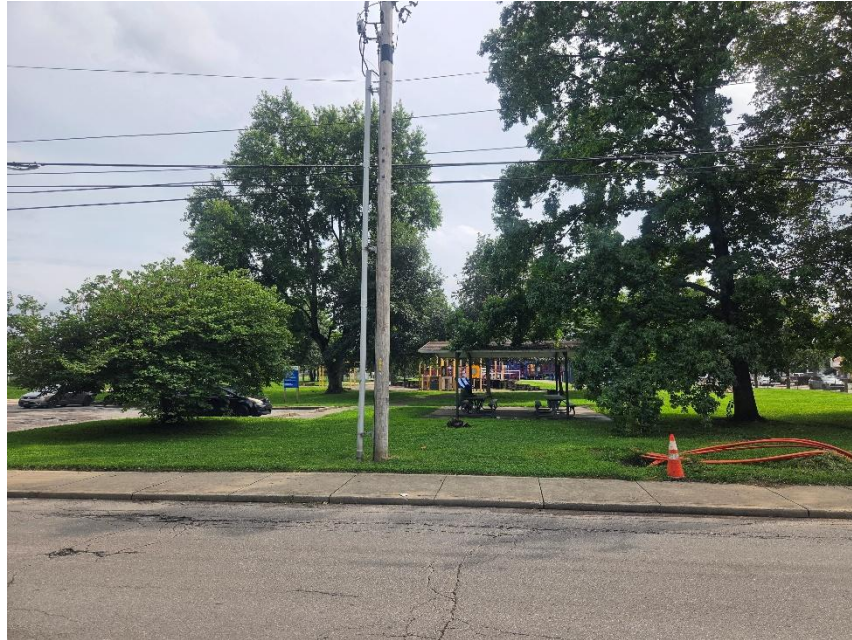
Photo 1: Existing Shelter Viewed from North
