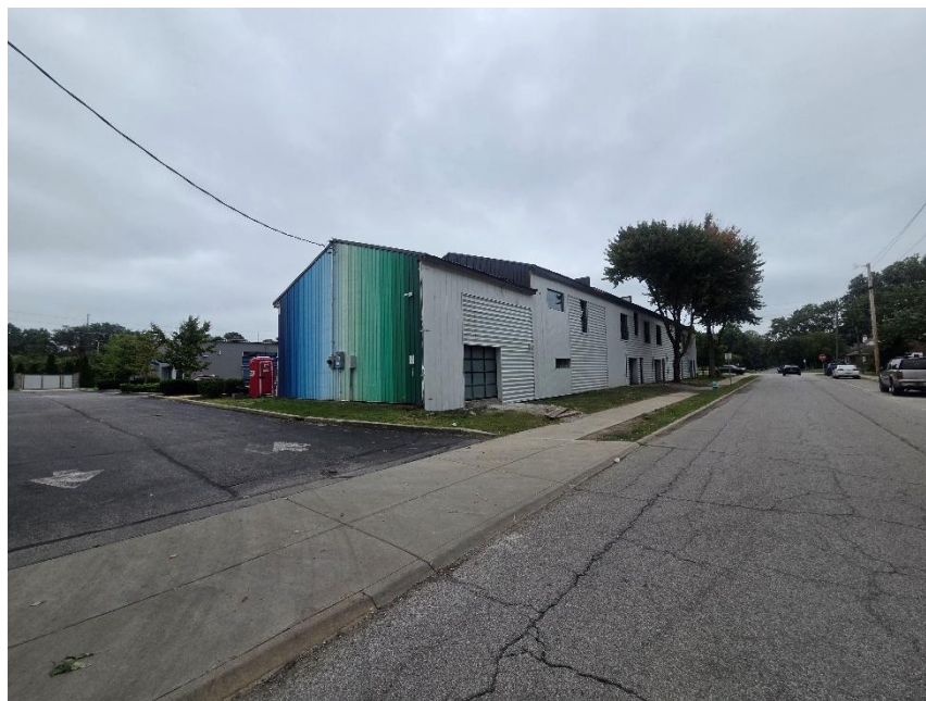
Photo 4: Western Building Viewed from Northwest
