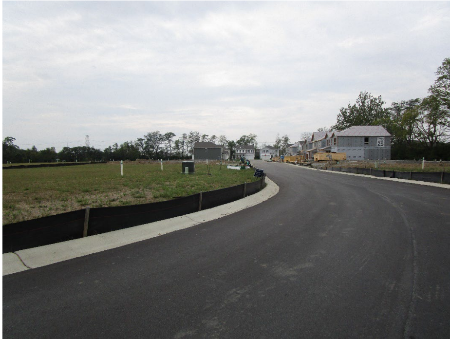
View looking west along Everland Place
