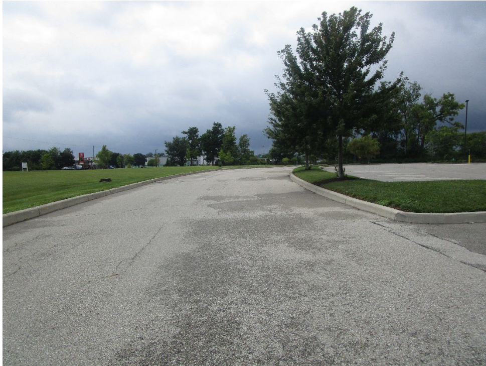
View looking west along Northview Way
