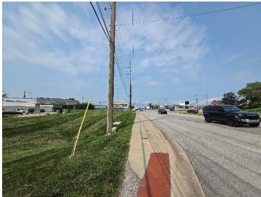
Photo 10: Allisonville Road Existing Sidewalk from South
