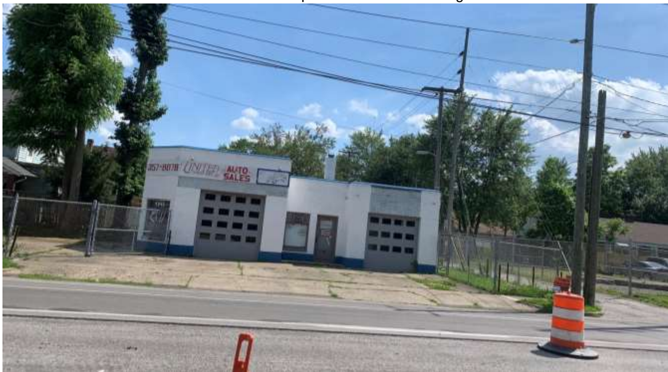
Photo of the western portion of the site looking south.
