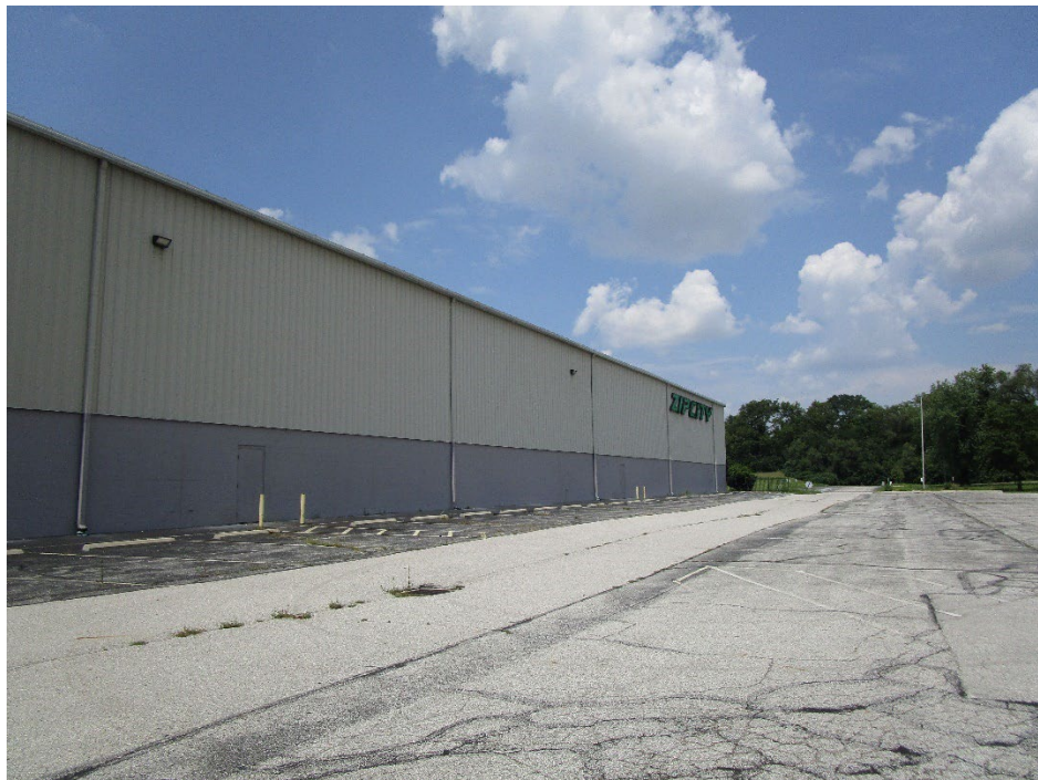
View of site looking north
