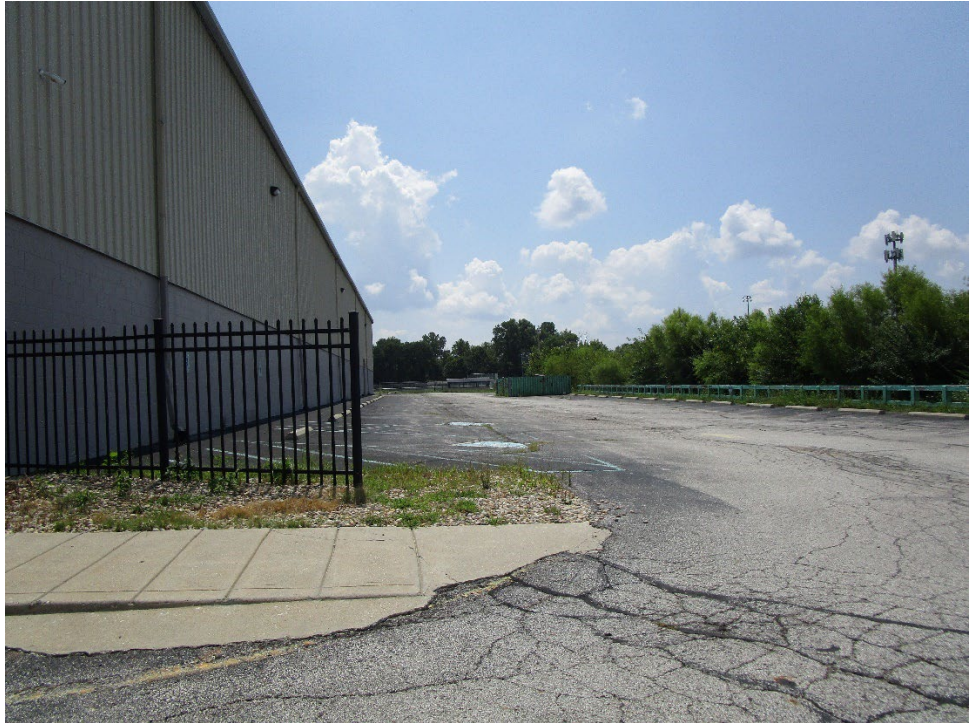
View of site looking south
