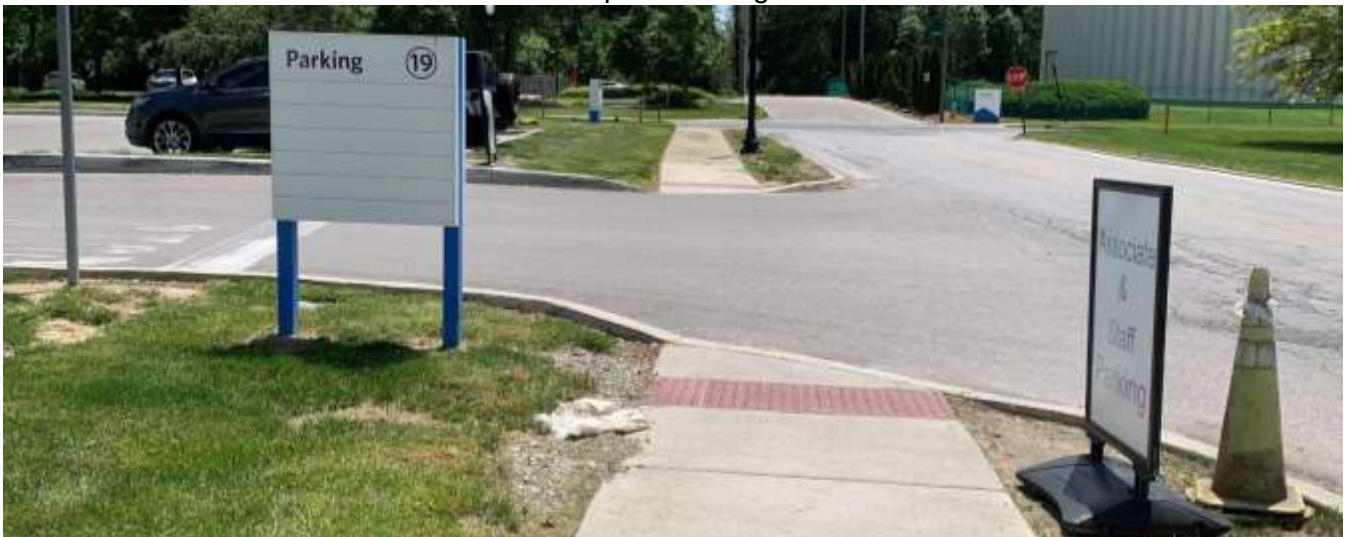
WF24 to be replaced along Naab Road.
