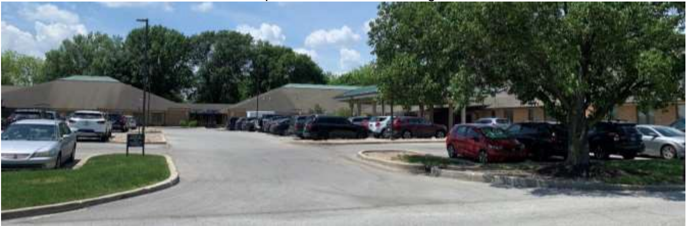
E18 to be replaced along Naab Road.
