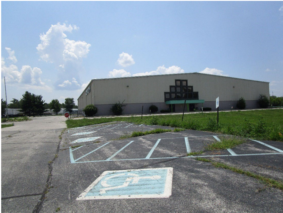
View of site looking south
