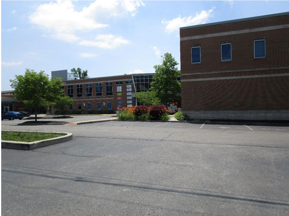
View from site looking southeast
