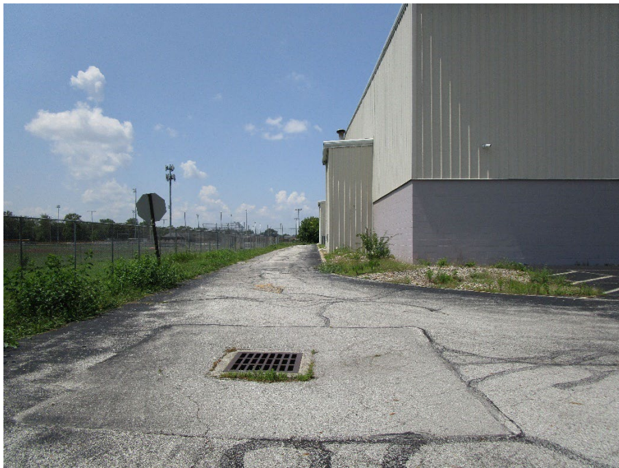
View of site looking west along southern boundary
