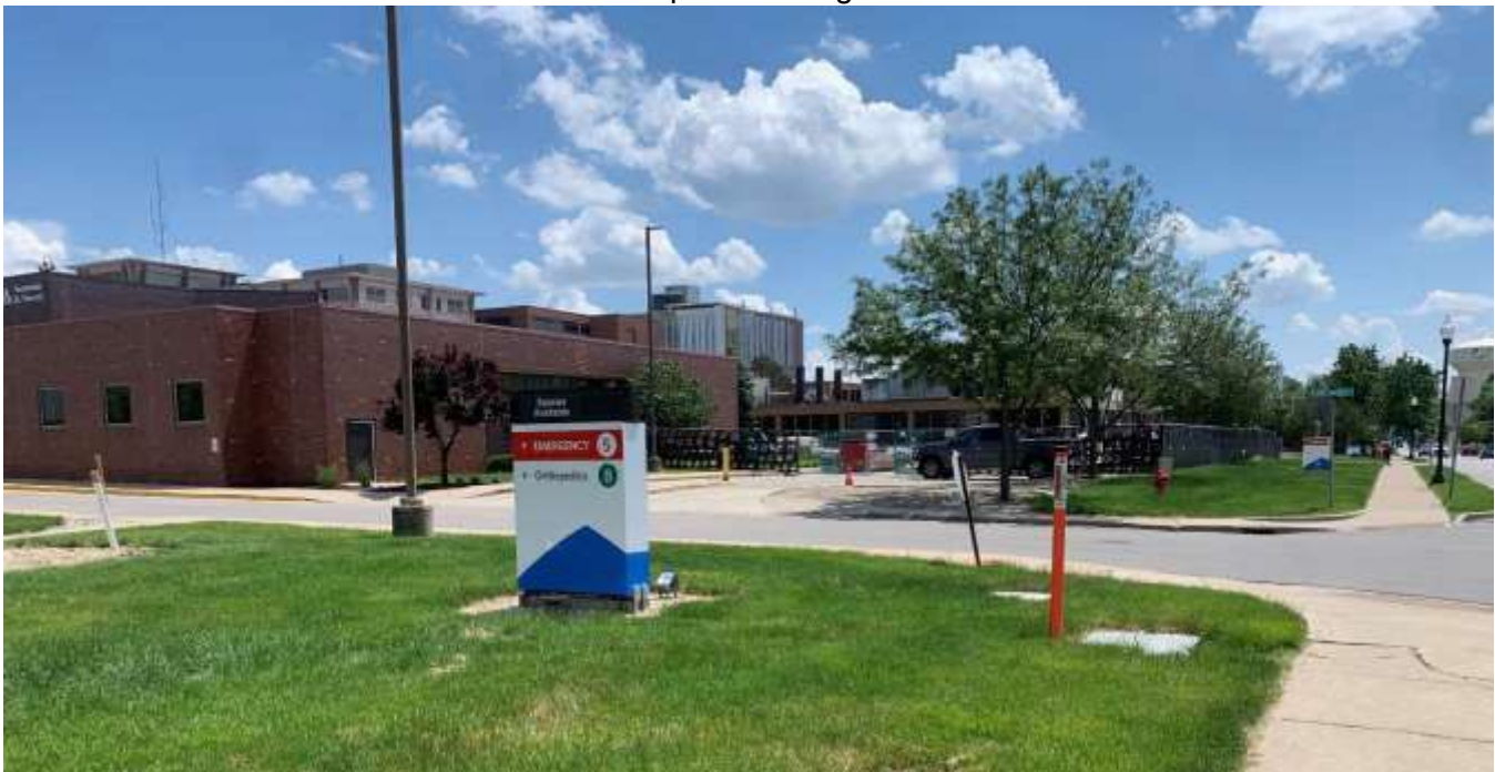
E14 to be replaced along Naab Road.
