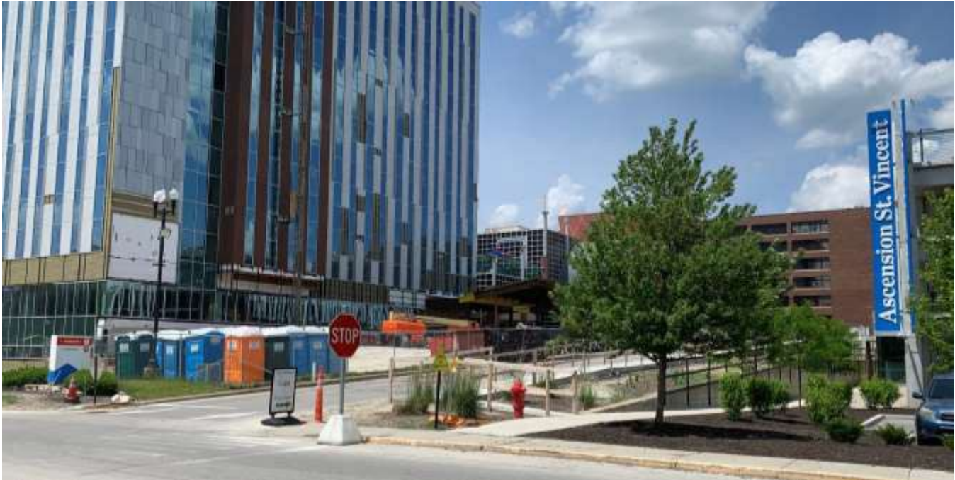
WF07 new sign to be installed along Kate Knox Drive.
