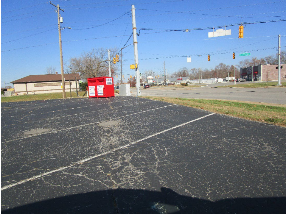
View looking north along north Keystone Avenue
