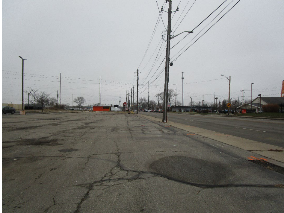
View looking south along North Sherman Drive
