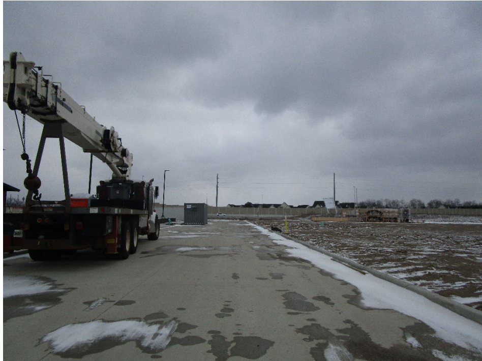
View looking east along Southport Commons Drive
