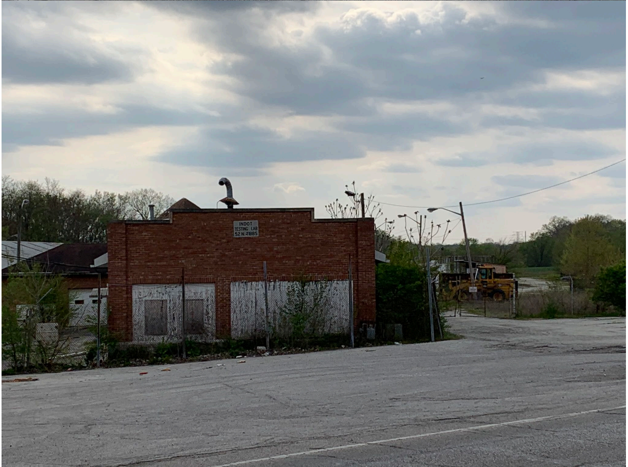
Views of existing buildings on the subject site
