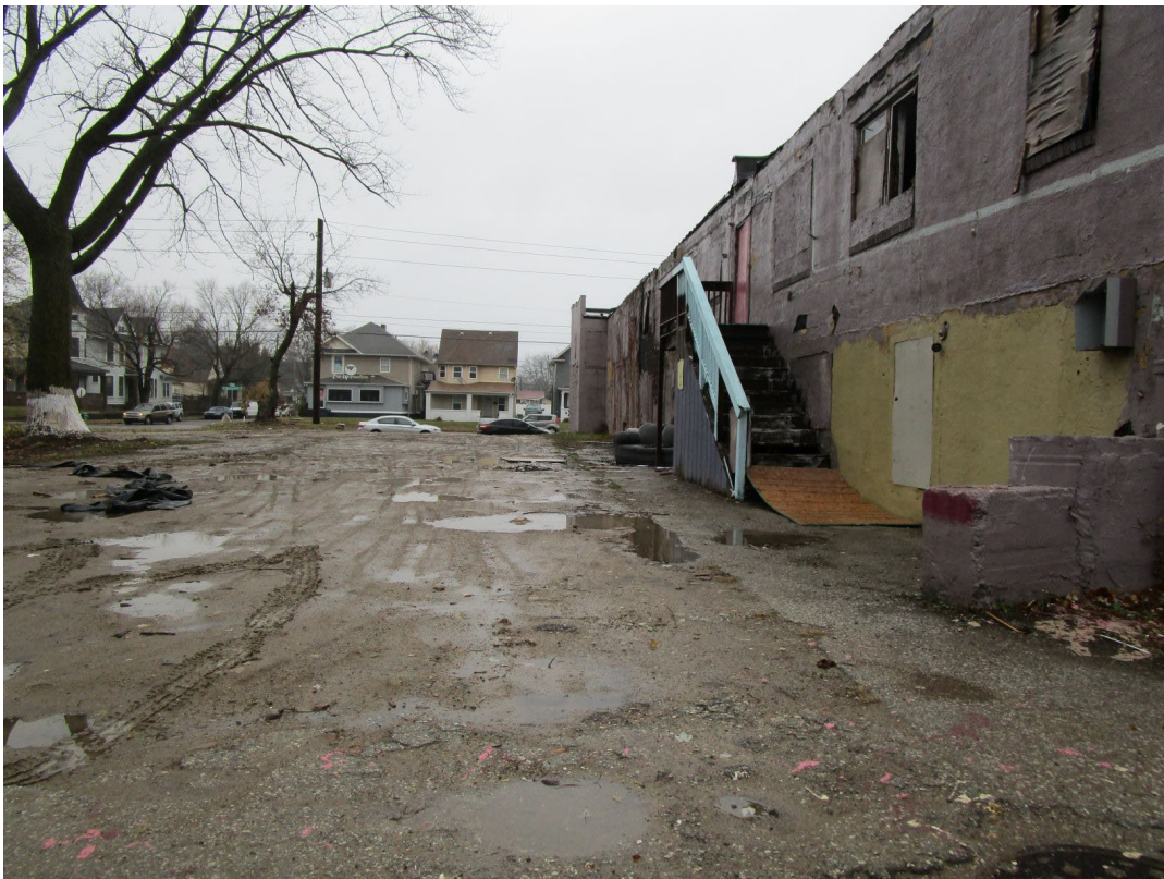
View of site looking north
