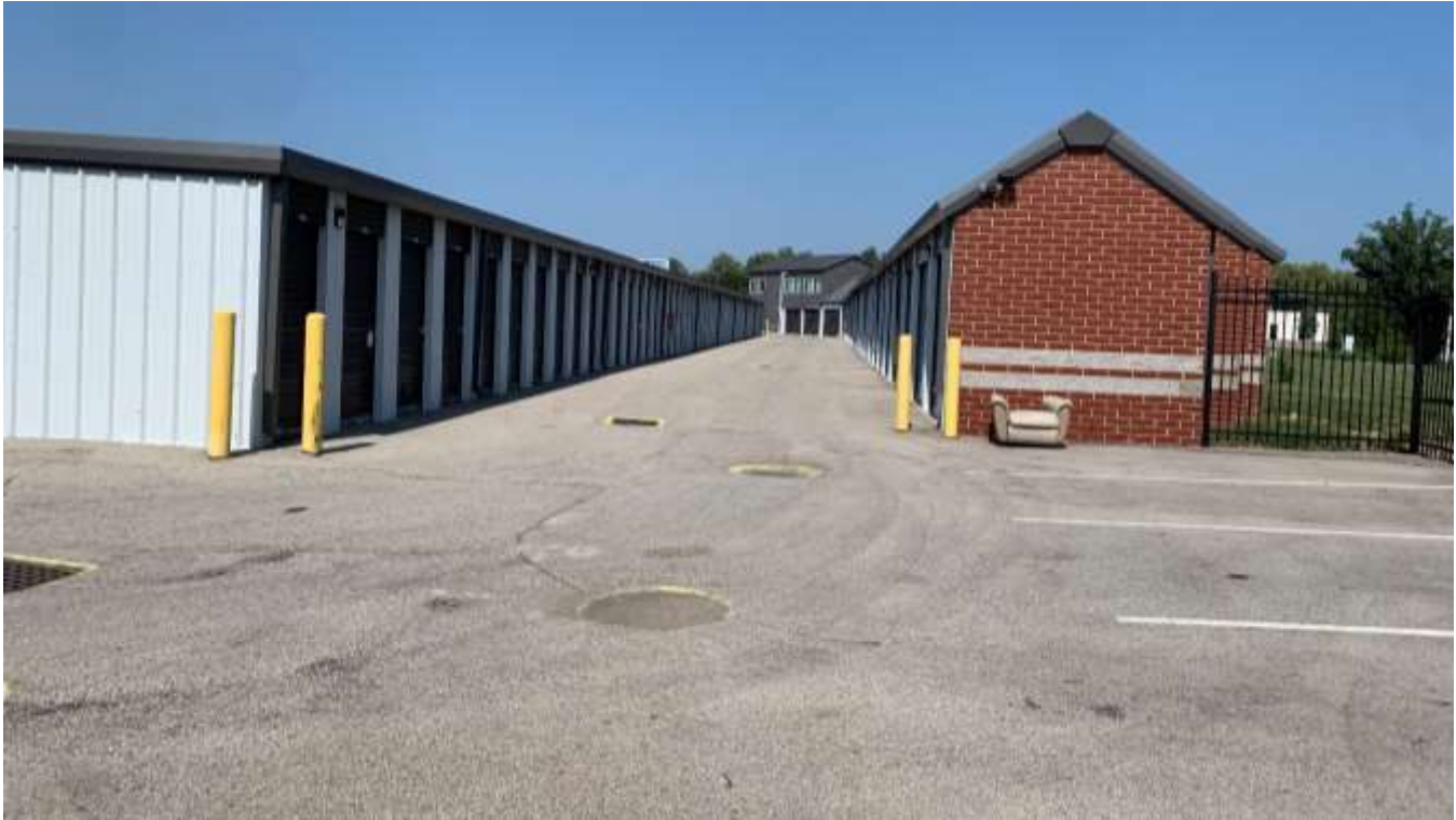
Photo of the storage facility looking northeast.
