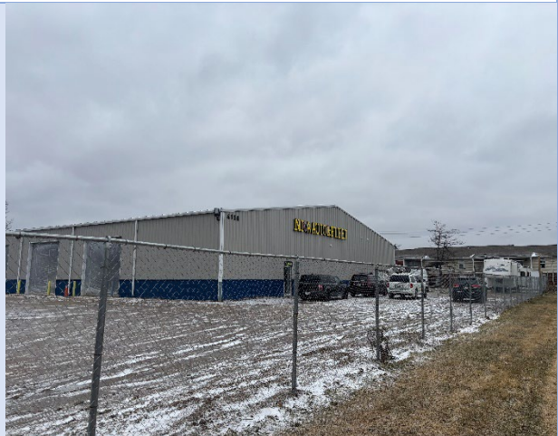
Looking form private drive to subject site
