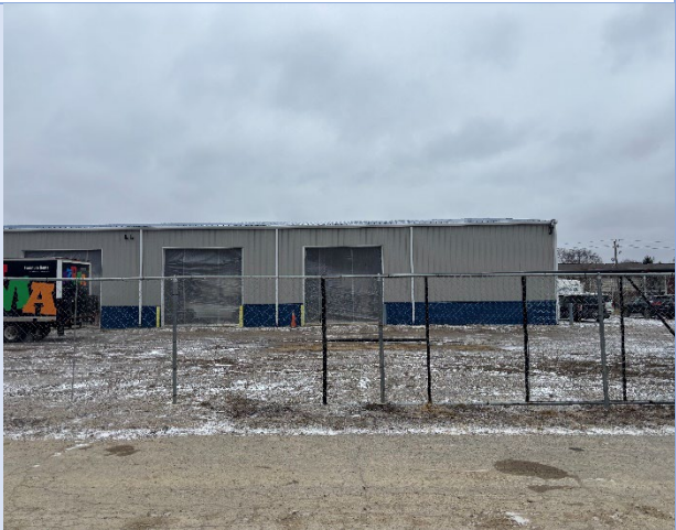
Looking form private drive to subject site
