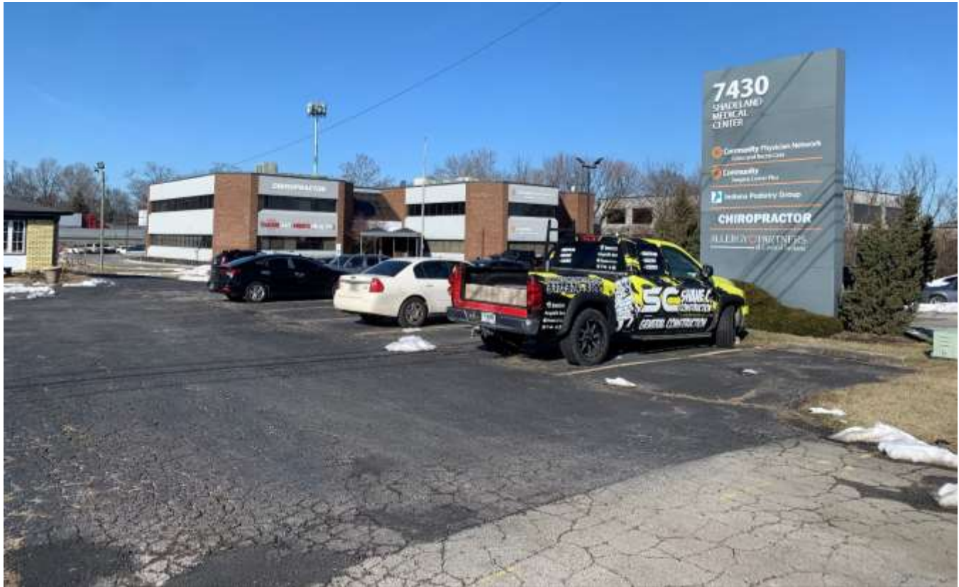
Photo of the front parking area and offices north of the site.
