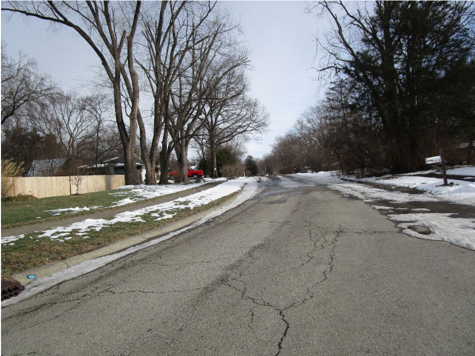
View looking east along East 88 th Street
