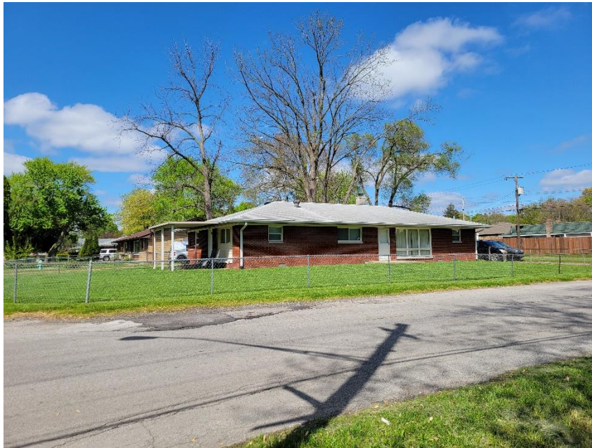
Photo 6: Adjacent Property to the Northeast
