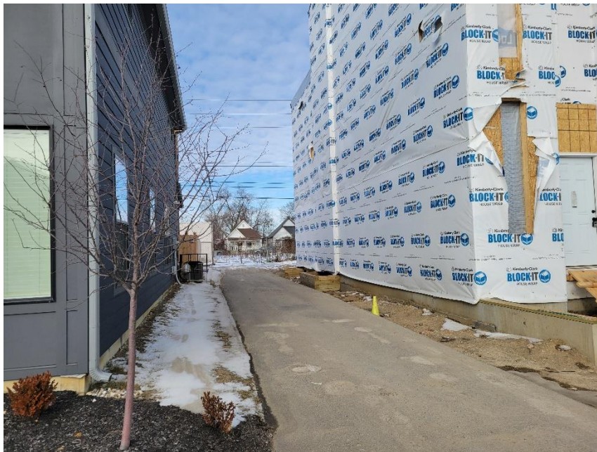
Photo 2: Existing Side Alley Viewed from South
