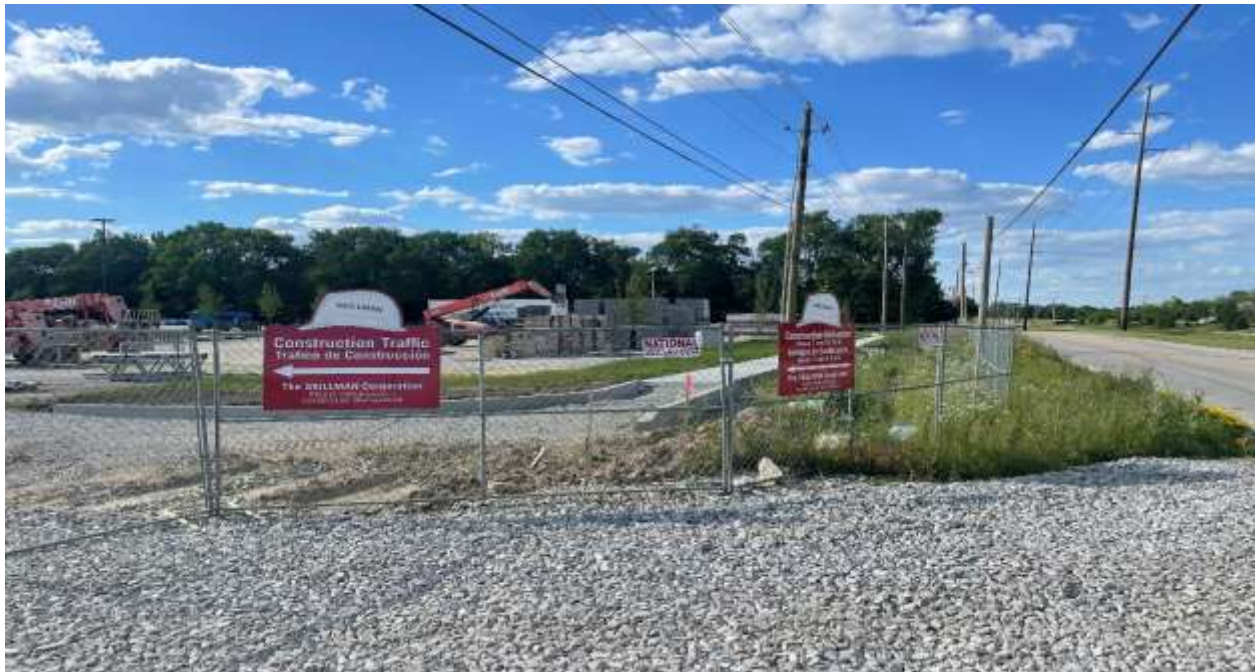
Photo Two: Looking North along Senour Road
