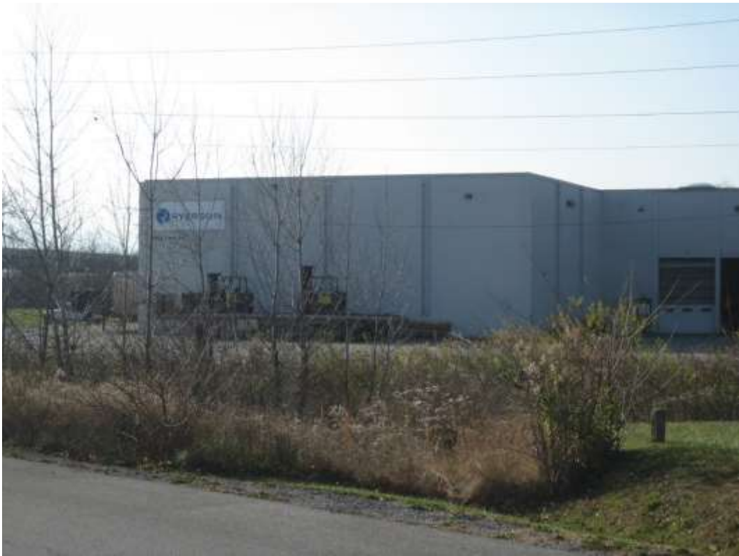
Adjacent manufacturing facility to the west of the site.
