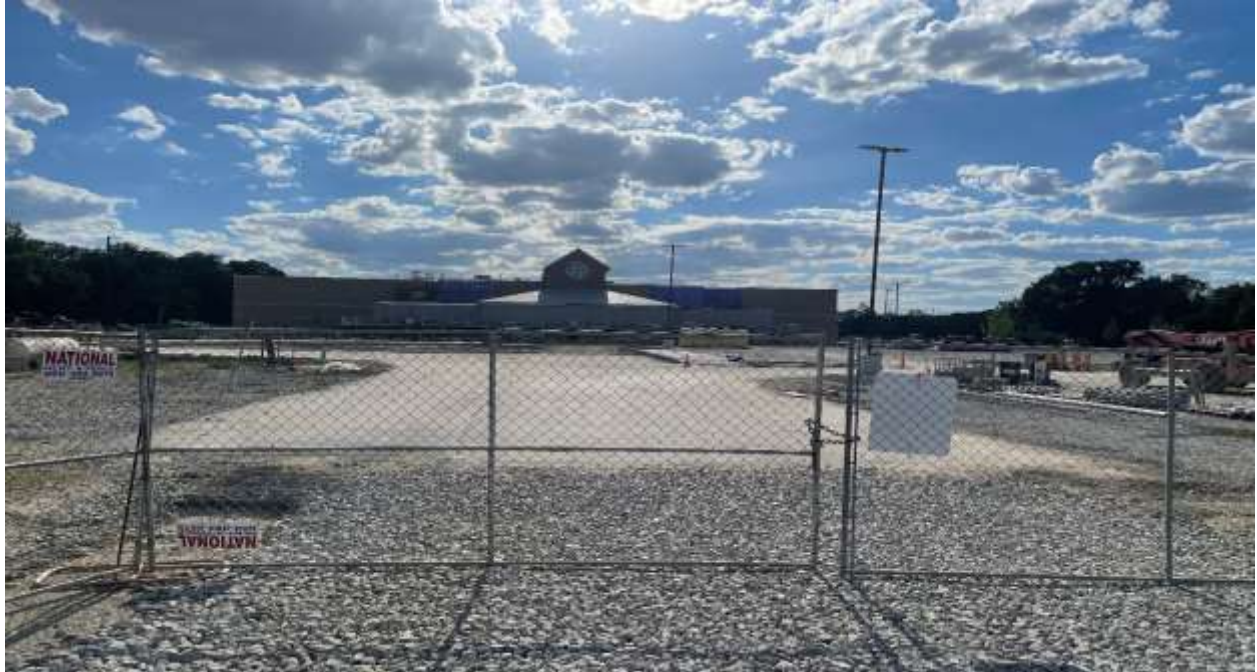
Photo One: Building under construction on subject site, facing West
