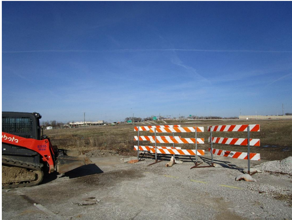
View of site looking northeast
