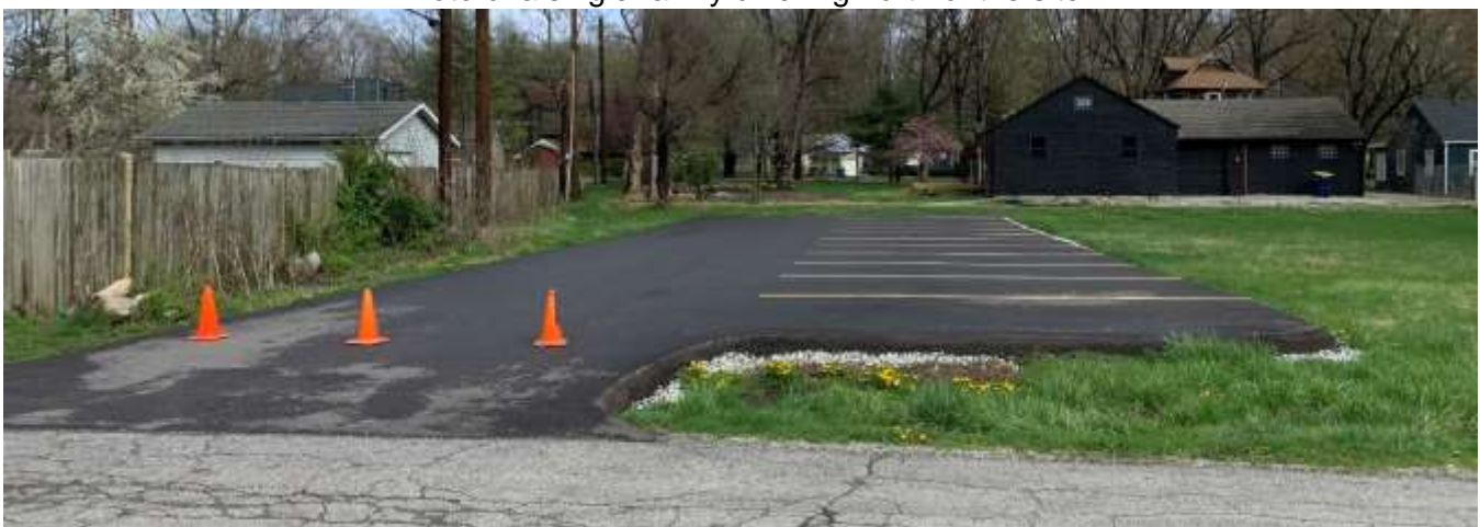
Photo of a parking lot at 7429 Westfield Boulevard that received a zoning violation.
