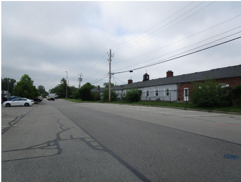
View looking southwest along access drive along eastern boundary
