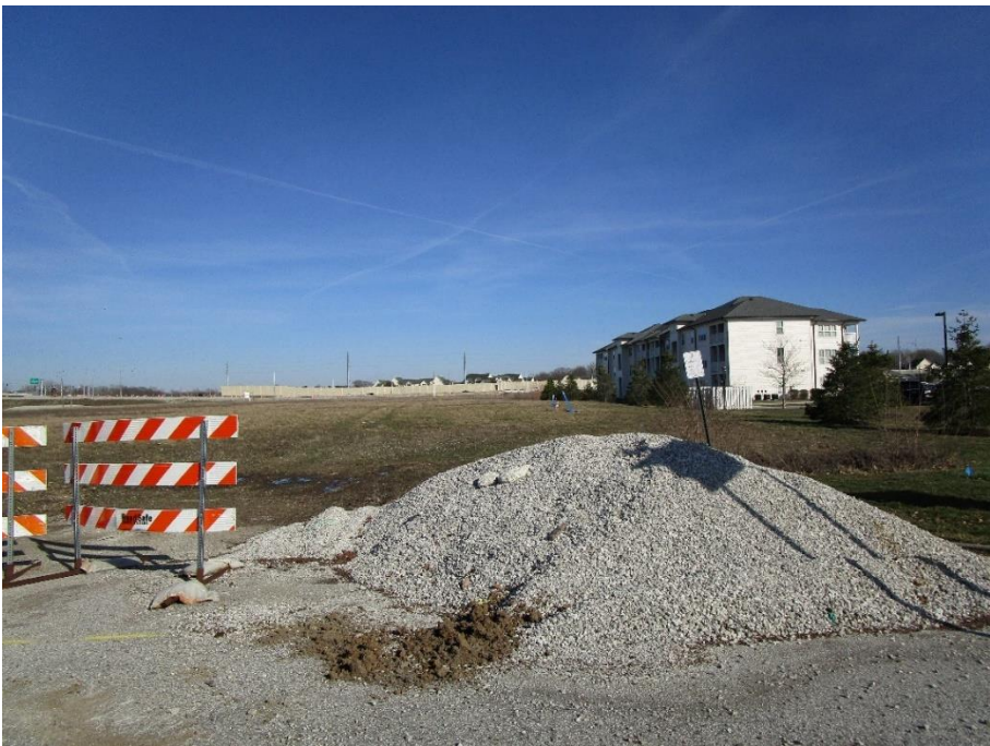
View of site looking east
