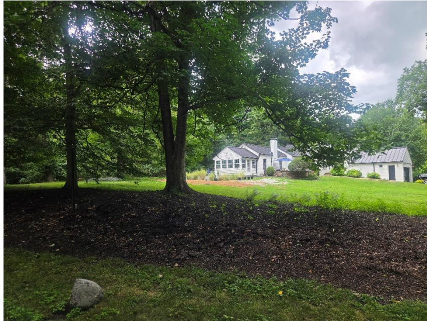
Photo 3: Subject Site Viewed from Northwest
