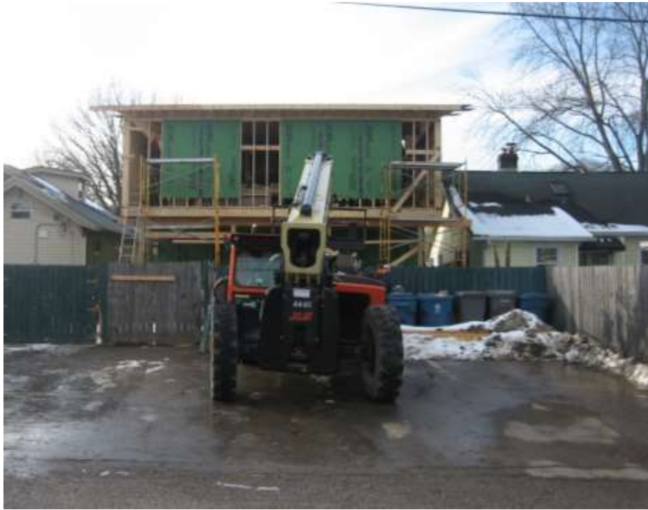
Subject site rear, looking west from adjacent rear alley.
