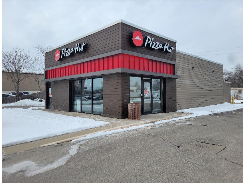
Photo 1: Subject Building Viewed from Southeast
