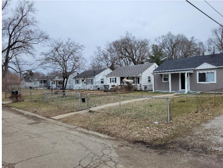
Photo 5: Adjacent Property to East of Subject Site
