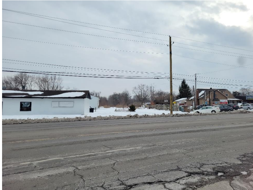
Photo 7: Adjacent Property to South
