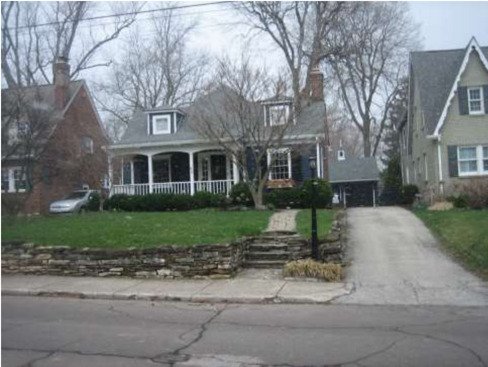
Adjancet dwellign to the west, looking north.
