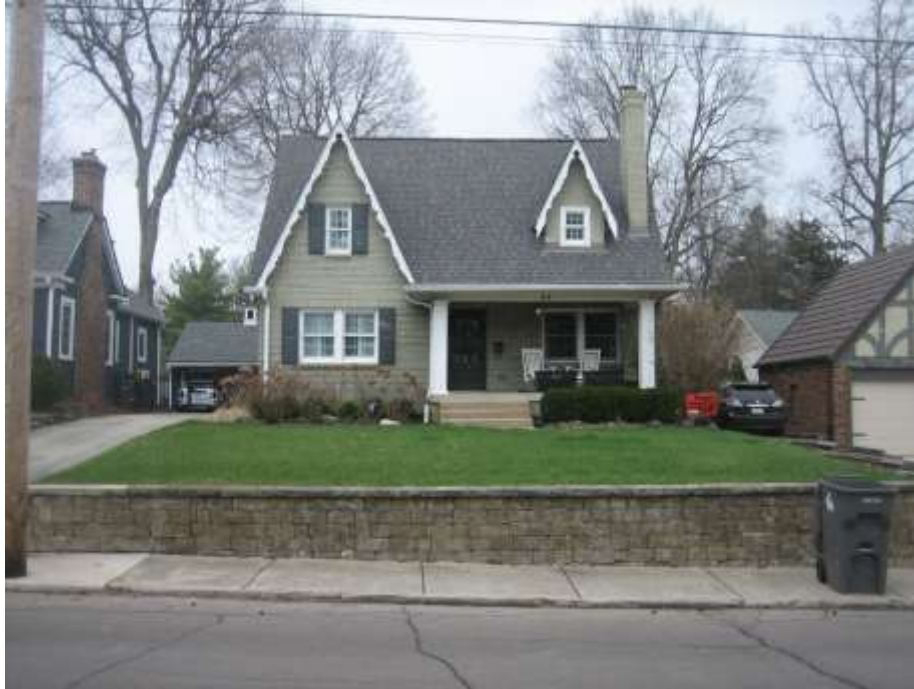
Subject site, existing dwelling, looking north.
