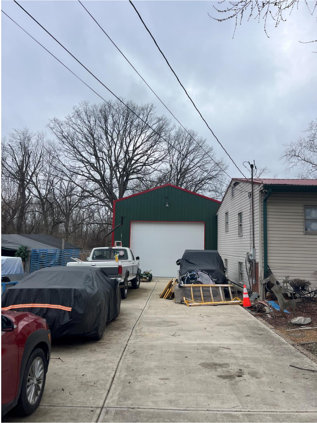
Photo 2: Subject property barn (taller than primary dwelling)
