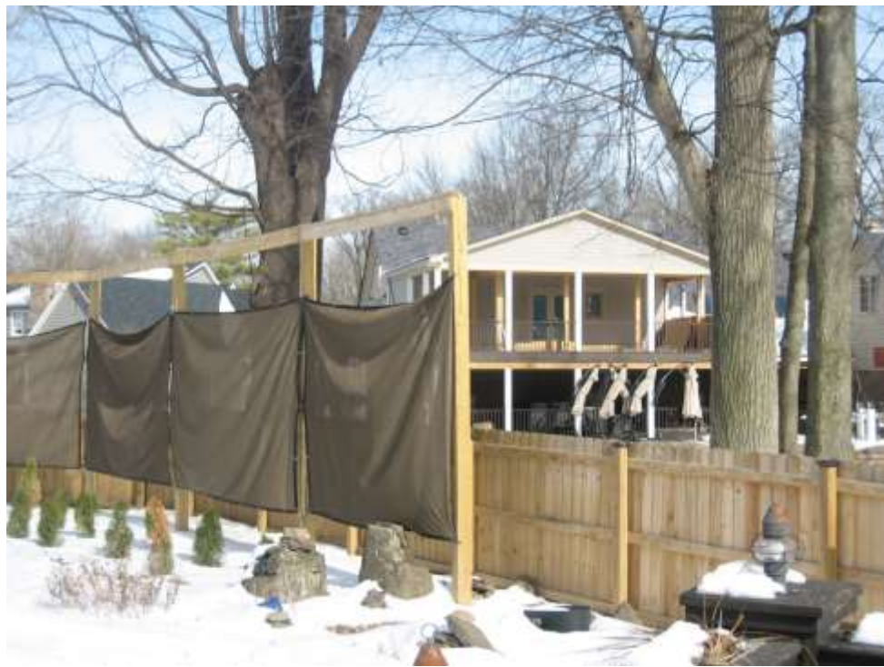
Subject property proposed fence looking north.
