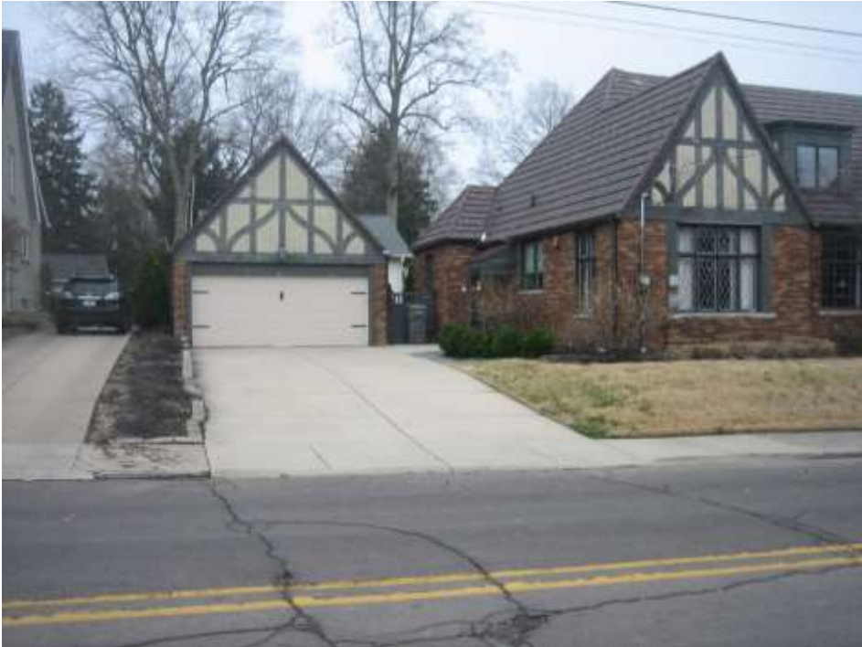
Adjacent dwelling to the east, with similar garage setback, looking north.
