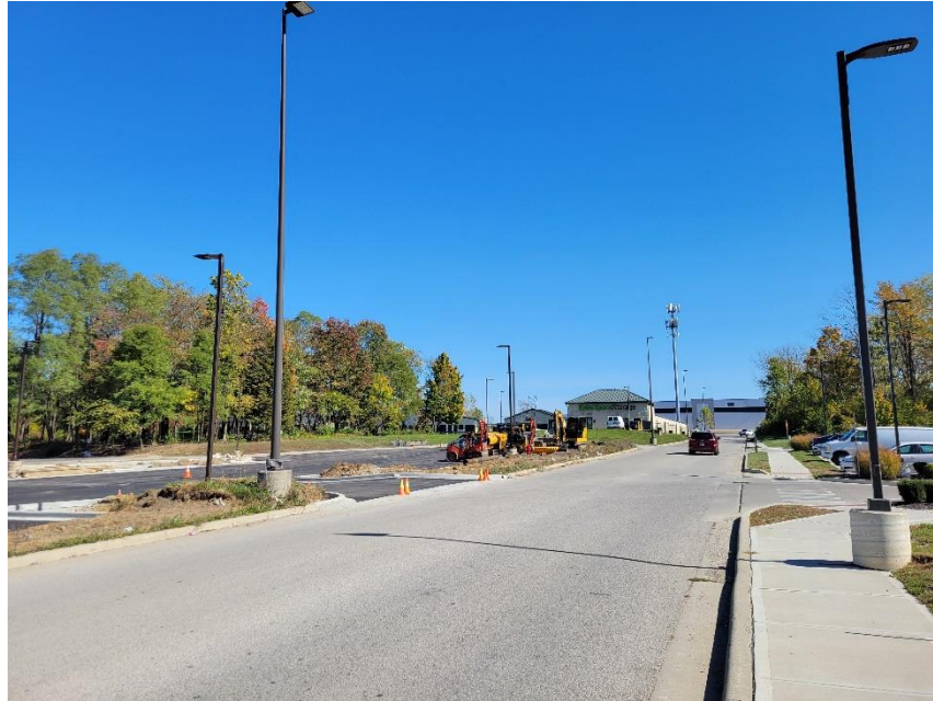
Photo 7: Adjacent Property to East
