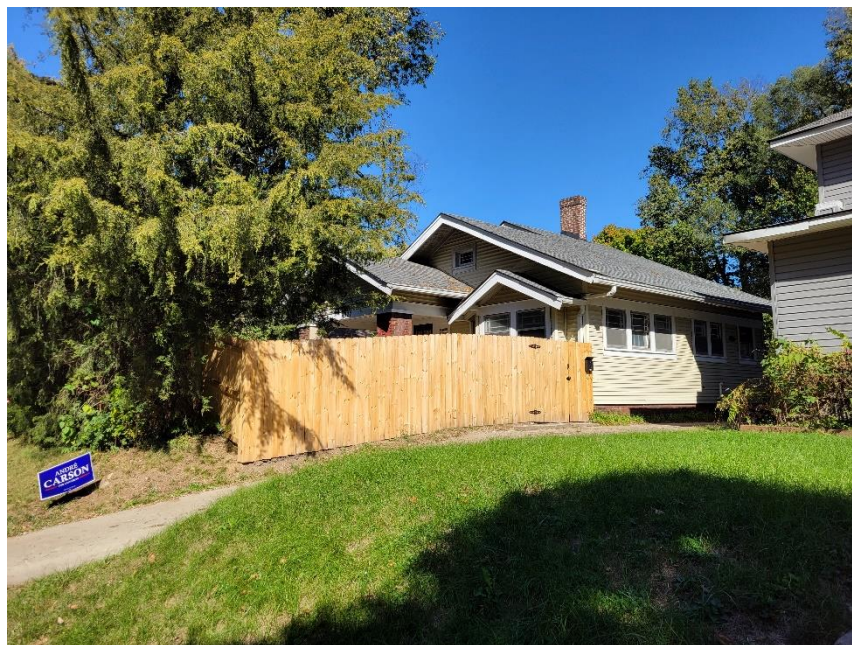
Photo 4: Subject Site Viewed from Southwest
