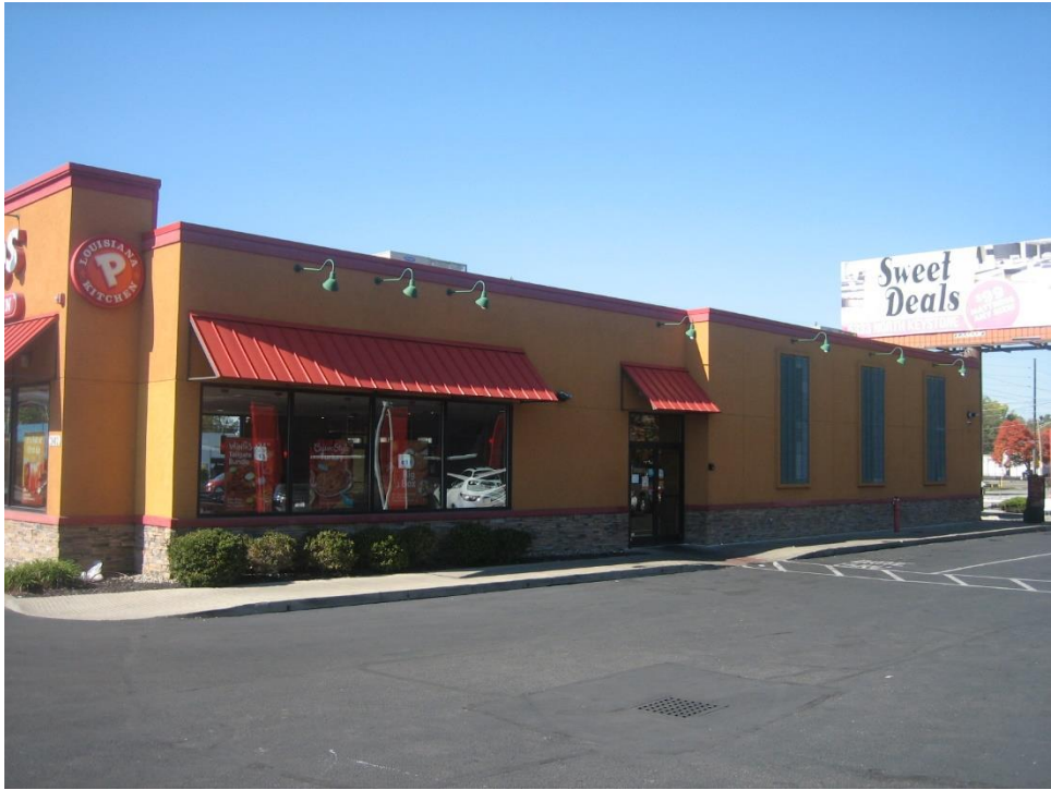
Subject site, east façade, looking northwest.
