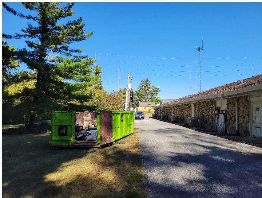
Photo 6: Rear of Building (multiple tenant bays)
