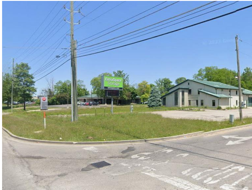
Photo 3: Subject Site from Southwest (May 2023)
