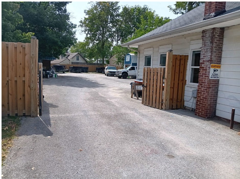
Exhibit 9: Work area behind 9111 Crawfordsville.
