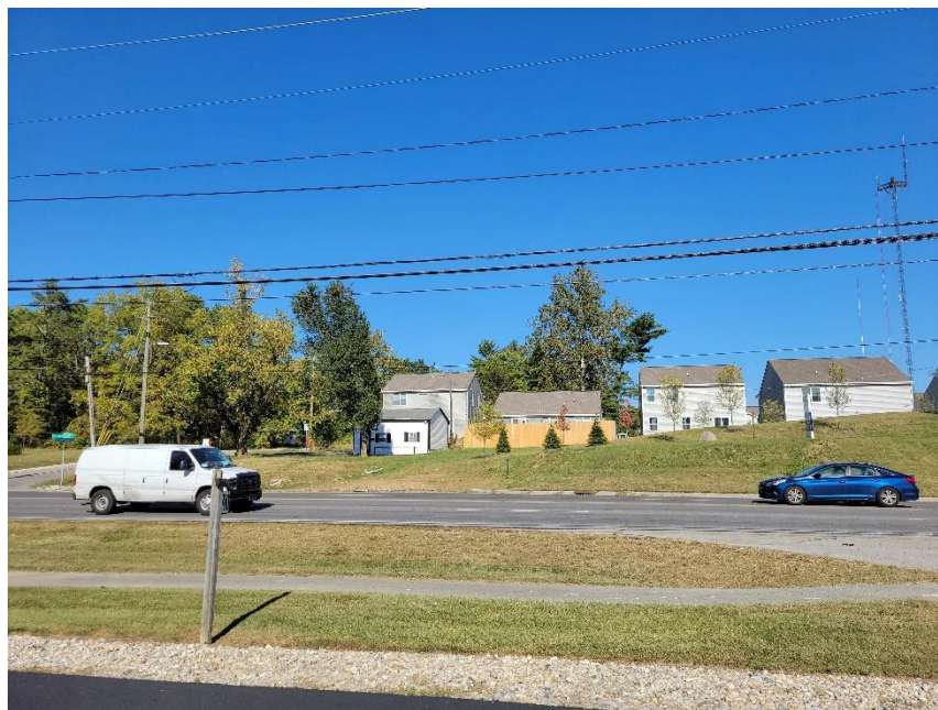
Photo 4: Adjacent Property to East
