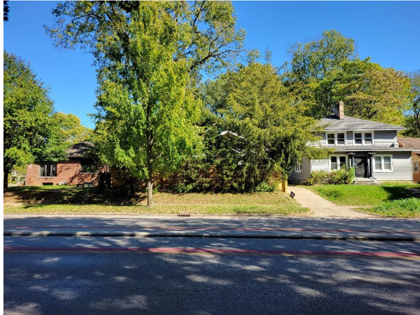
Photo 1: Subject Site Viewed from West (further sidewalk)
