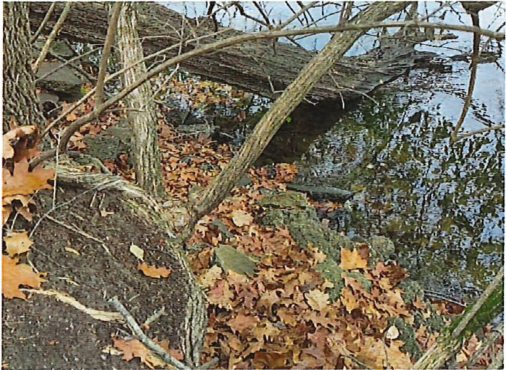
8. Stone at toe of bank on adjacent White River.
