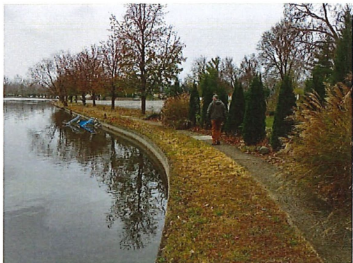
2. Concrete seawall along Event Center is stable.
