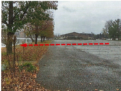
4. Event Center parking lot stormwater runoff into lake.
