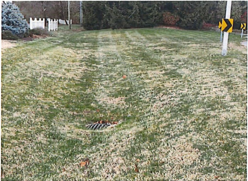
6. Roadside drain inlet draining to White River.
