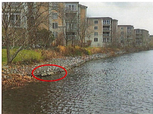
1. Riprap extends along entire shoreline at Condominiums.
