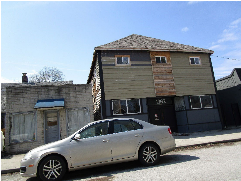
View of site looking west across North Olney Street
