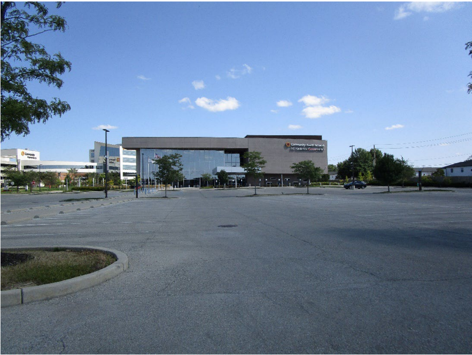
View of site looking north
