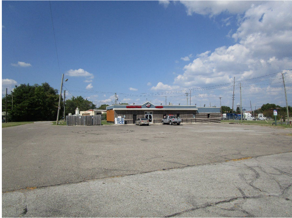
View of site looking north
