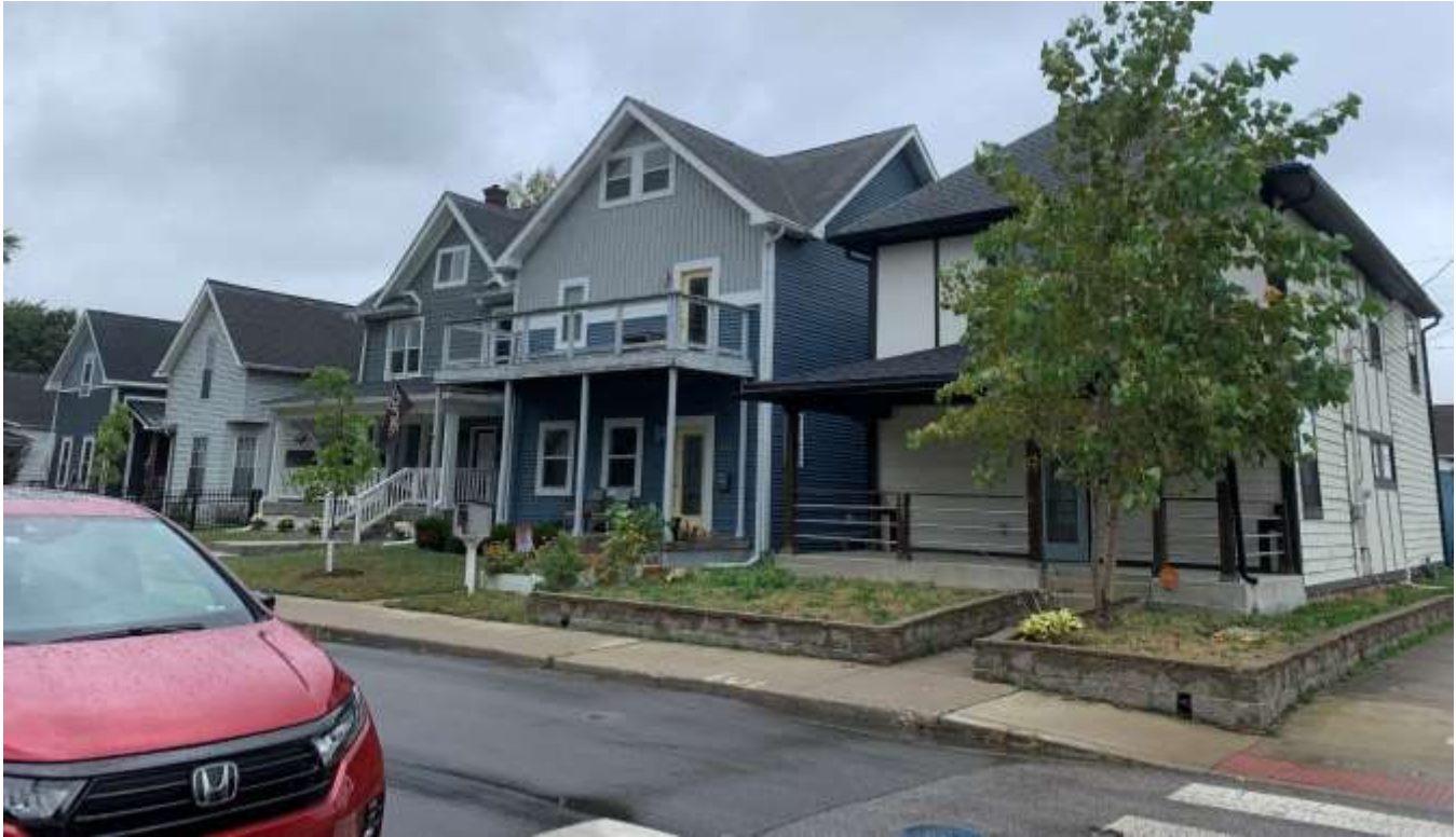
Photo of the single-family dwellings north of the site.
