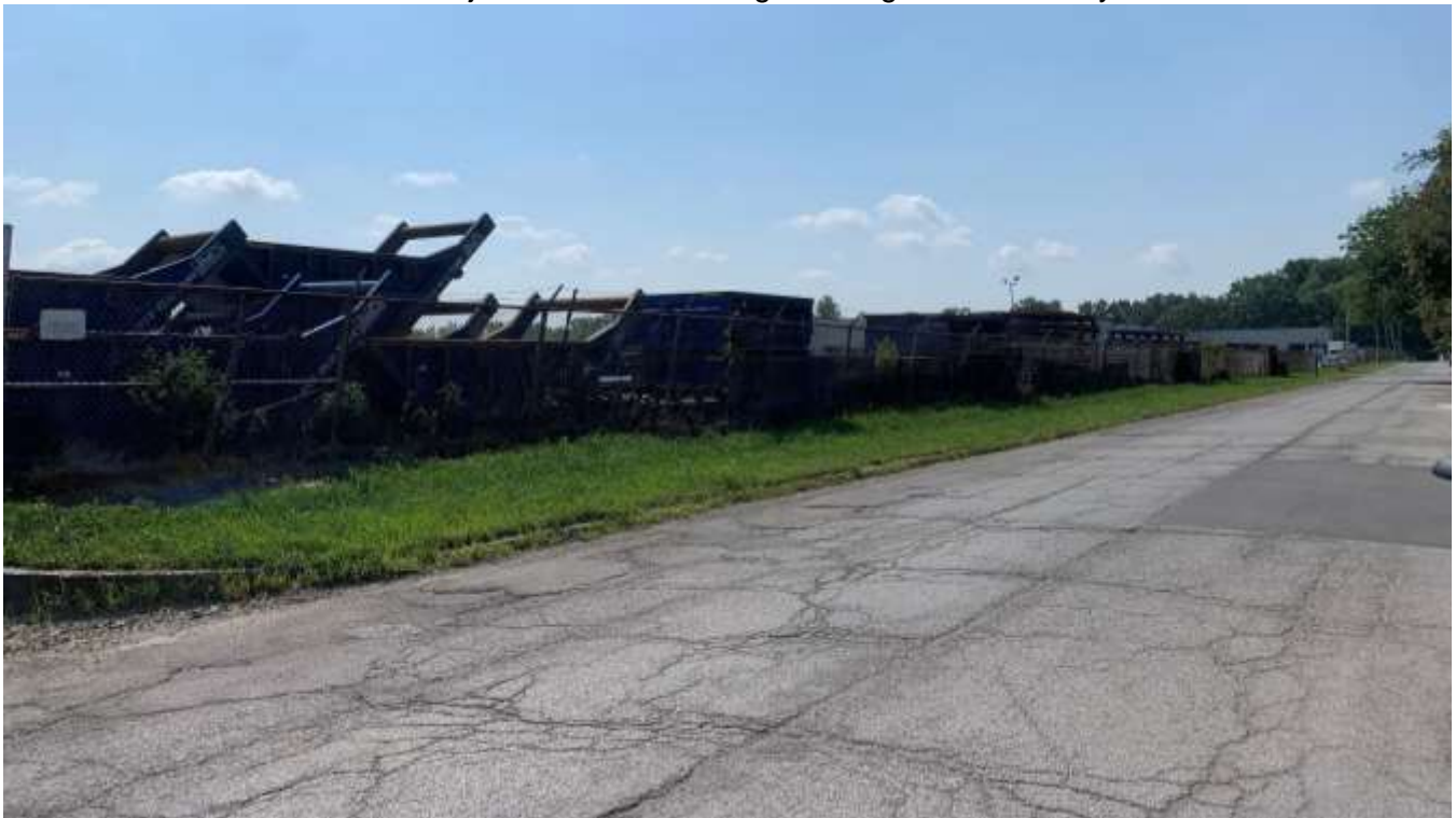
Photo of the subject site street frontage looing south on Olney Street from the closed driveway on site.
