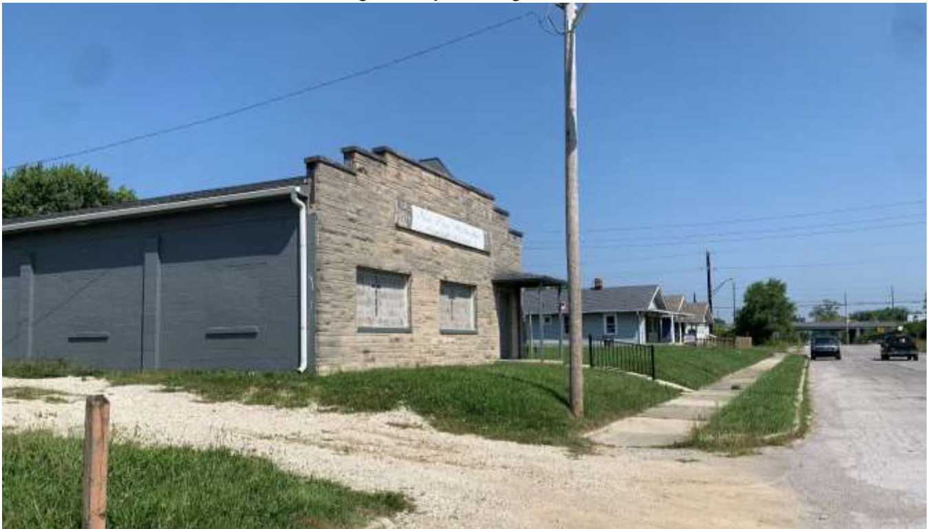
Photo of a church west of the site.
