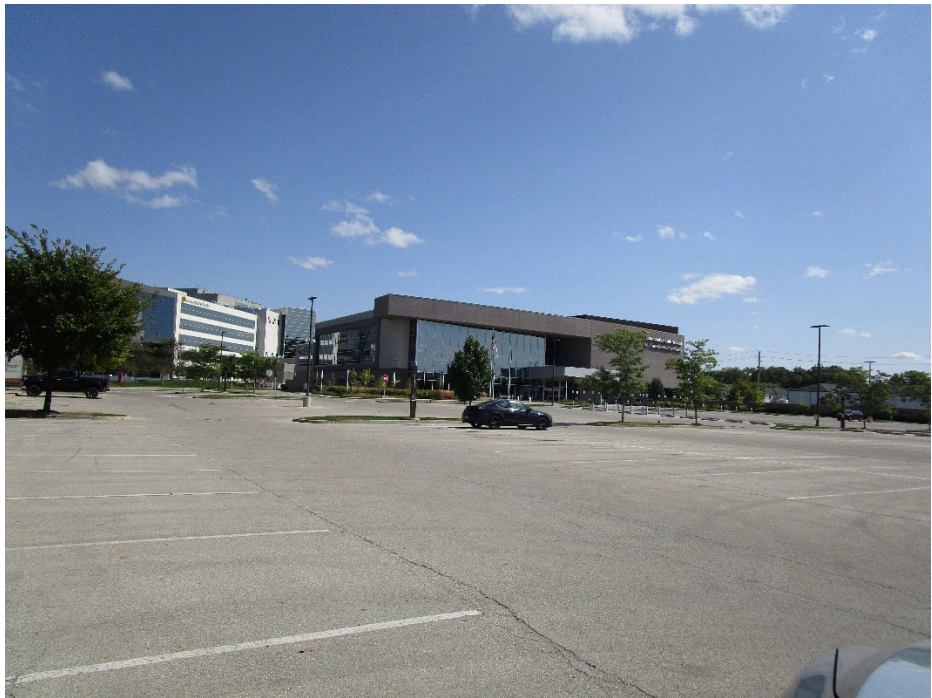
View of site looking southeast
