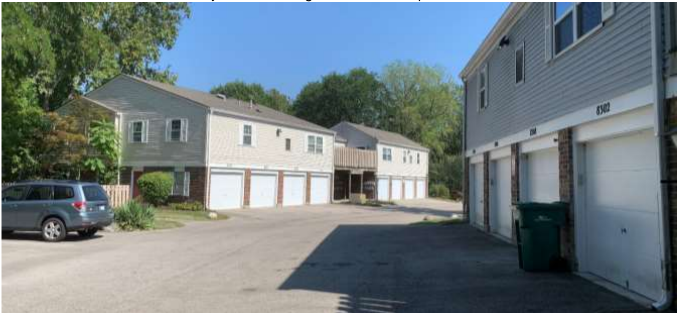
Photo of the quadrominiums southeast of the site looking southeast towards Woodall Drive.
