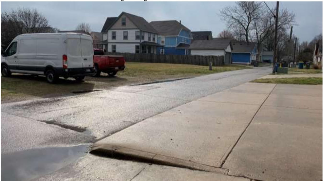
Photo of the alley west of 2460 North Delaware Street.
