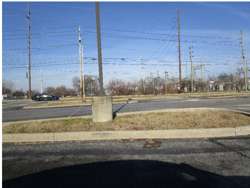
View from site looking north across West 10th Street
