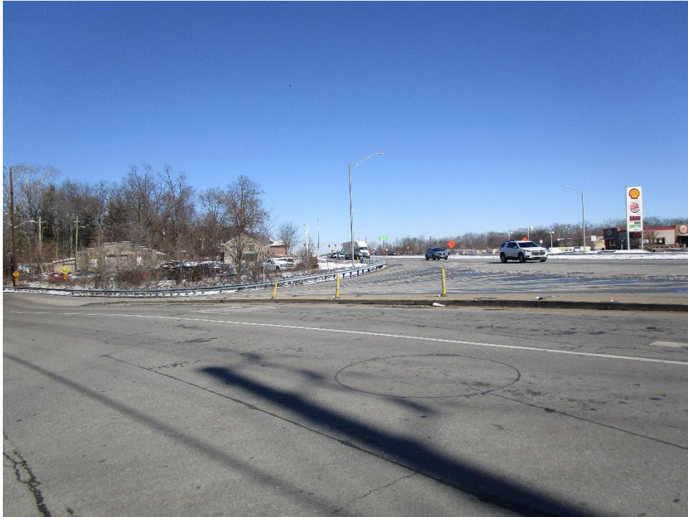
View looking north across intersection of South High School Road and Kentucky Avenue
