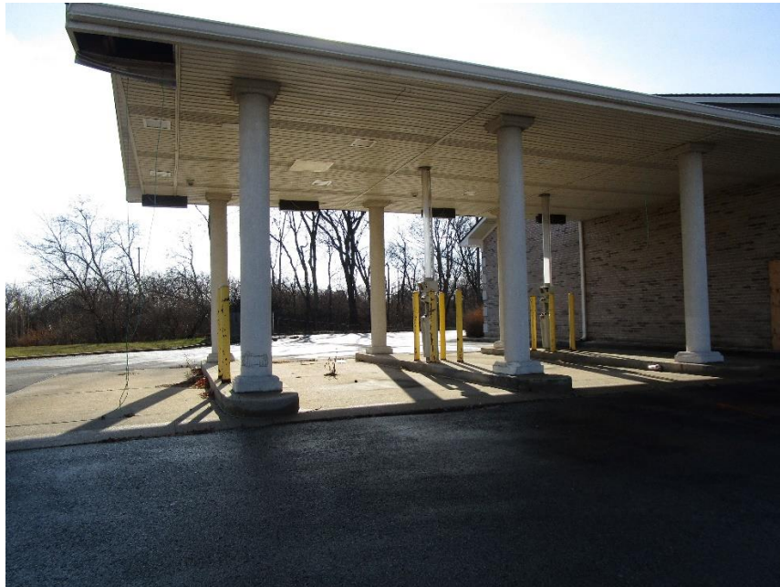
View of canopy to be removed looking south
