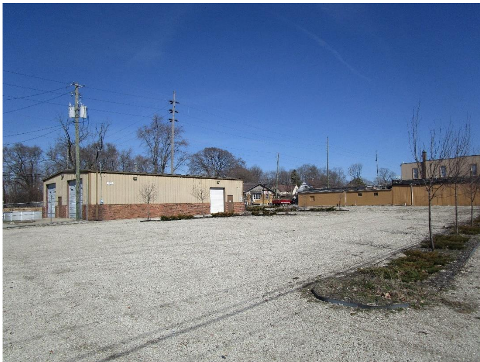
View of site looking northeast
