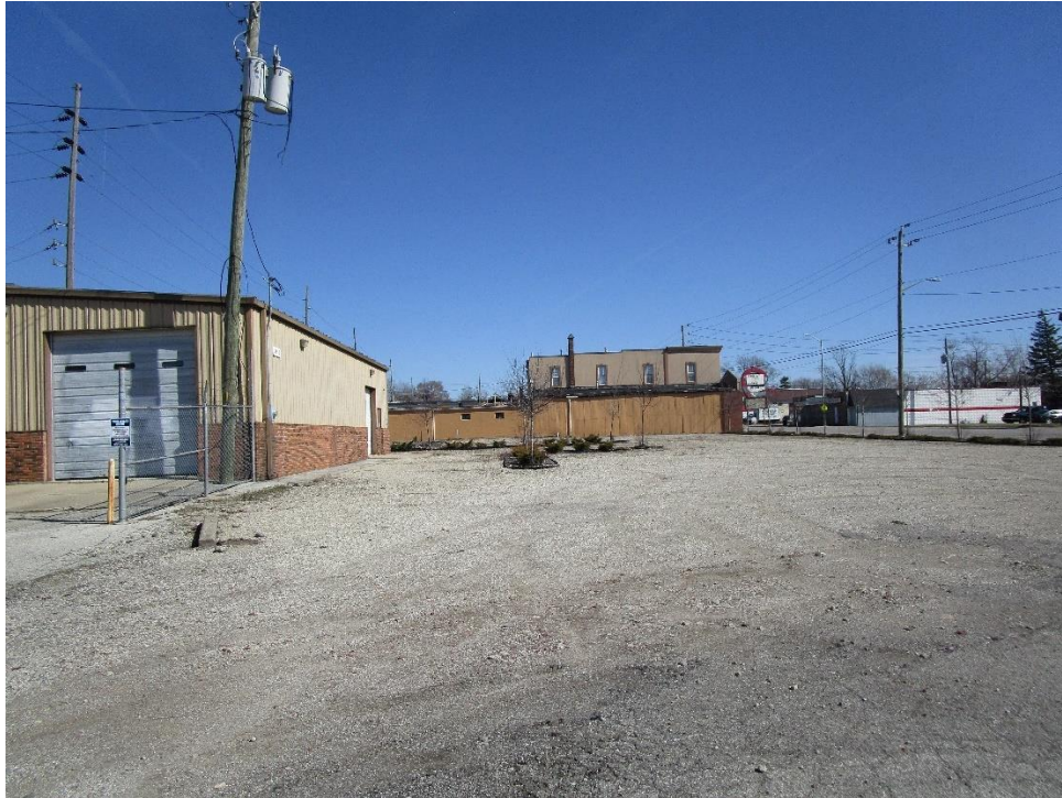
View of site looking east
