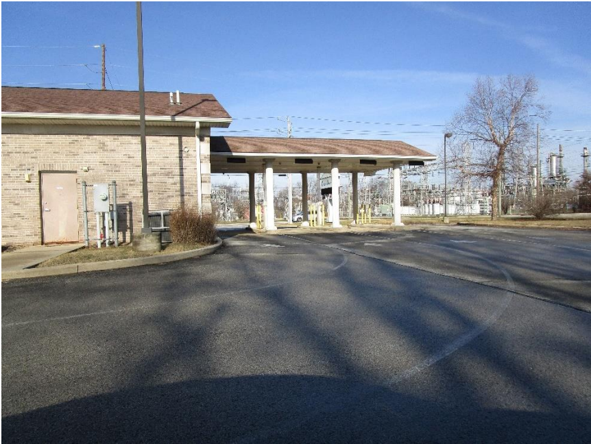
View of site looking northeast
