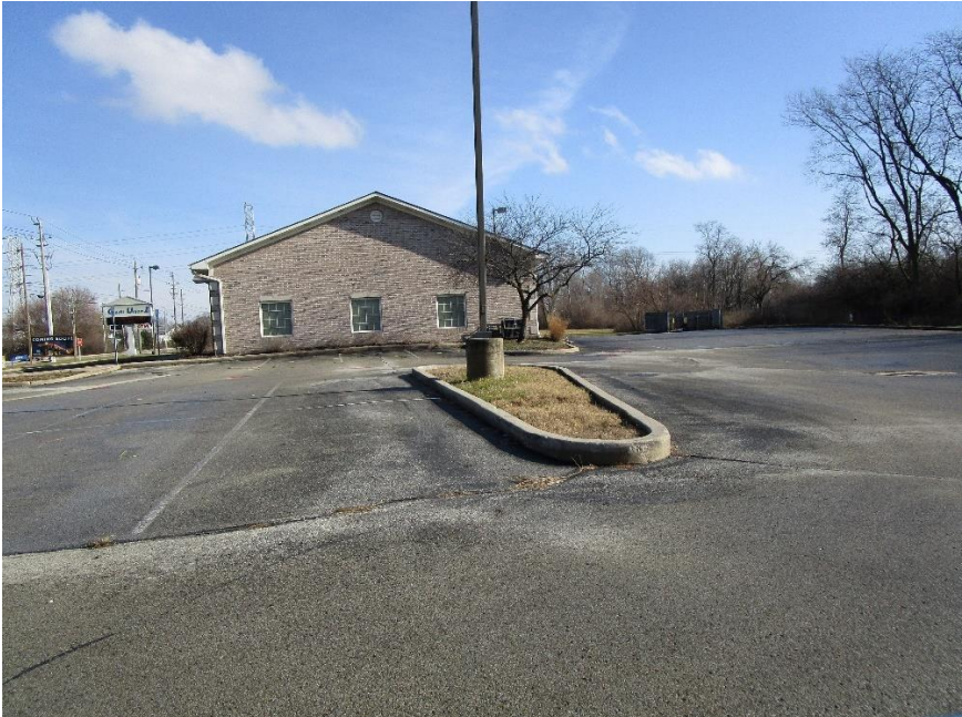
View of site looking east
