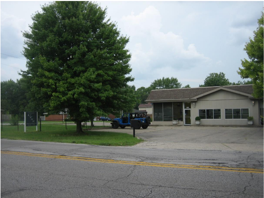
Photo of adjacent property to the south, looking west.
