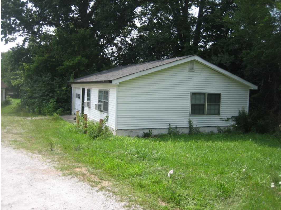
Photo of subejct site parcel two garage/auxiliary dwelling, looking west.
