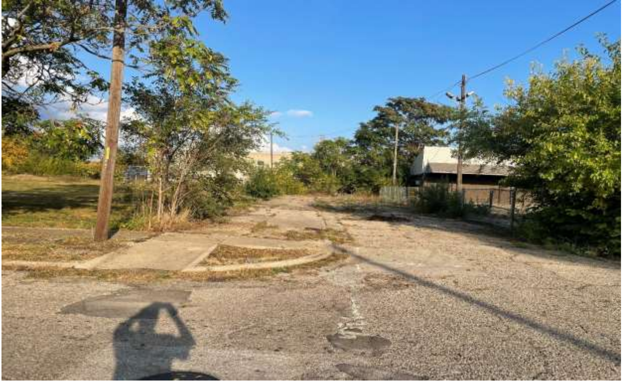
Photo One: East 24 th Street, Facing East
