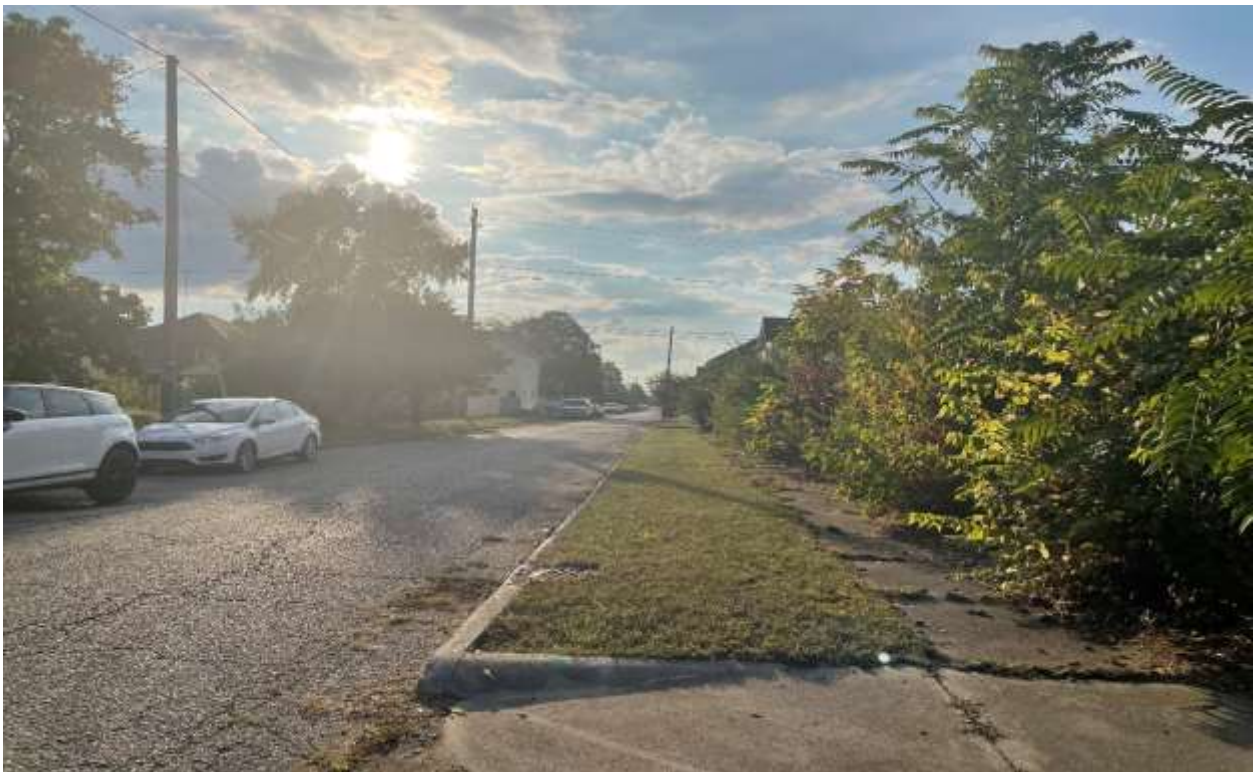
Photo Two: East 24 th Street, Facing West
