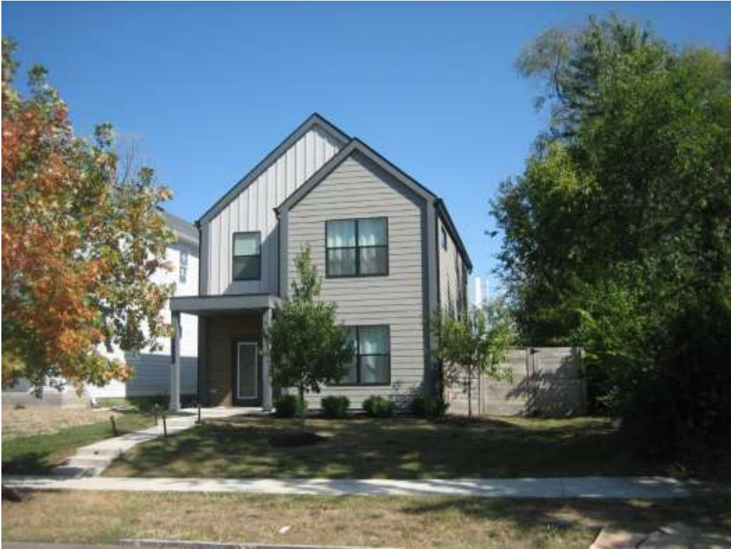
Single-Family Dwelling to the north of the site, looking east.
