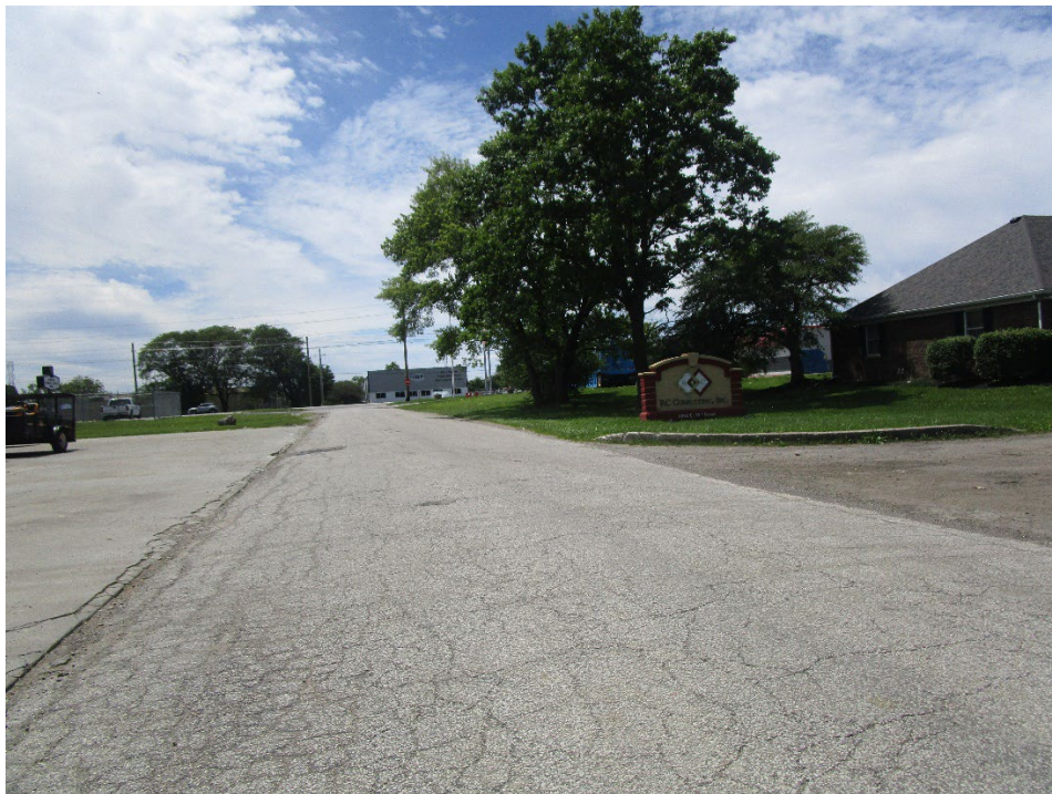
View looking west along East 33 rd Street
