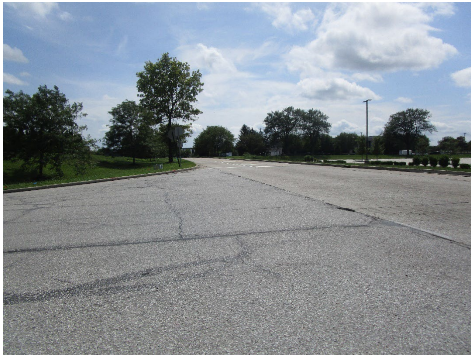
View looking south along Woodland Drive
