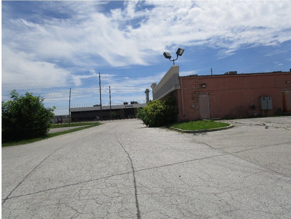
View looking south along access drive
