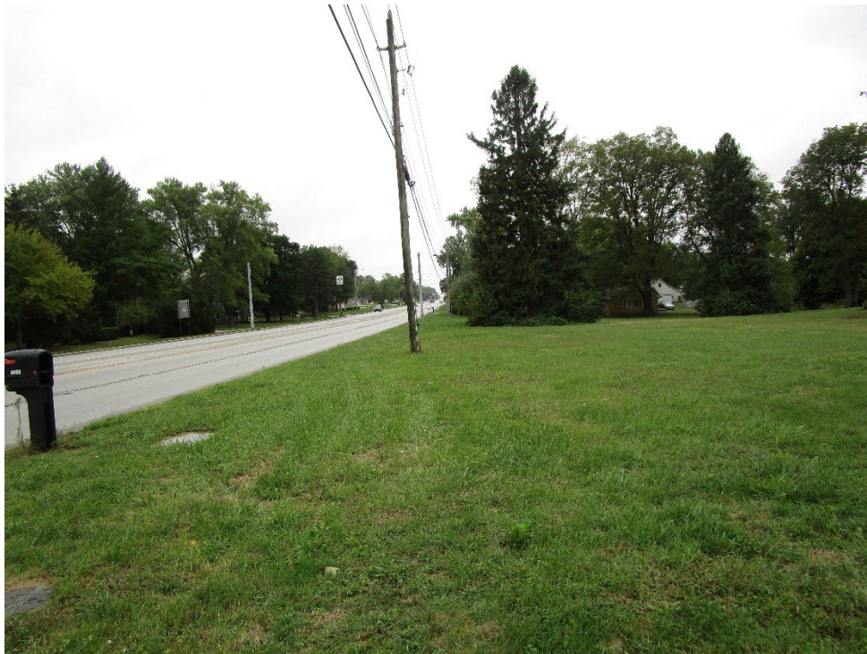
View looking south along Meridian Street
