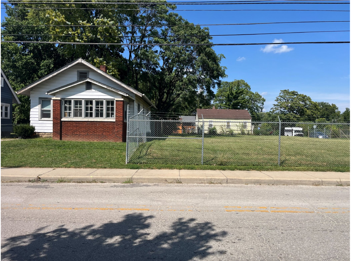
Photo 6: Looking north at subject site from 42 nd Street. Single-family homes can be seen next to the parcel and in the background.
