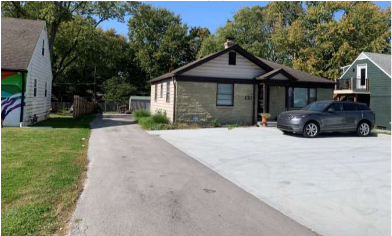
Photo of the residential property north of the site.
