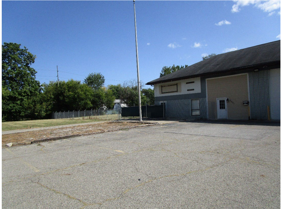
View of site looking southeast
