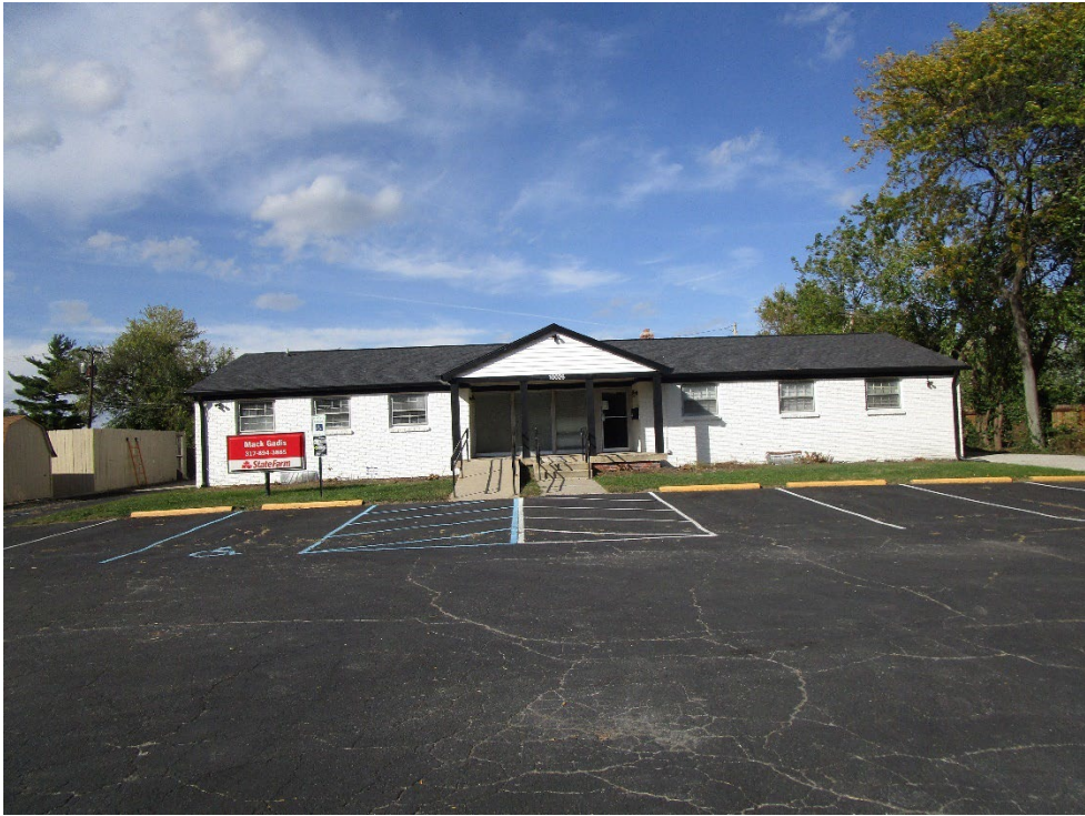
View of site looking north
