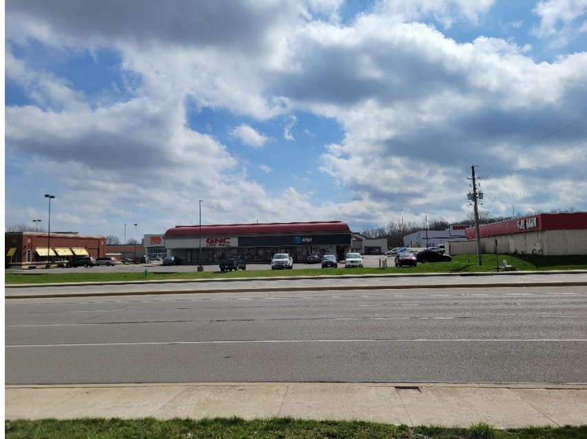
Photo 3: Adjacent Property to South
