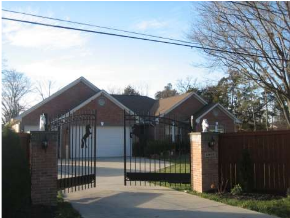
Adjacent single family dwelling to the west
