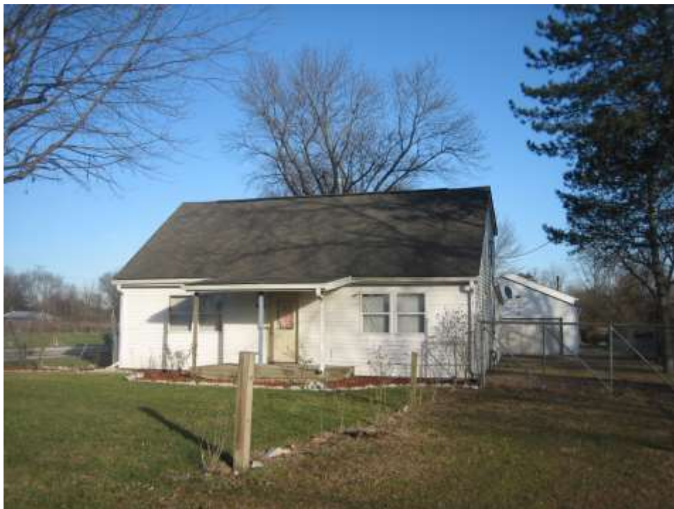
Subject site 2815 Curry Road single family dwelling, looking east
