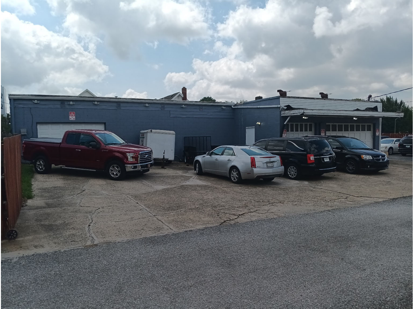
Exhibit 5: Picture of the back of Fountain Square Cremation and Funeral Services at 1420 Prospect St. The addition will be added to the left side of the building where the red truck sits to match the placement of the right side of the building.
