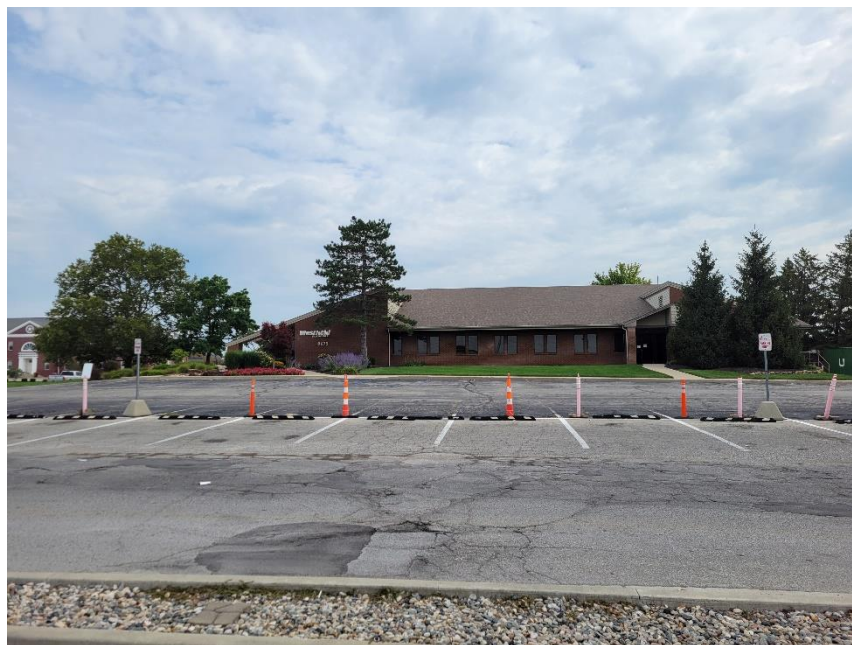
Photo 10: Adjacent Property to North
