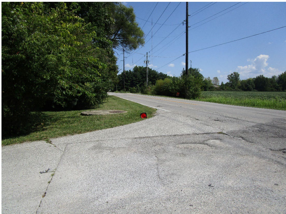
View looking east along Rawles Avenue
