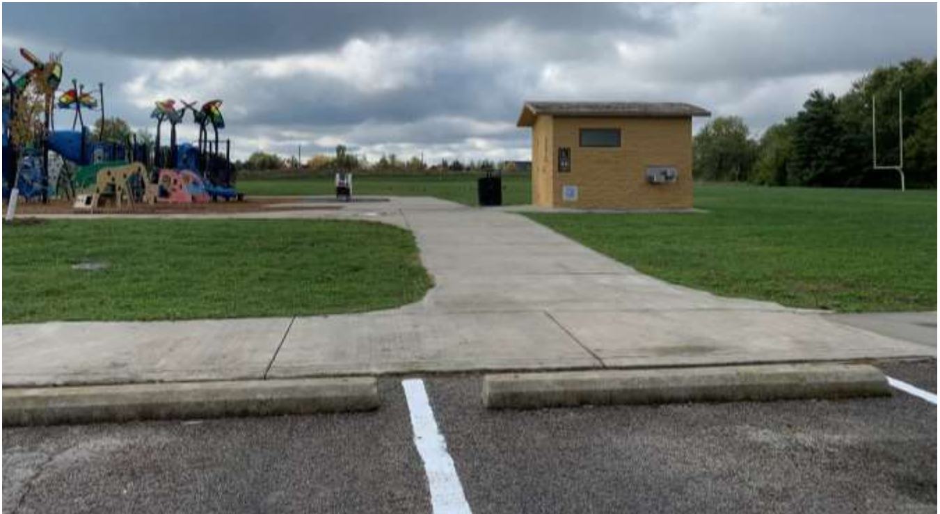
Photo of the existing playground equipment and restrooms looking south.
