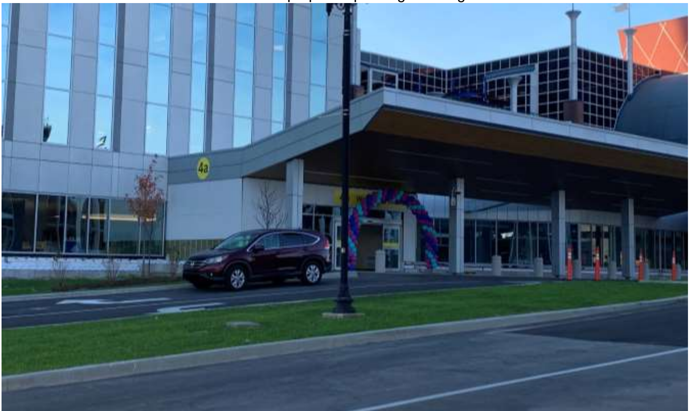
Photo of one of the wall sign locations along the southern building façade.
