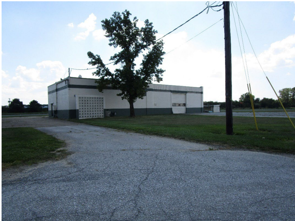
View of site looking south
