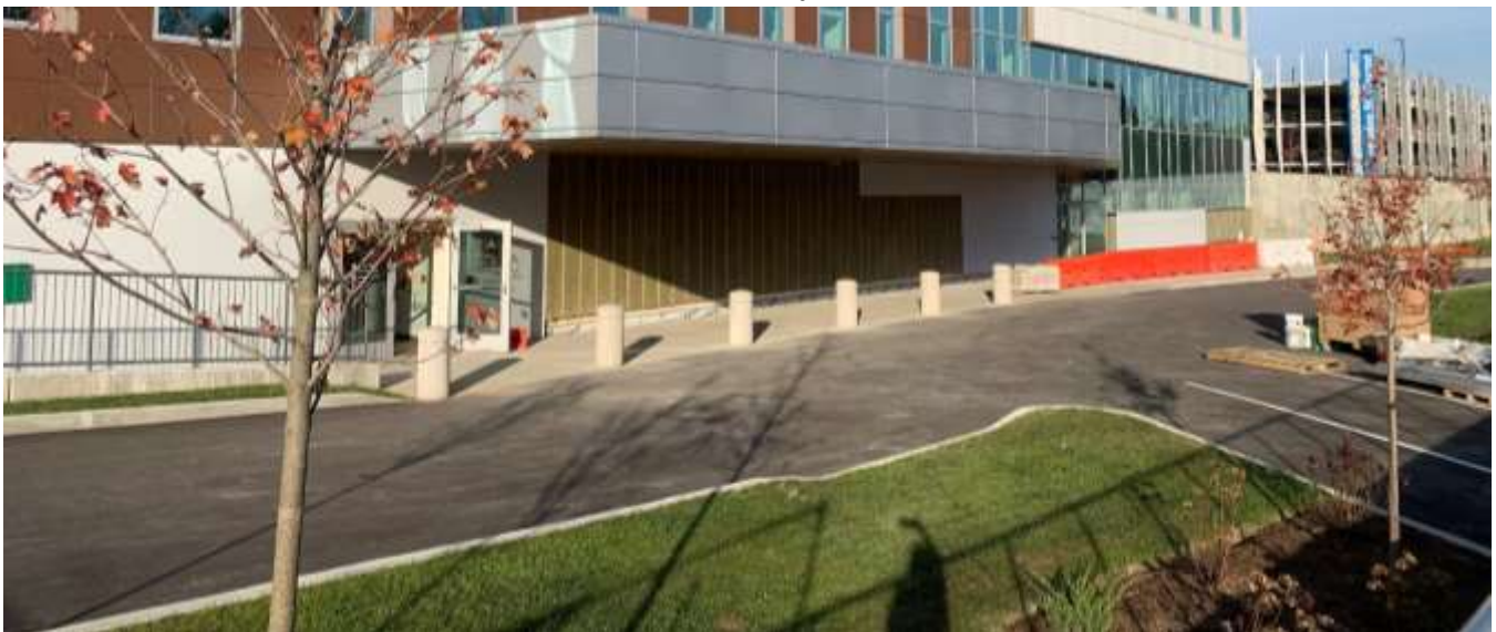
Photo of the wall sign location above the open doorway.
