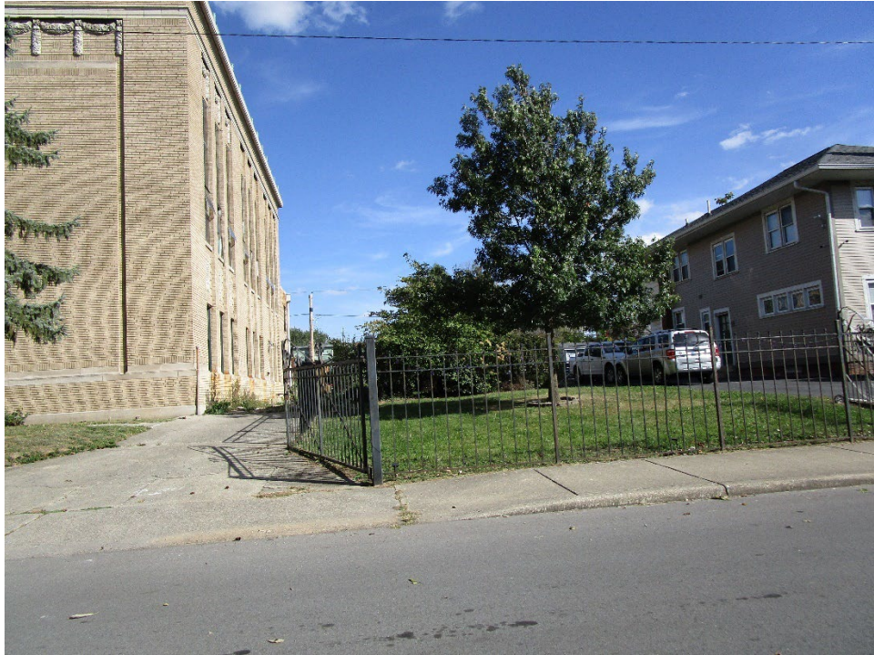
View looking east across Ruckle Street
