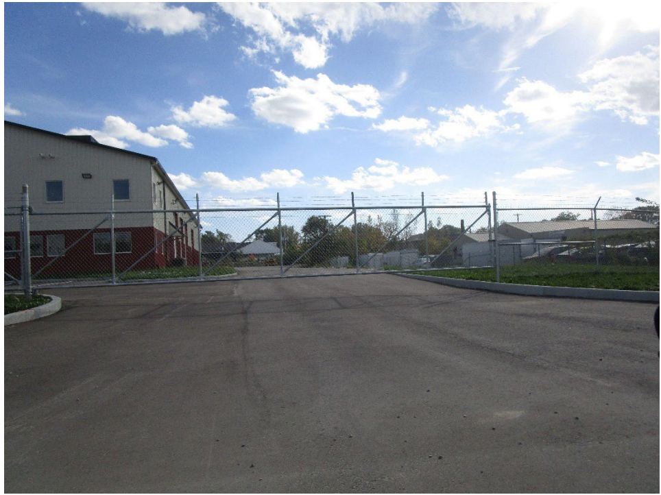
View of site looking west across Enterprise Park Place
