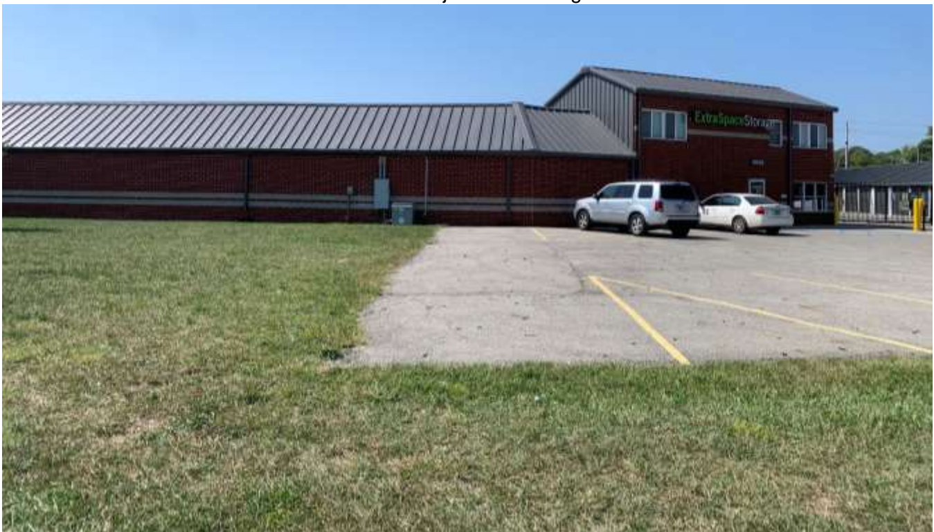
Photo of the subject site looking northwest.
