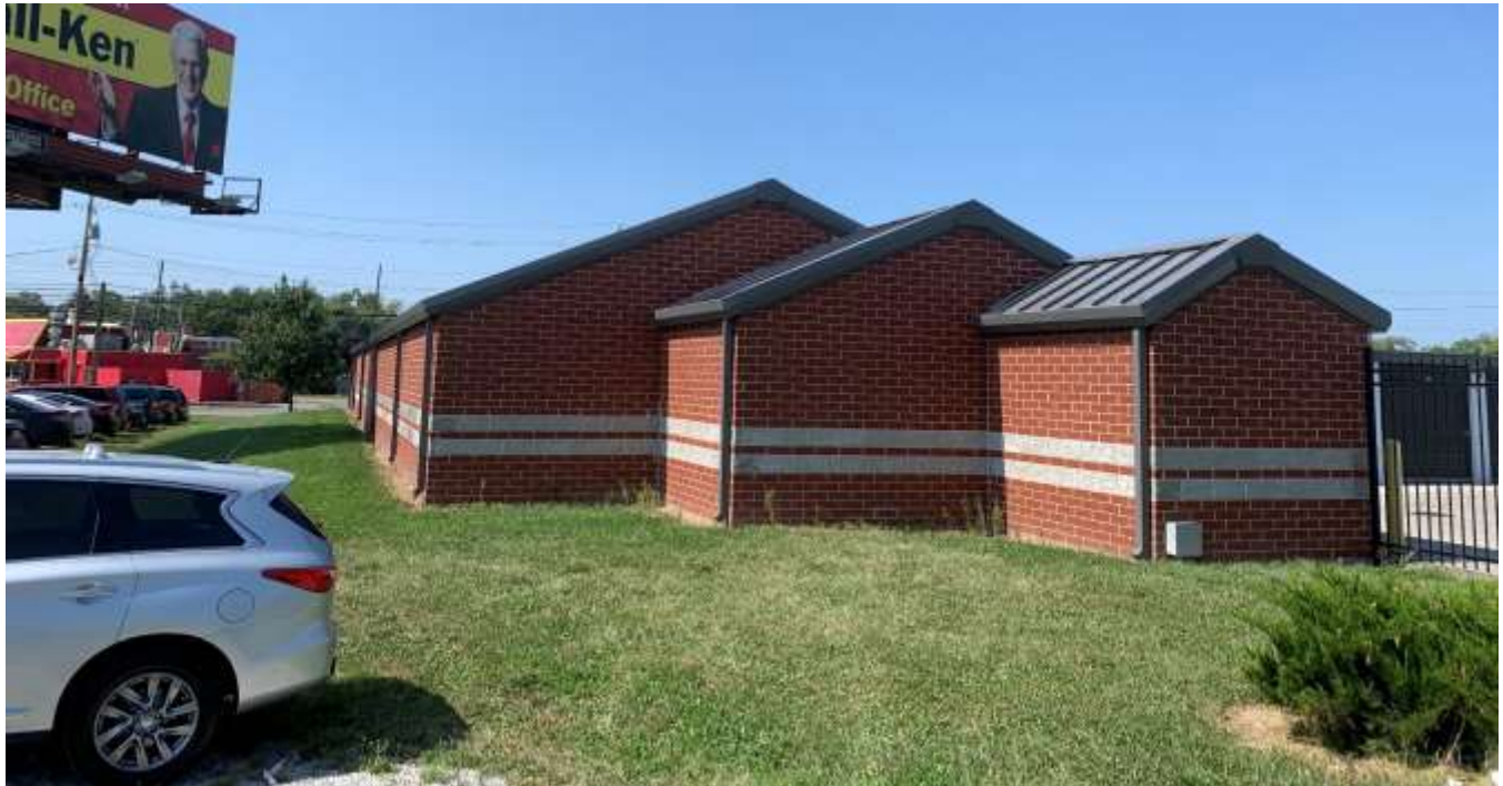
Photo of the southwestern property boundary and existing storage building.
