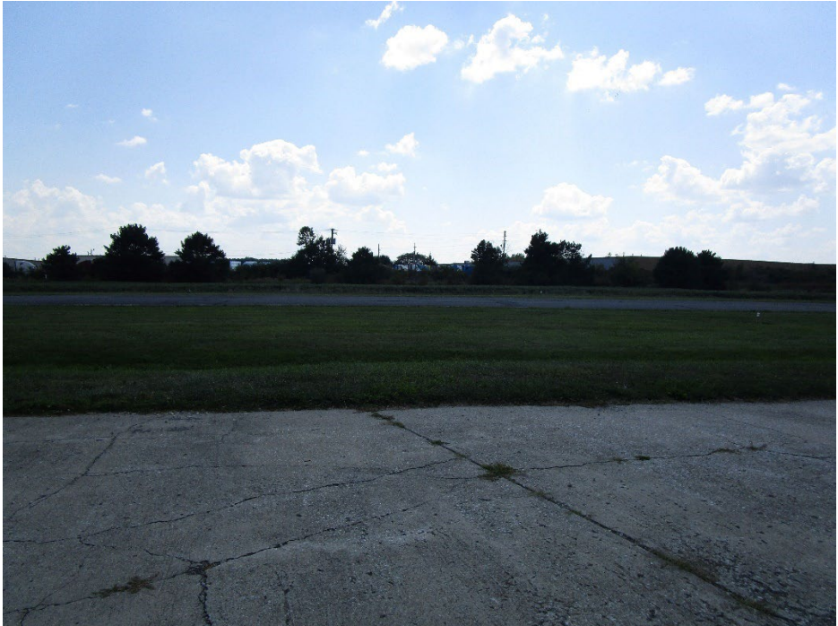
View of site looking south
