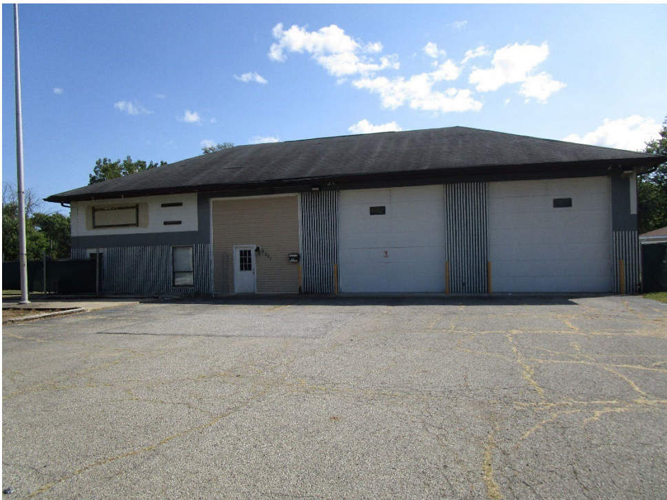
View of site looking south
