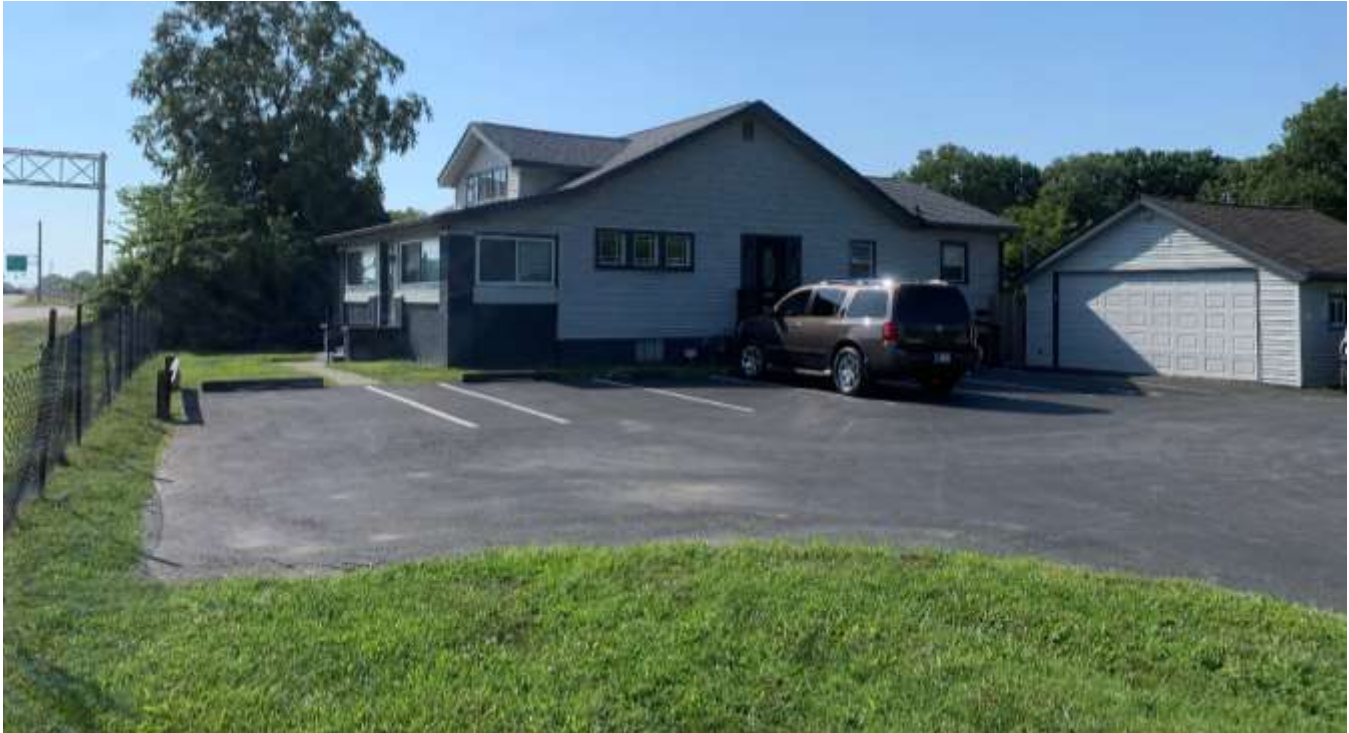
Photo of the existing residential building to be used as an office.
