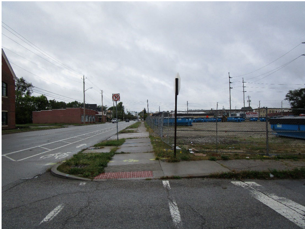
View looking north along North Illinois Street
