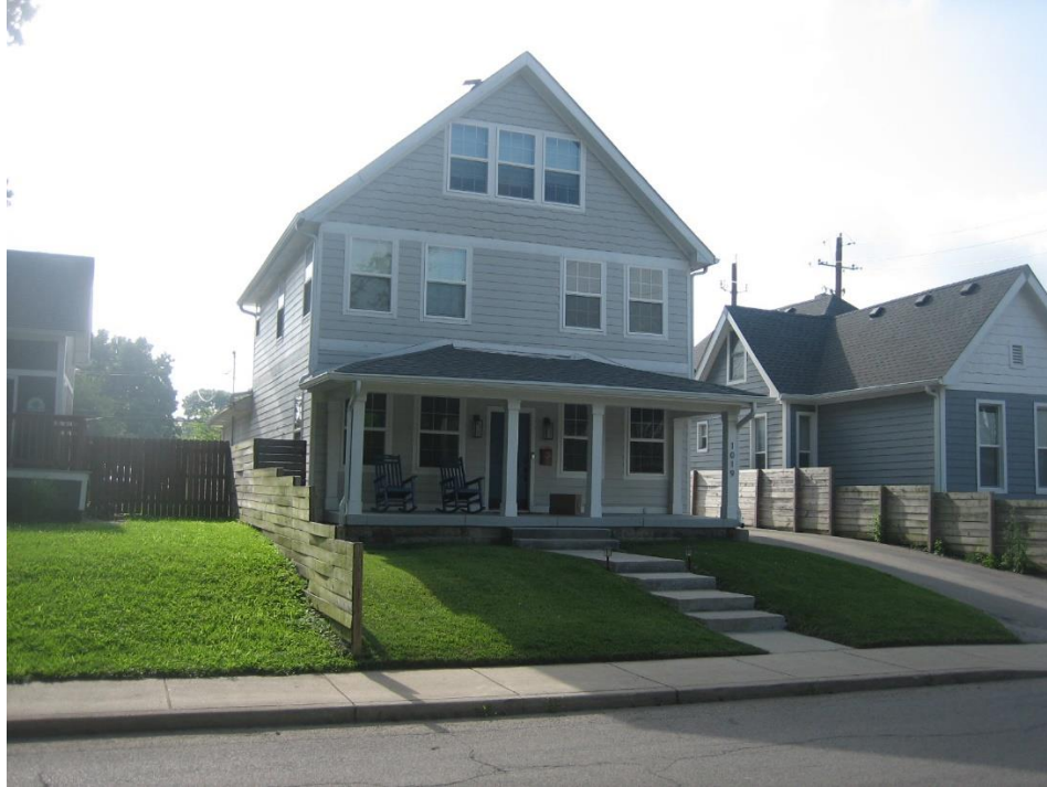
Subject site, looking east
