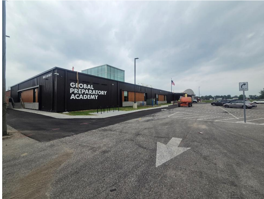
Photo 5: Building Viewed from Southeast
