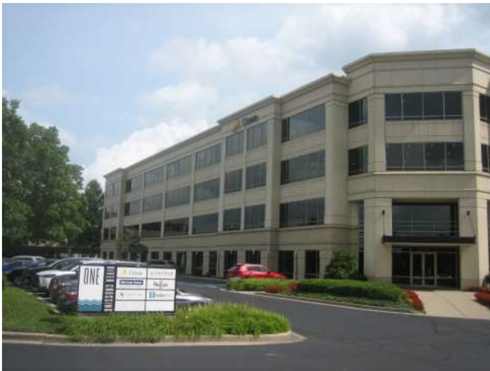
3815 River Crossing north façade, looking southeast
