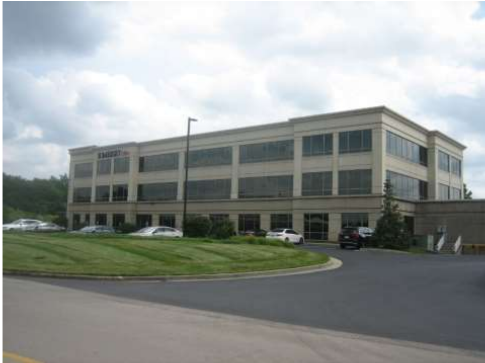
3925 River Crossing north façade, looking southeast
