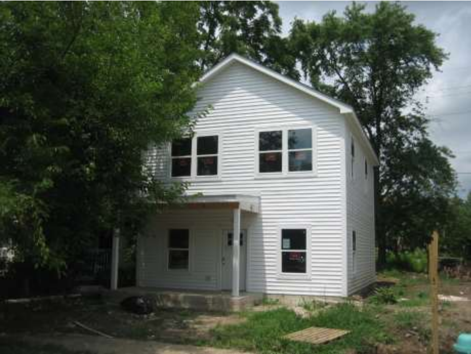
Adjacent property to the west, looking north.
