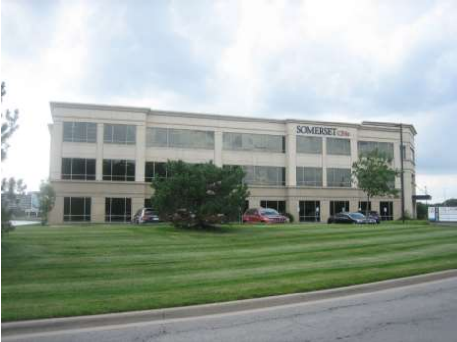
3925 River Crossing east façade, looking west
